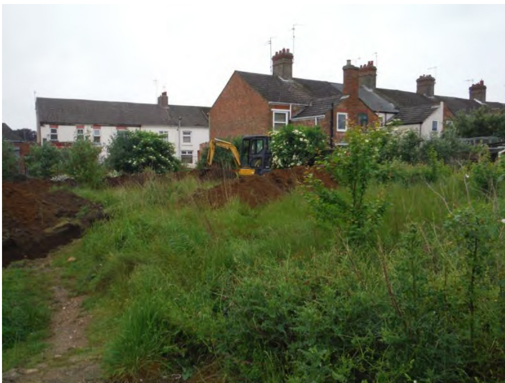
Plate 5: Site post-excavation, view southwest
