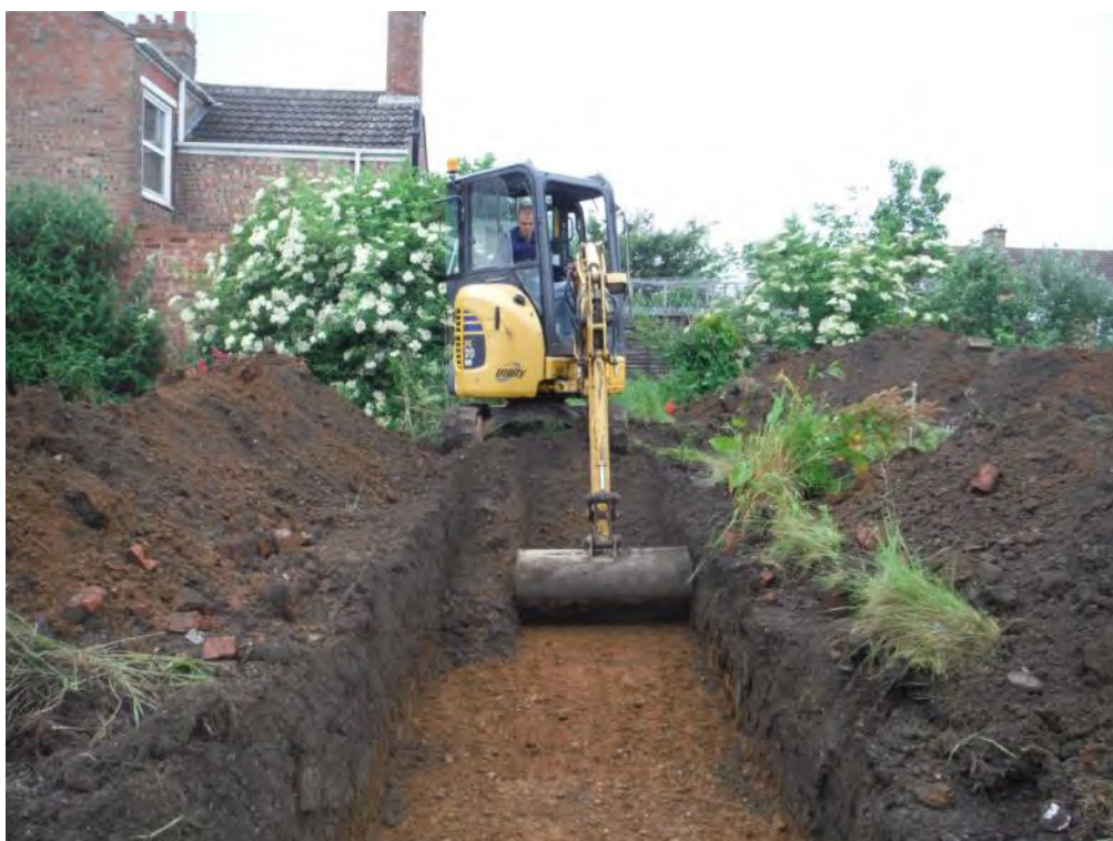
Plate 2: Machining of site, view west
