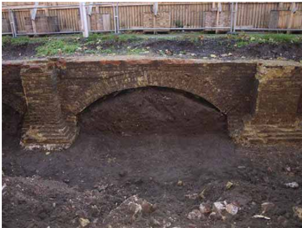
Plate 3 – The footings of St Gabriel's Church – Looking South
