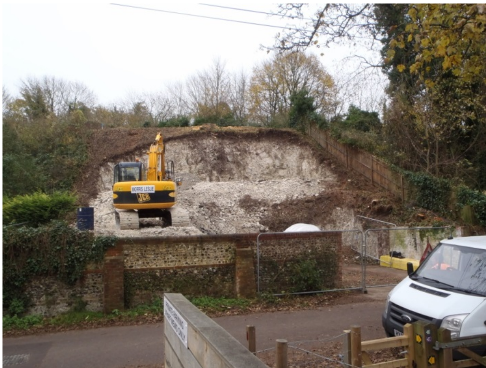
Plate 1: Mass excavation of natural chalk underway. View to east from Domum Road. Digital image D6.
