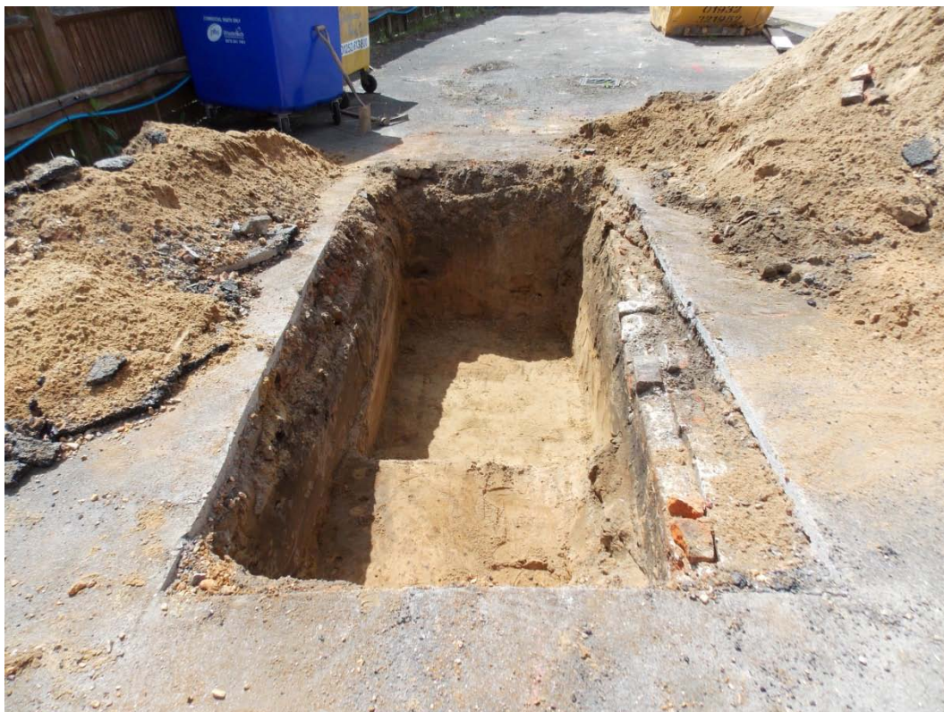
Plate 4: Overview of Trench 3, facing south.
