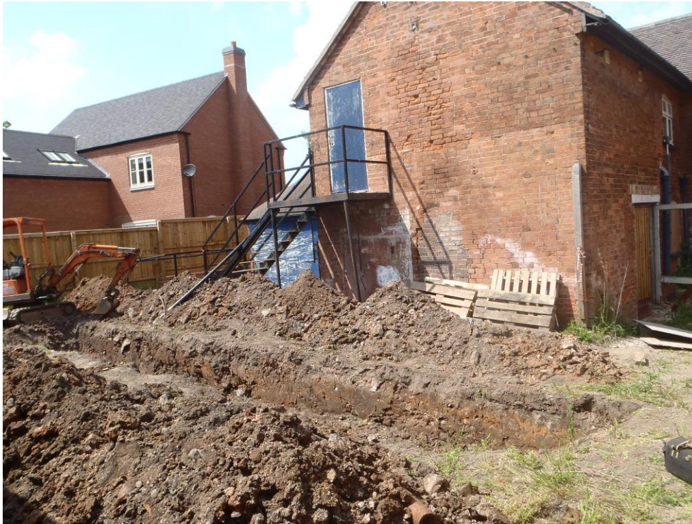
Plate 1: General View of Trench (looking North West)
