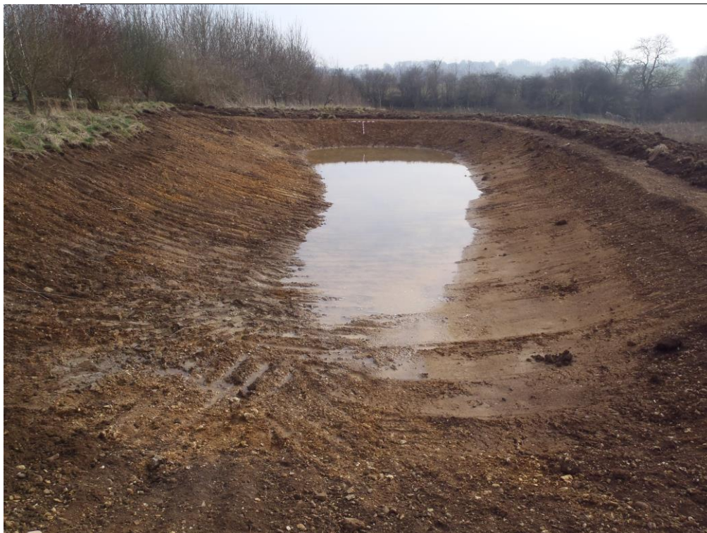
Plate 5: General View of Pond 2H (looking South, Scales 1x1m)
