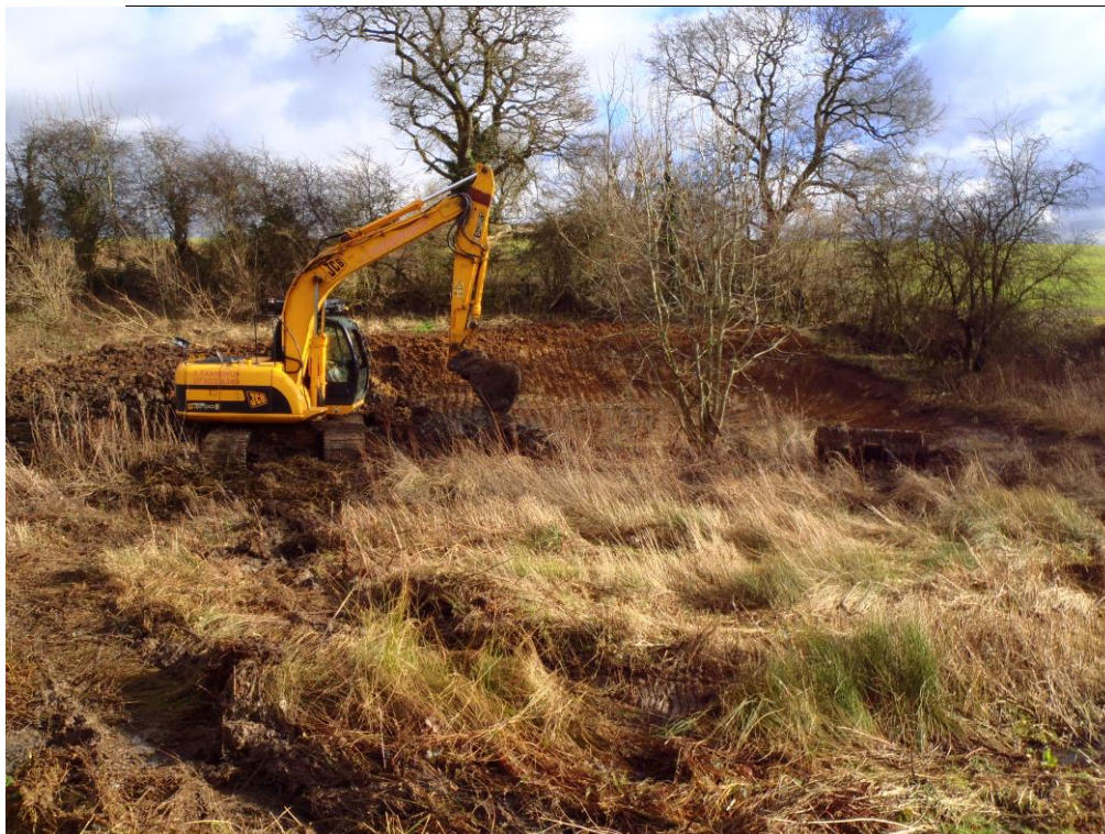
Plate 9: General working view of Pond 8A (looking South-East)
