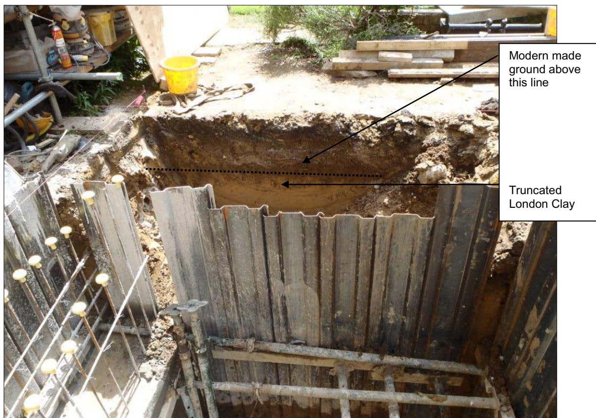
Plate 2: Excavation at South of Site, Looking South
