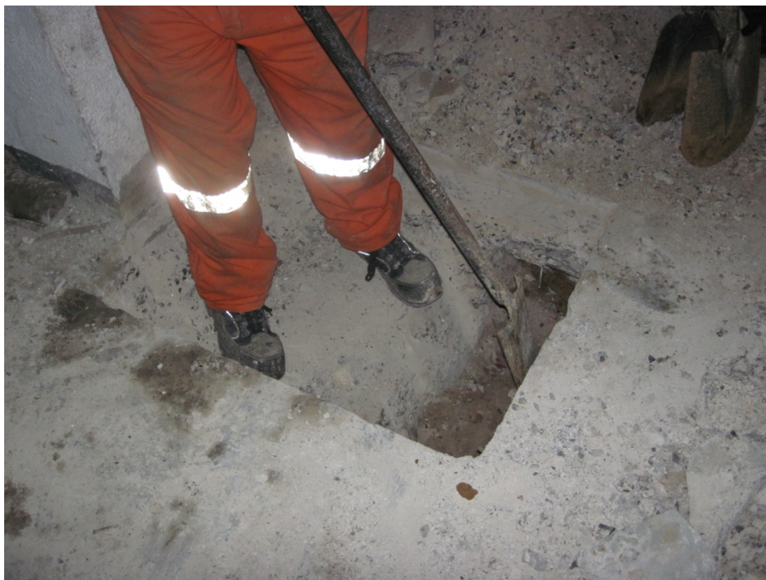
Plate 3 South facing view of Test Pit 3; only (+) (concrete and hardcore) was encountered
