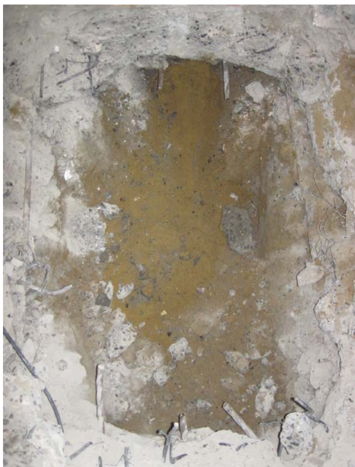
Plate 7 East facing view of Test Pit 8; natural deposits immediately below concrete
