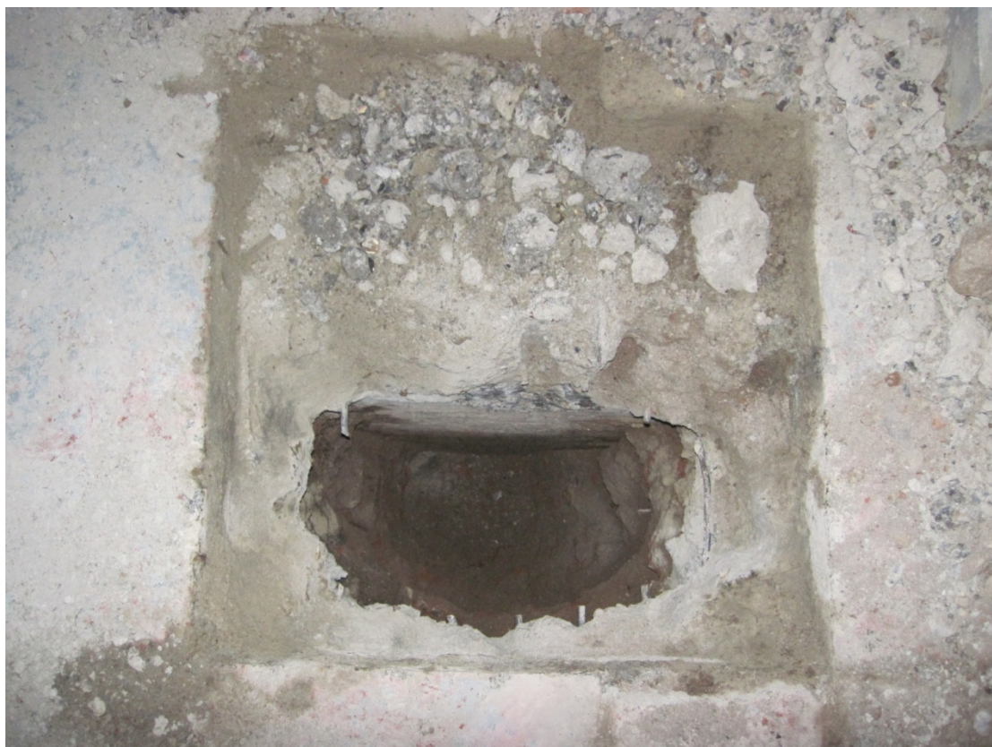
Plate 3 South facing view of Test Pit 3; only (+) (concrete and hardcore) was encountered
