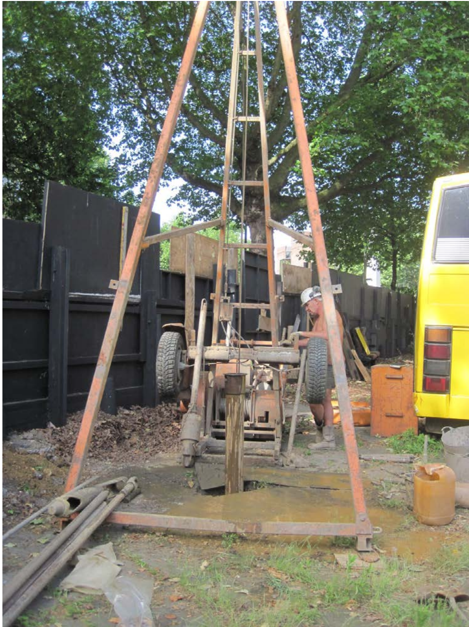
Plate 8 West facing view of Borehole 6 being excavated
