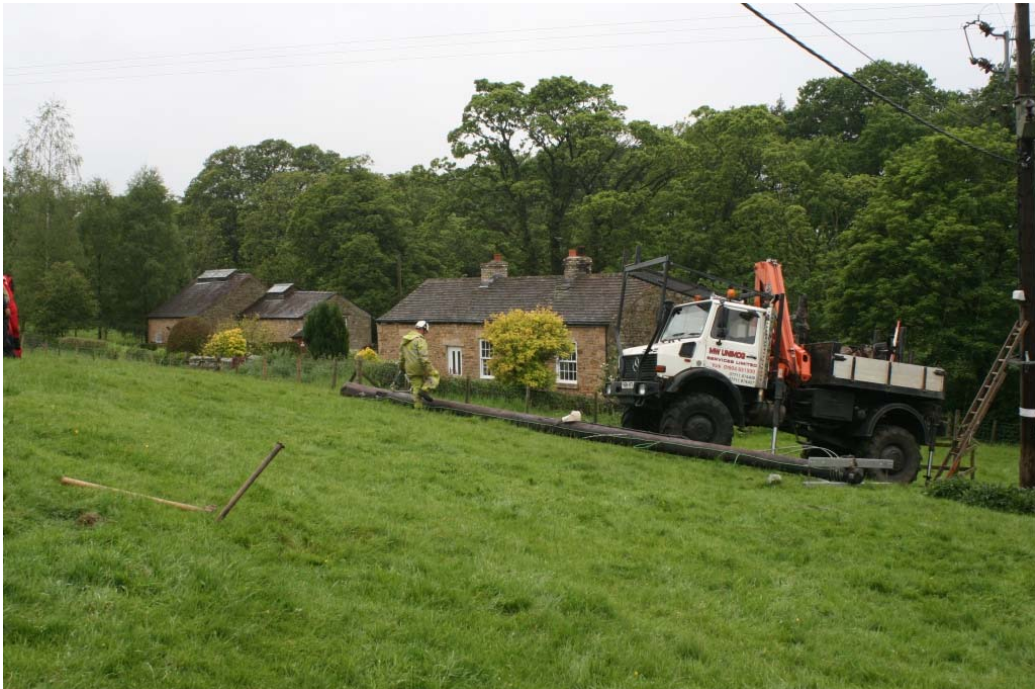
Plate 4. Installation of OHL H-pole with Teesview Cottage in the background
