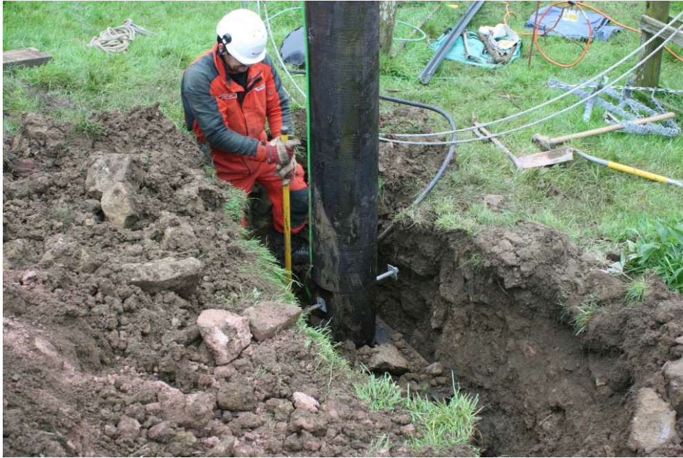
Plate 3. Installation of OHL H-pole in trench
