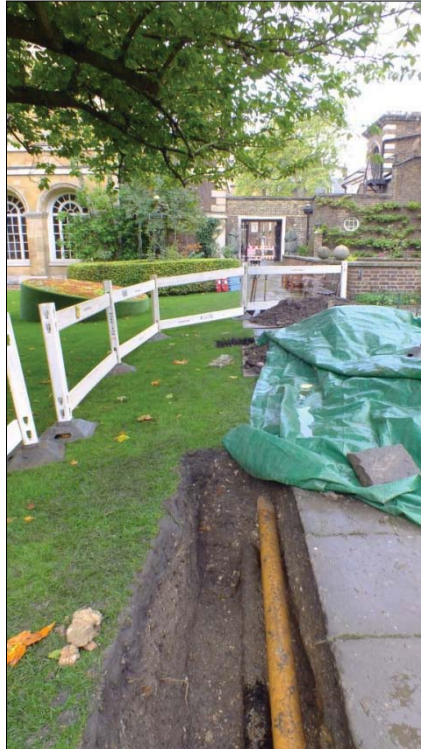
Plate 3: Trench 100 (foreground) and Trench 101 (middle distance), Looking West
