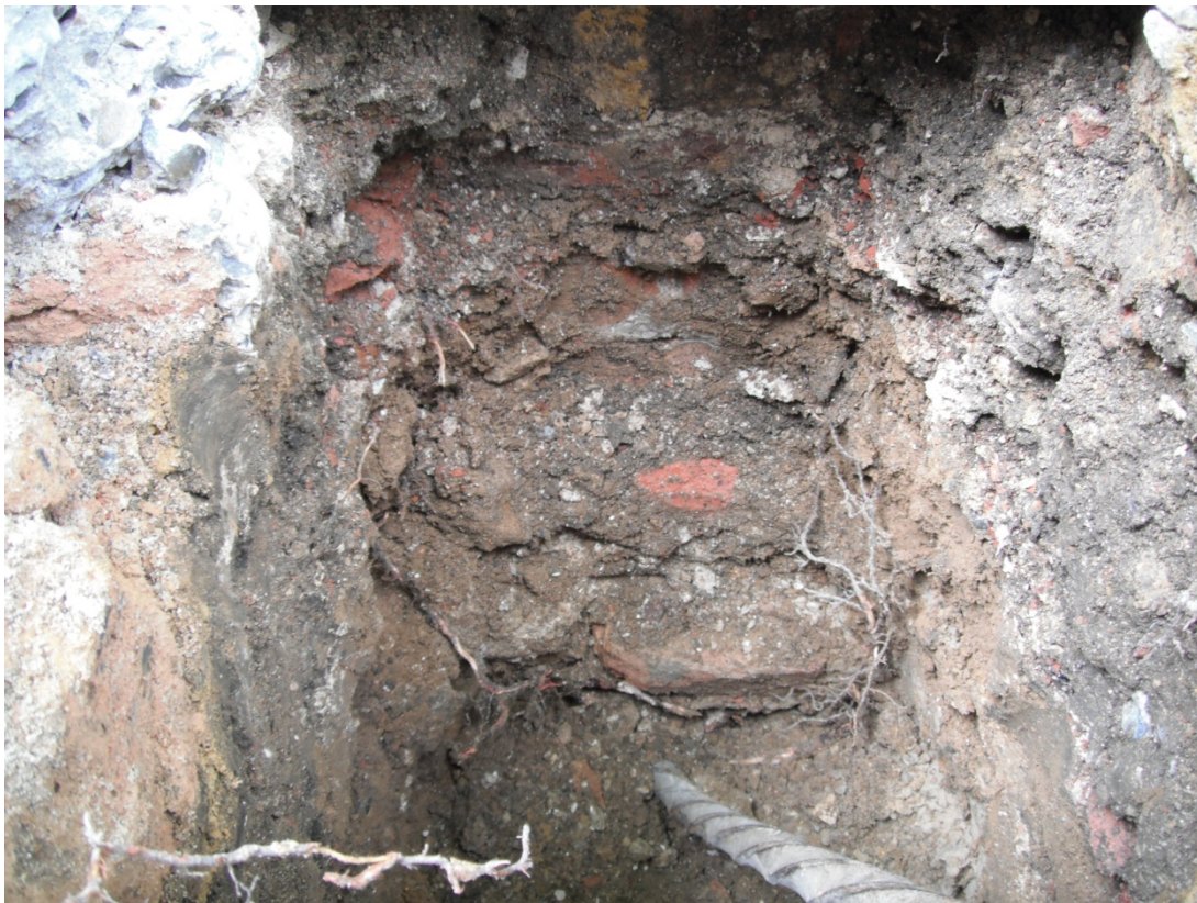
Test Pit 2 showing earlier stepped brick footing
