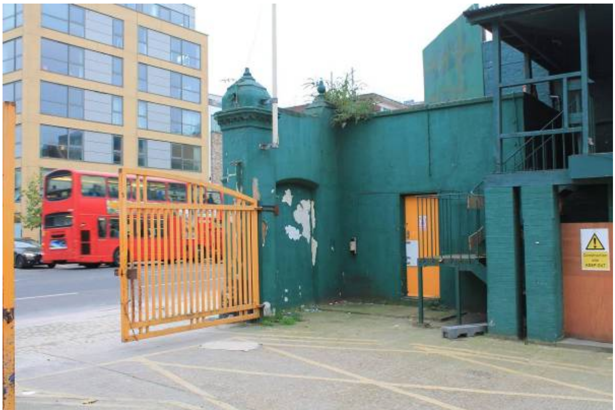
Plate 14 View to southern gate pier and blocked pedestrian entrance, looking south-east
