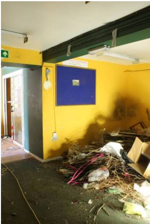
Plate 20 Area CG5 looking south-east
