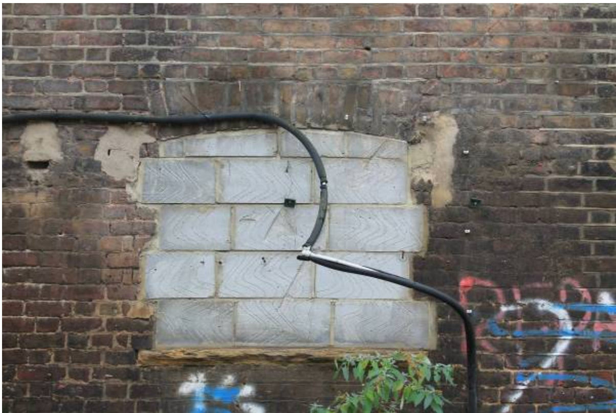
Plate 10 Detail of blocked ground floor window in building (C), looking south
