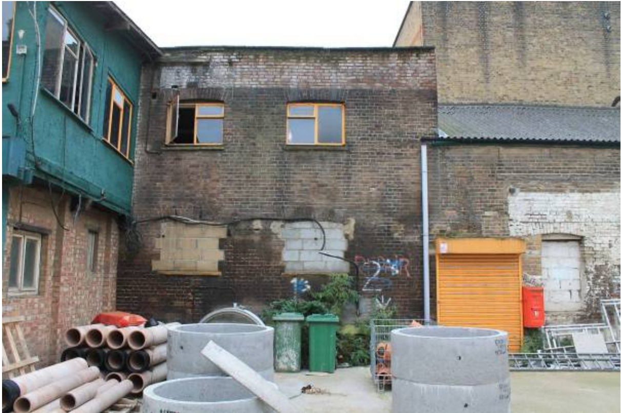
Plate 9 Western part of building (C) looking south
