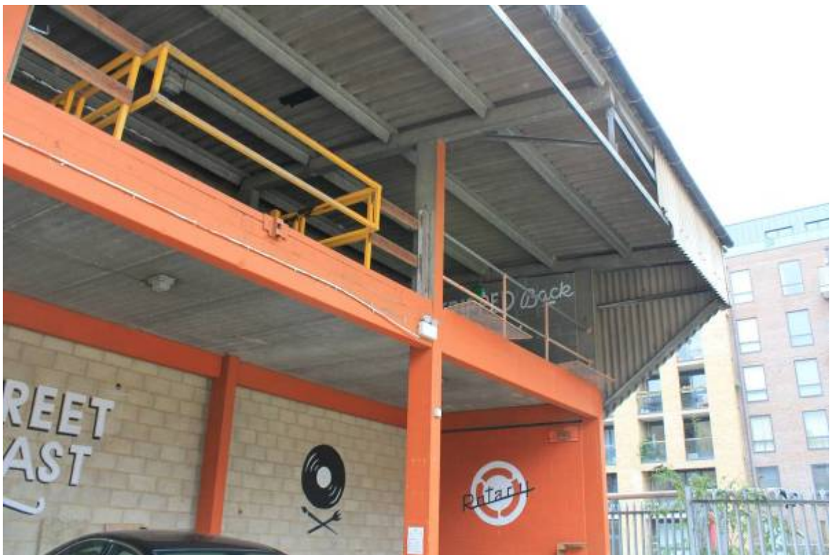
Plate 6 Structural detail of shelter (A), looking west
