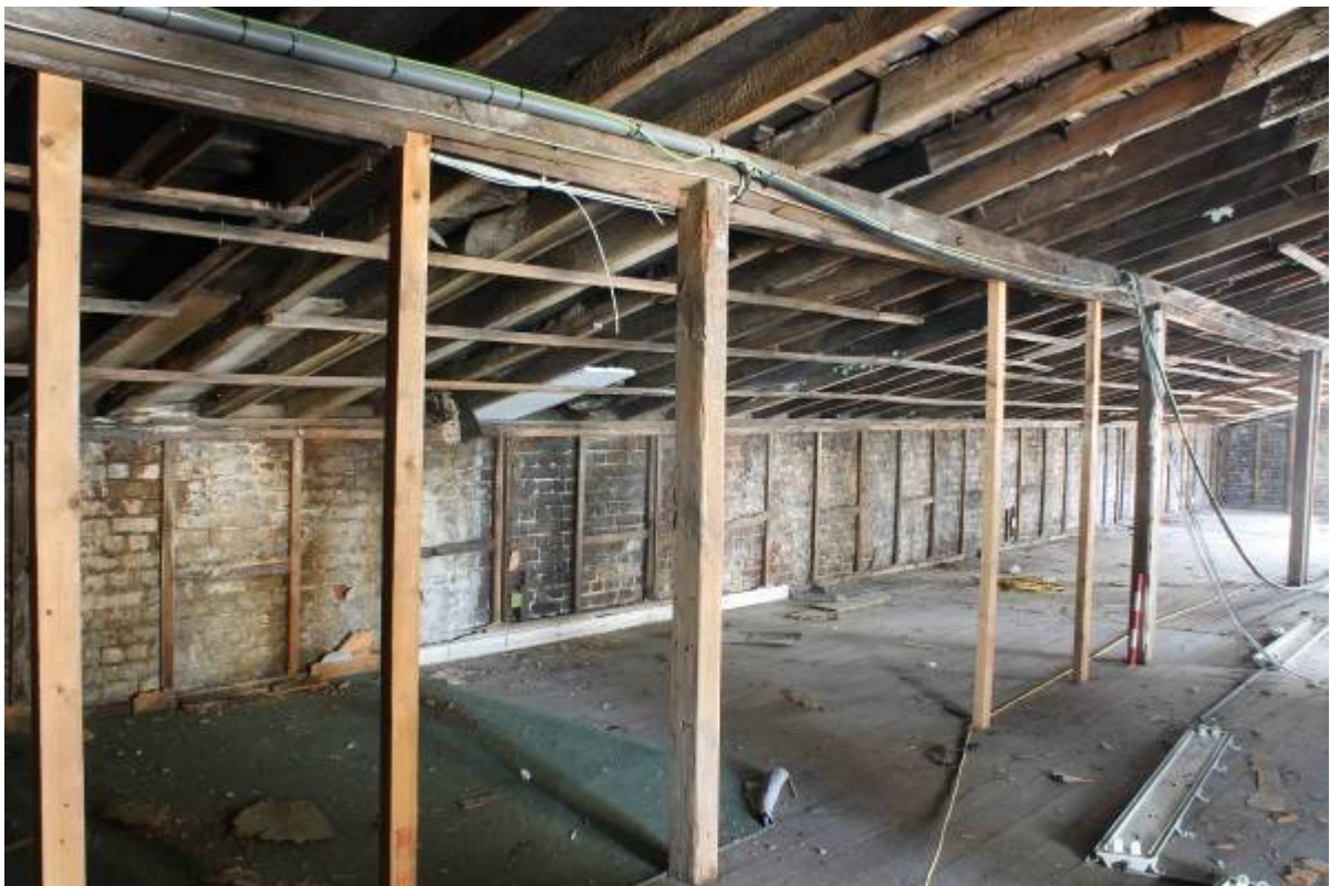
Plate 32 Area CF2, showing lean-to roof, looking south-west
