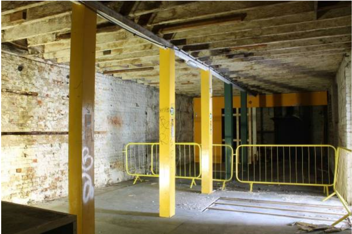
Plate 23 Area CG7 (Stable C) showing posts (to former stalls), looking west
