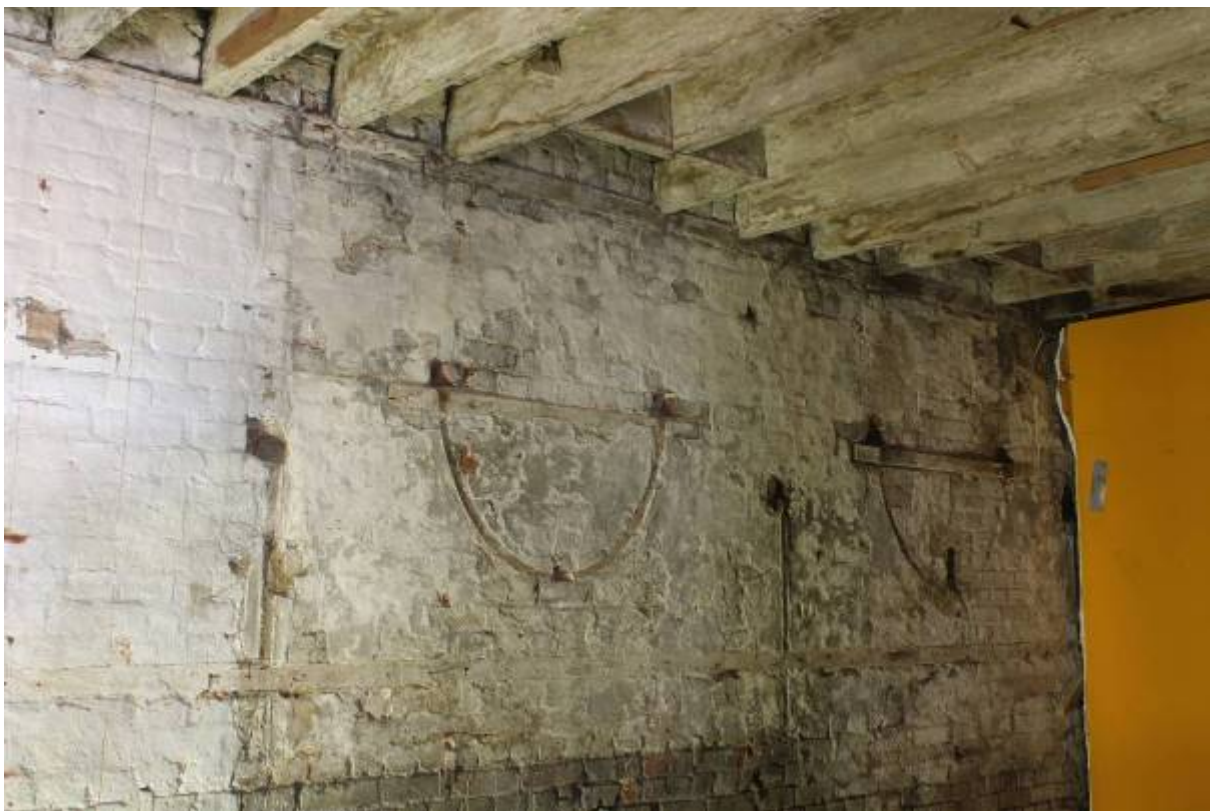
Plate 26 Scars of hay baskets seen directly below hatches, looking south-west
