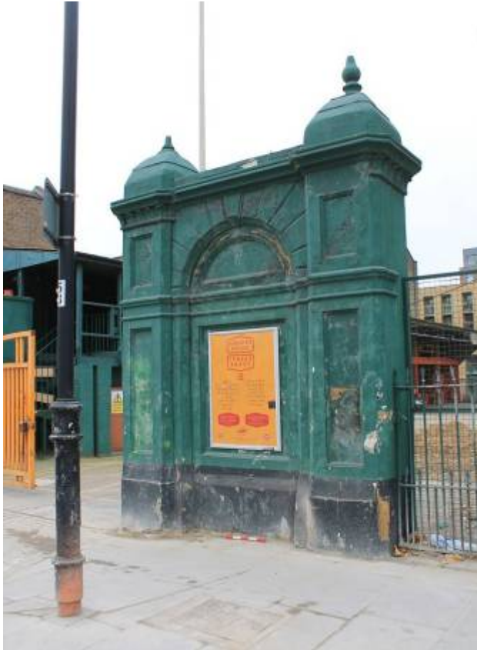
Plate 17 Northern gate pier from Kingsland Road, looking west
