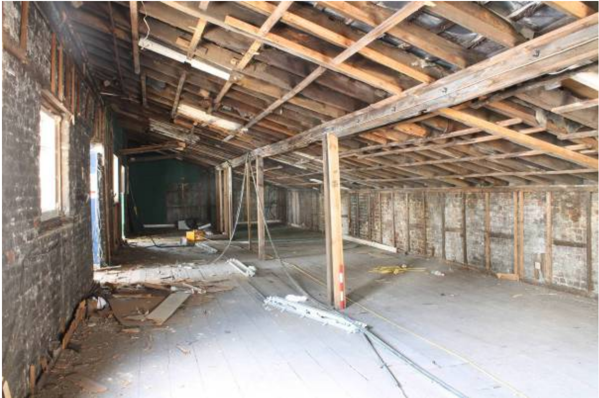
Plate 33 Area CF2 looking east showing lean-to roof and purlin
