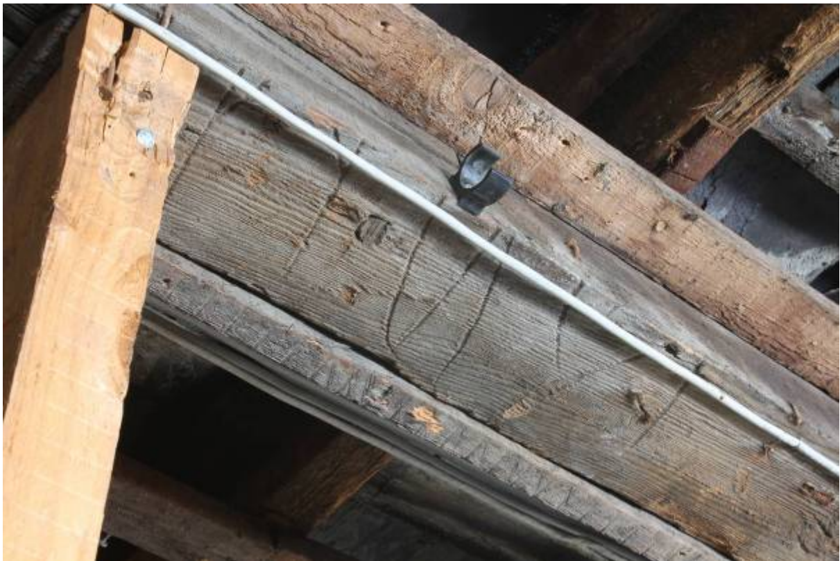
Plate 34 Baltic marks on purlin, looking south-west
