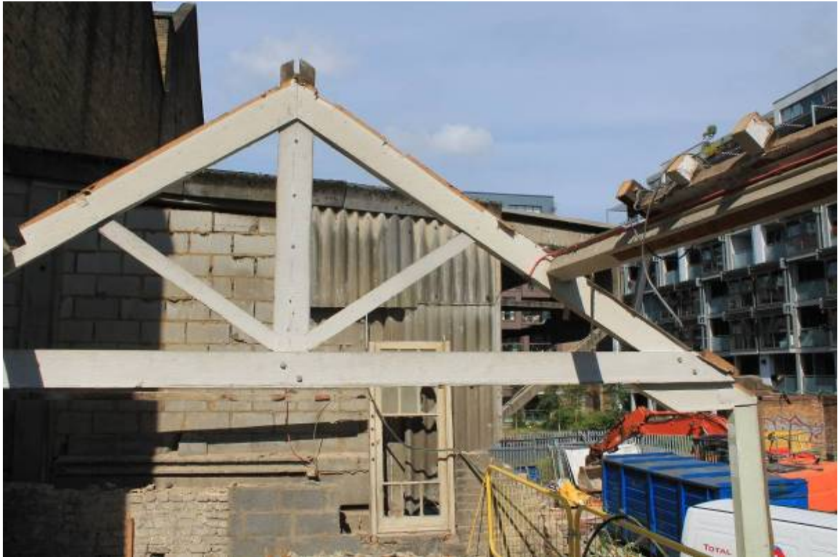
Plate 31 Area BF1 during demolition, showing kingpost truss, looking west
