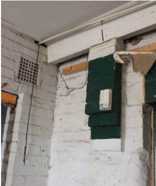
Plate 21 Brick corbel and bull-nosed jamb with stop in area DG9, looking south-east
