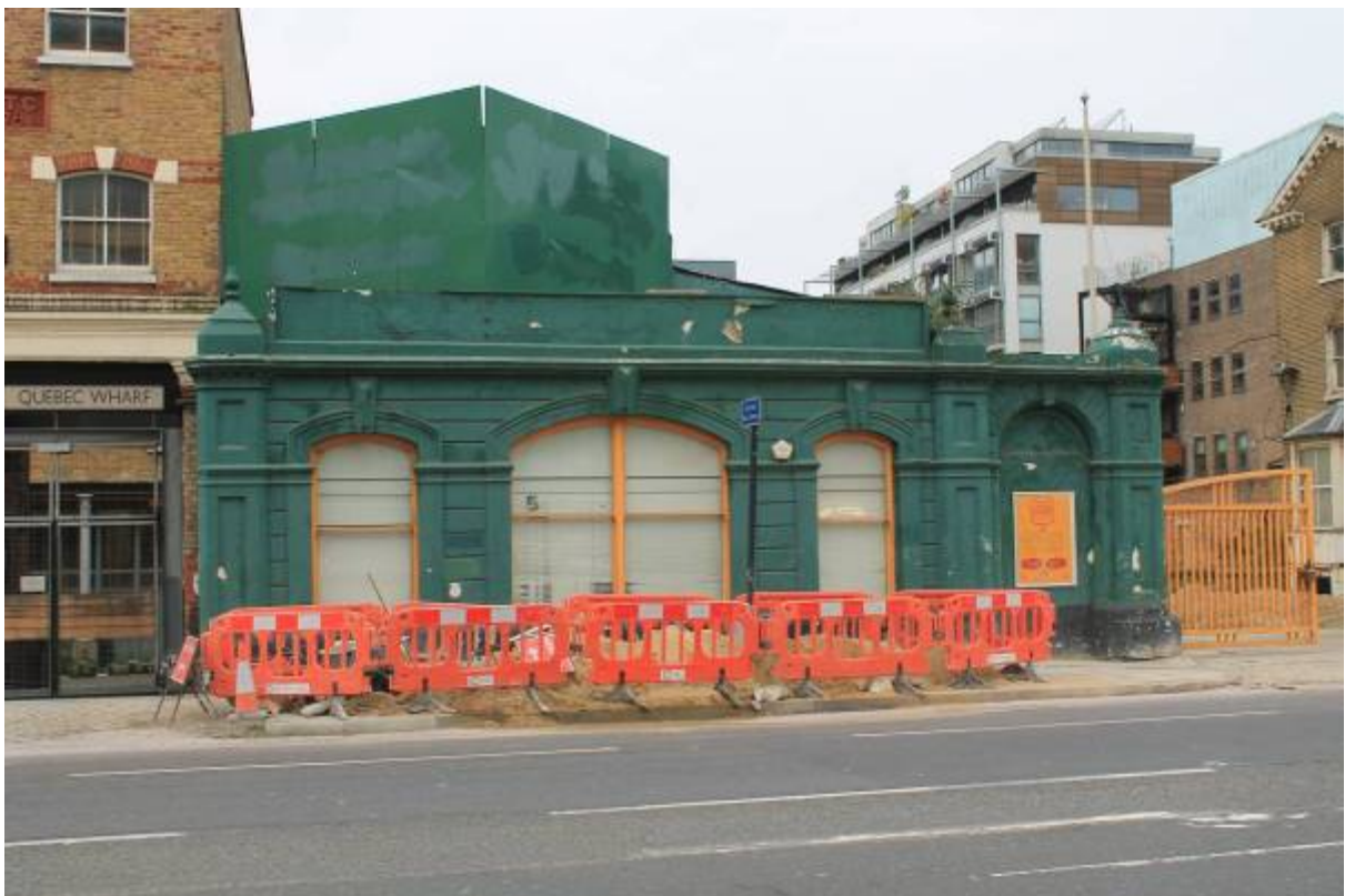
Plate 18 Office range (E) looking west from Kingsland Road
