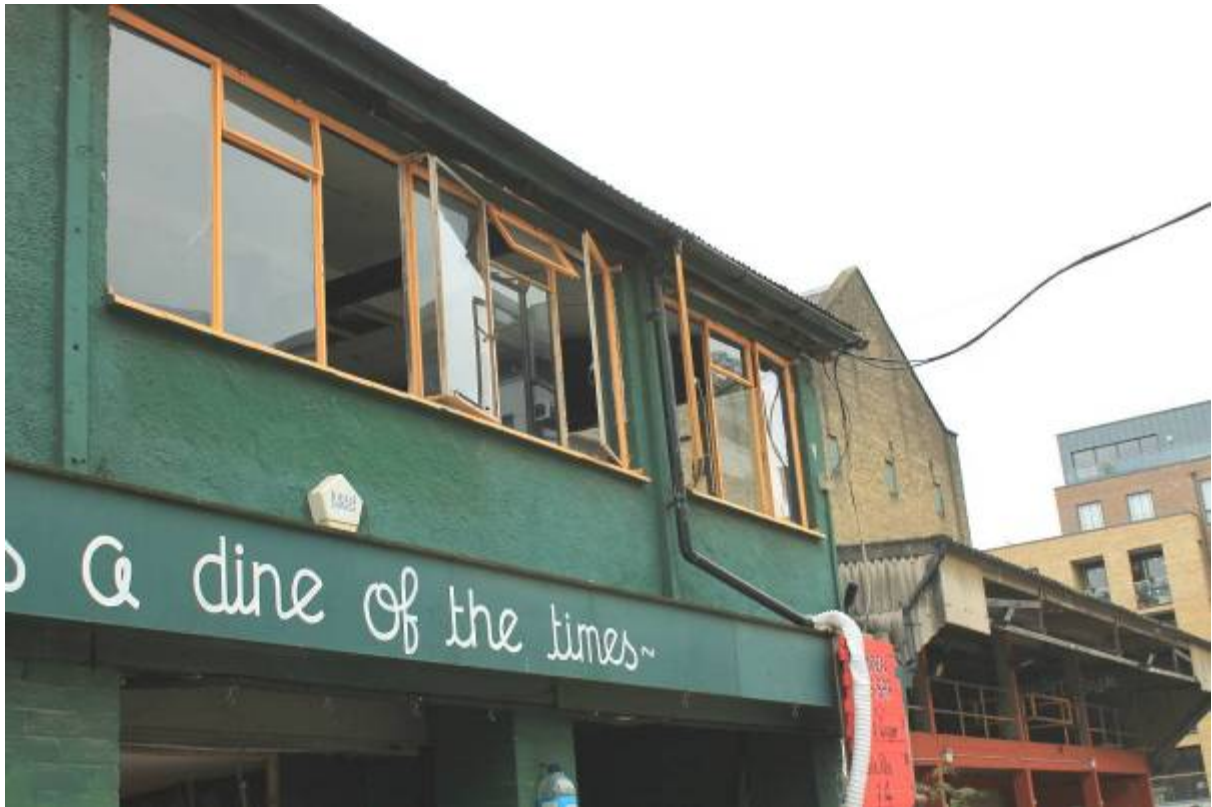
Plate 13 First floor windows in building (D), looking south-west
