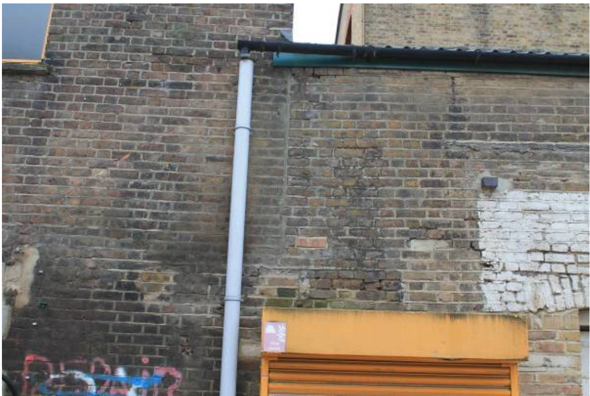
Plate 8 Straight joint between (B) and (C), looking south
