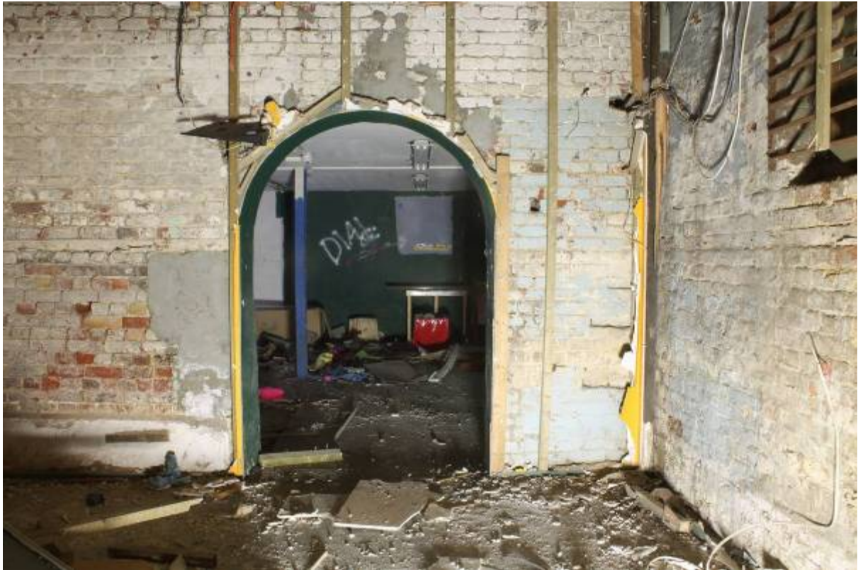
Plate 29 View towards BG13 from CG7, through inserted arch, looking west
