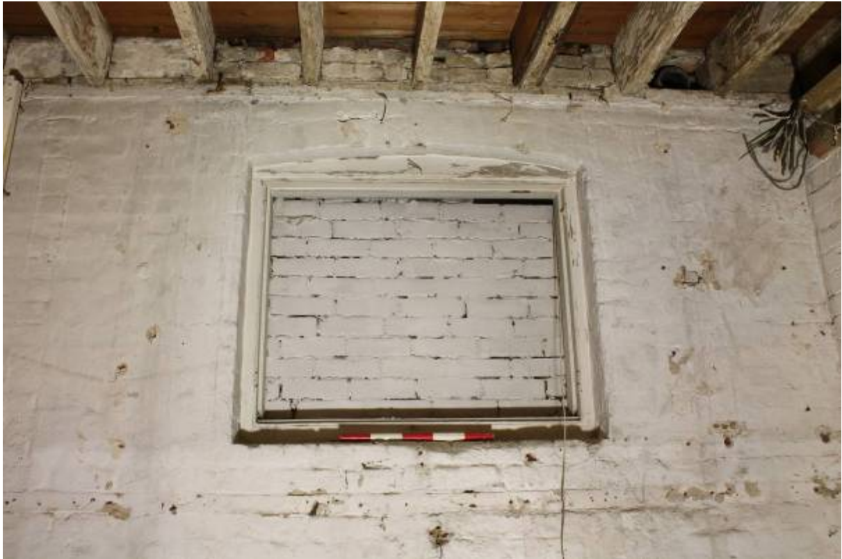
Plate 27 Blocked window in CG7 north wall, looking north
