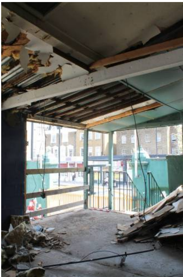
Plate 36 DF3 looking north-east
