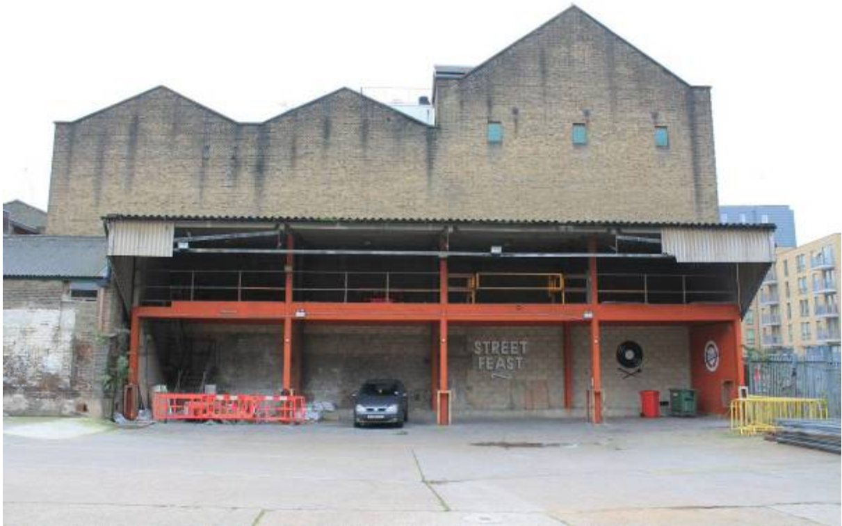
Plate 5 Open-fronted shelter range (A) looking south toward Quebec Wharf
