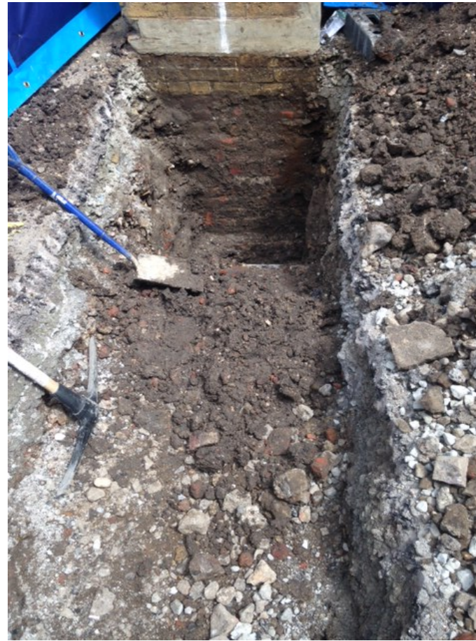
Plate 2: North facing shot of trial pit 1 illustrating made ground [2] in foreground
