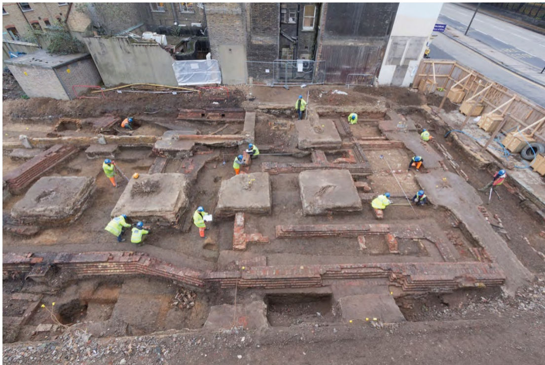
Plate 6 View of Phase 5 masonry (also shows in situ Phase 4c, Phase 4b and Phase 4a masonry; looking south-west)
