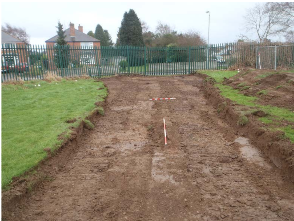
Plate 1: Site contractors service road. Facing South East
