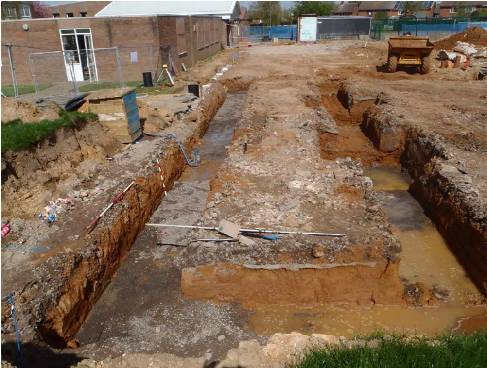
Plate 5: Footprint of Sports Hall: general location shot. Facing North
