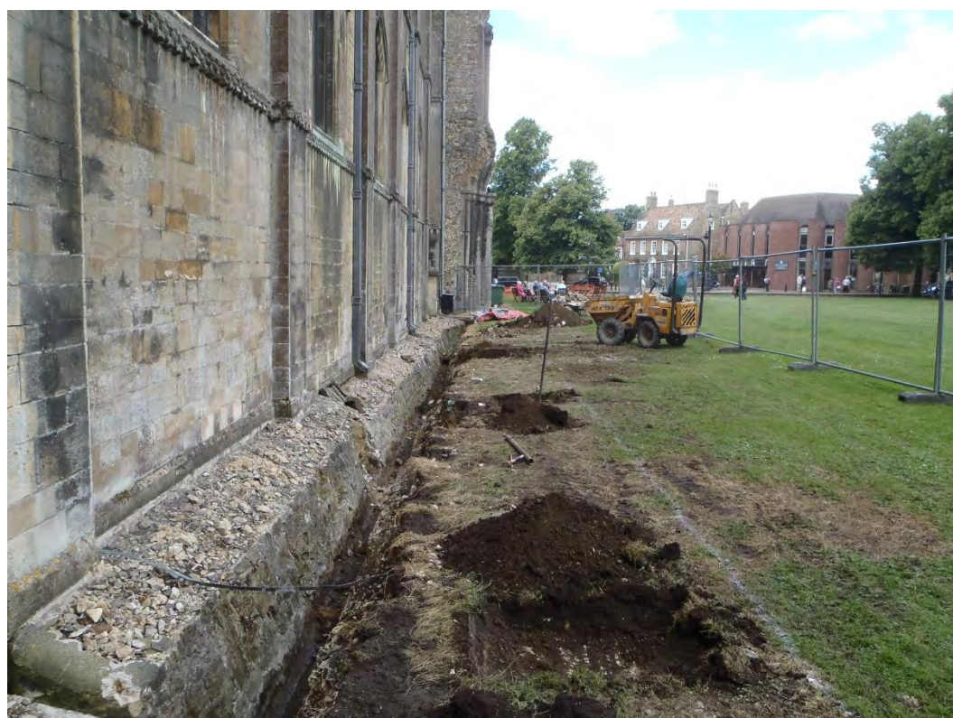
Plate 2: The site, view west
