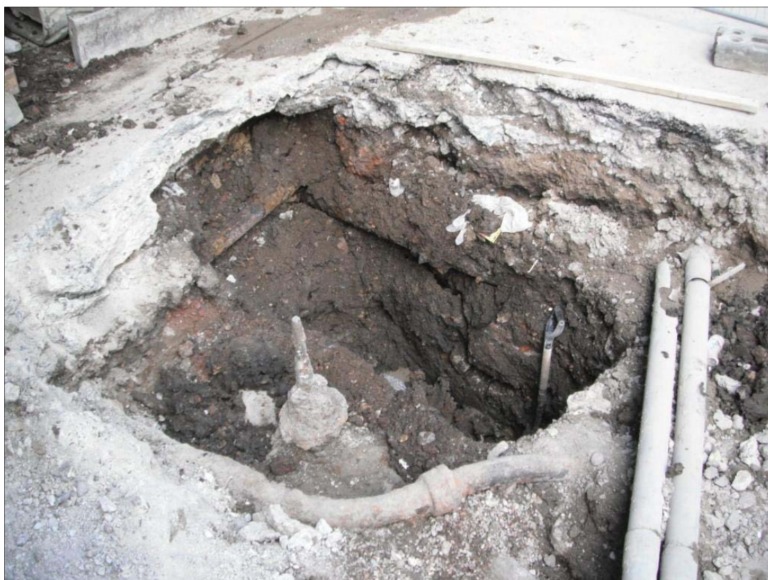
Plate 2: Inspection Pit 1, Looking South-East
