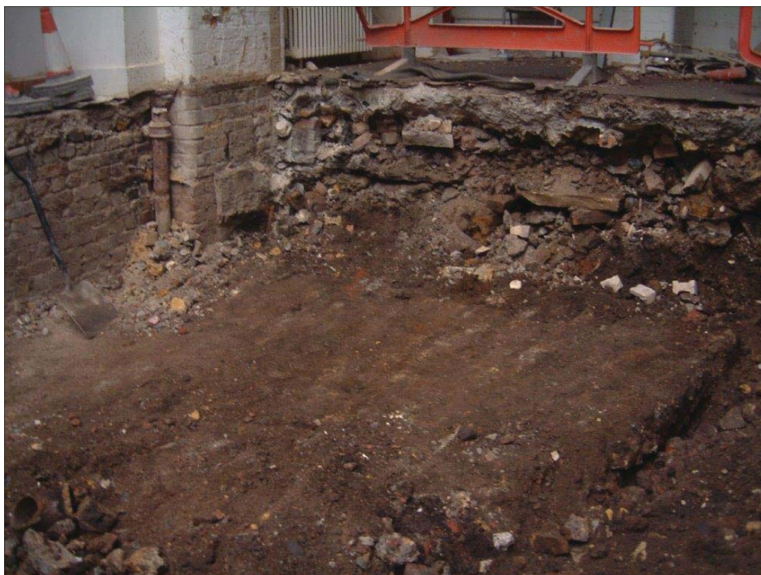
Plate 1: Crane Base Excavation Area, Looking North-West
