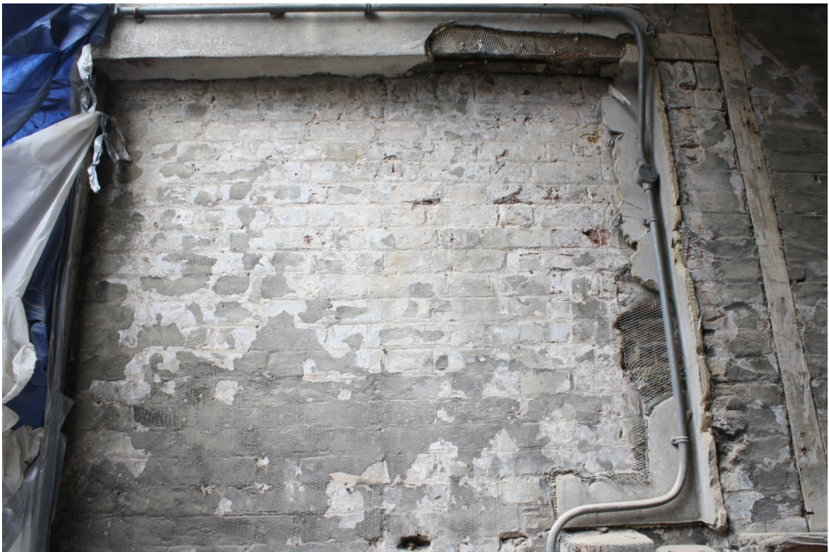
Plate 4: Upper part of the west end of the south elevation of no. 127 Borough High Street following the removal of the cement render, looking north
