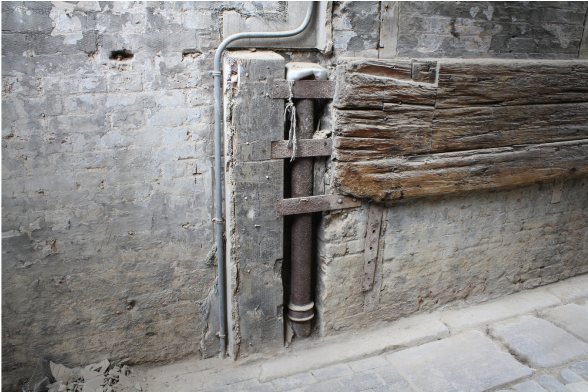
Plate 6: Vertical timber and drain pipe at the east end of the recess in the south elevation of no. 127 Borough High Street, looking north
