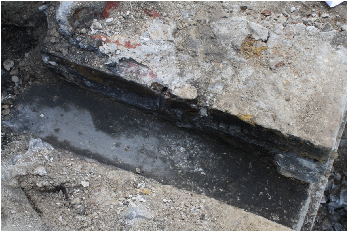
Plate 25: Plan view of Flue 1 during dismantling, looking down and south
