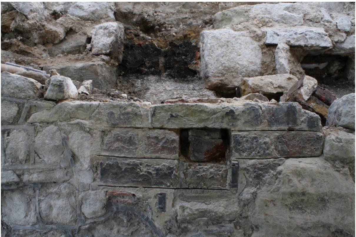
Plate 22: North elevation of Flue 1 during dismantling, looking south
