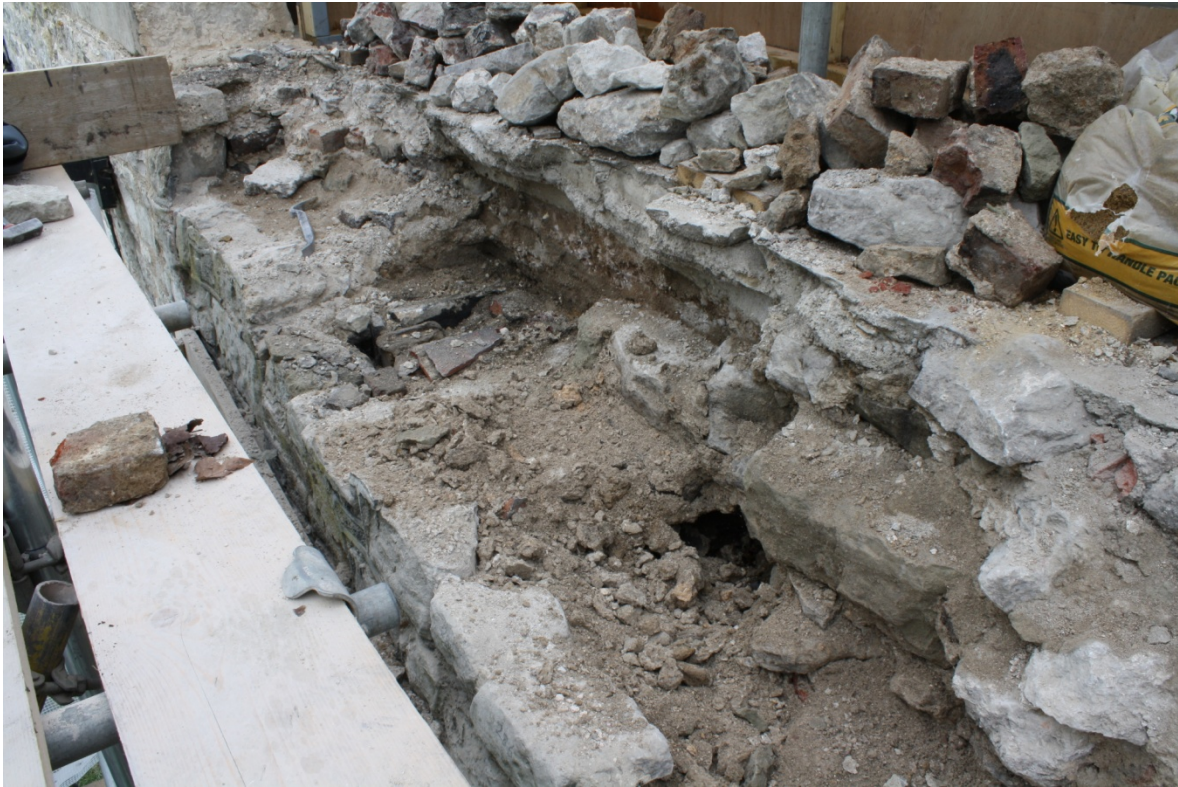
Plate 17: Plan view along the top of the wall during dismantling showing rubble inner core and Flue 1, looking down and south-east
