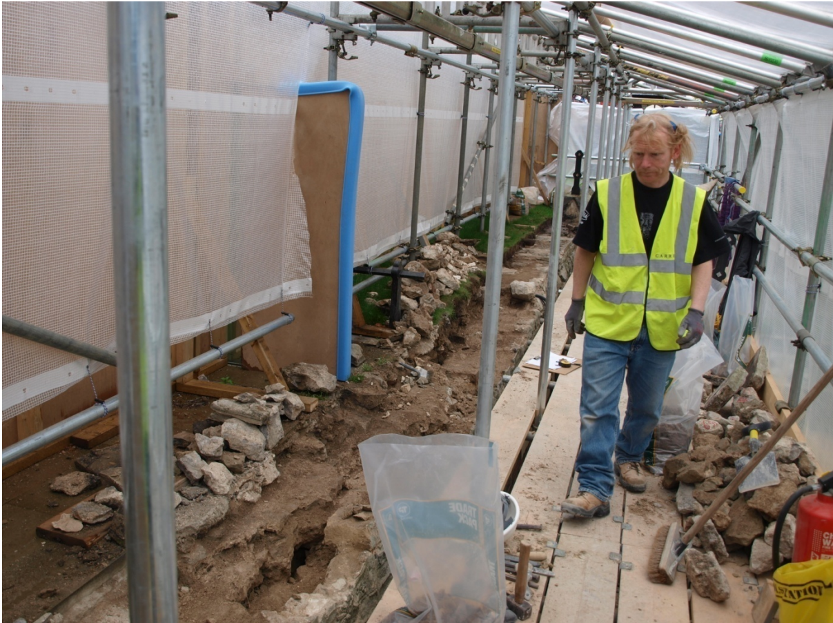
Plate 7: Dismantling of the outer face at the top of the South Moat Wall, looking east
