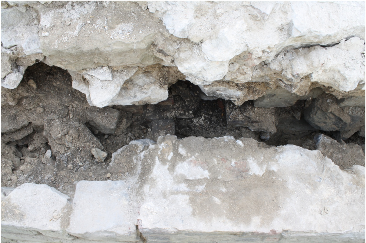
Plate 27: Plan view of Flue 2 during dismantling, looking down and south
