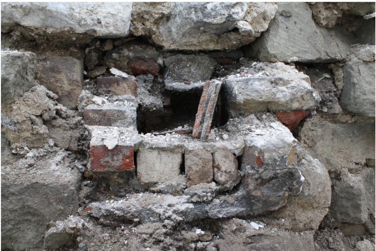
Plate 32: Flue 3 during dismantling, looking south
