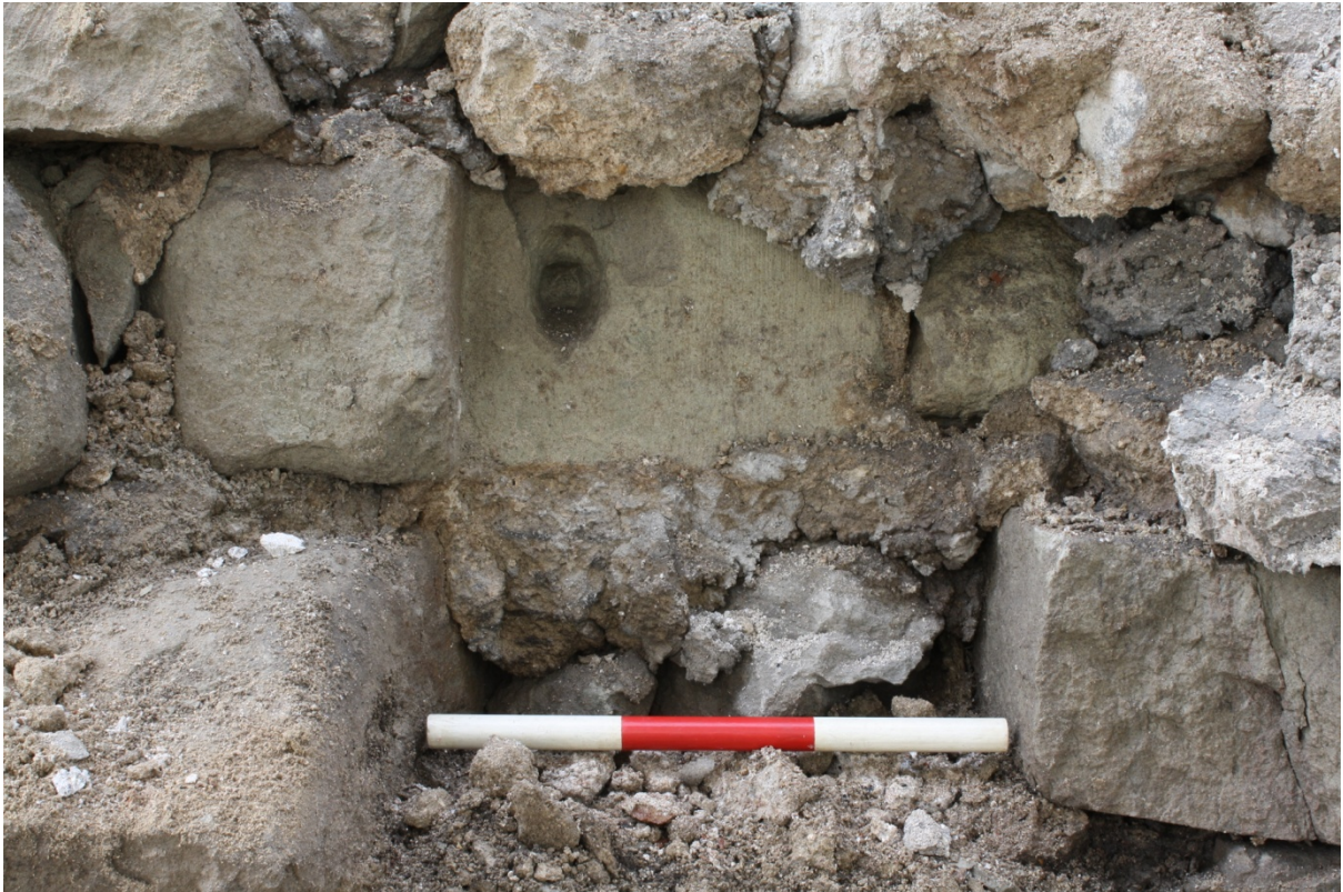
Plate 15: Worked Reigate stone within the inner rubble core, looking south
