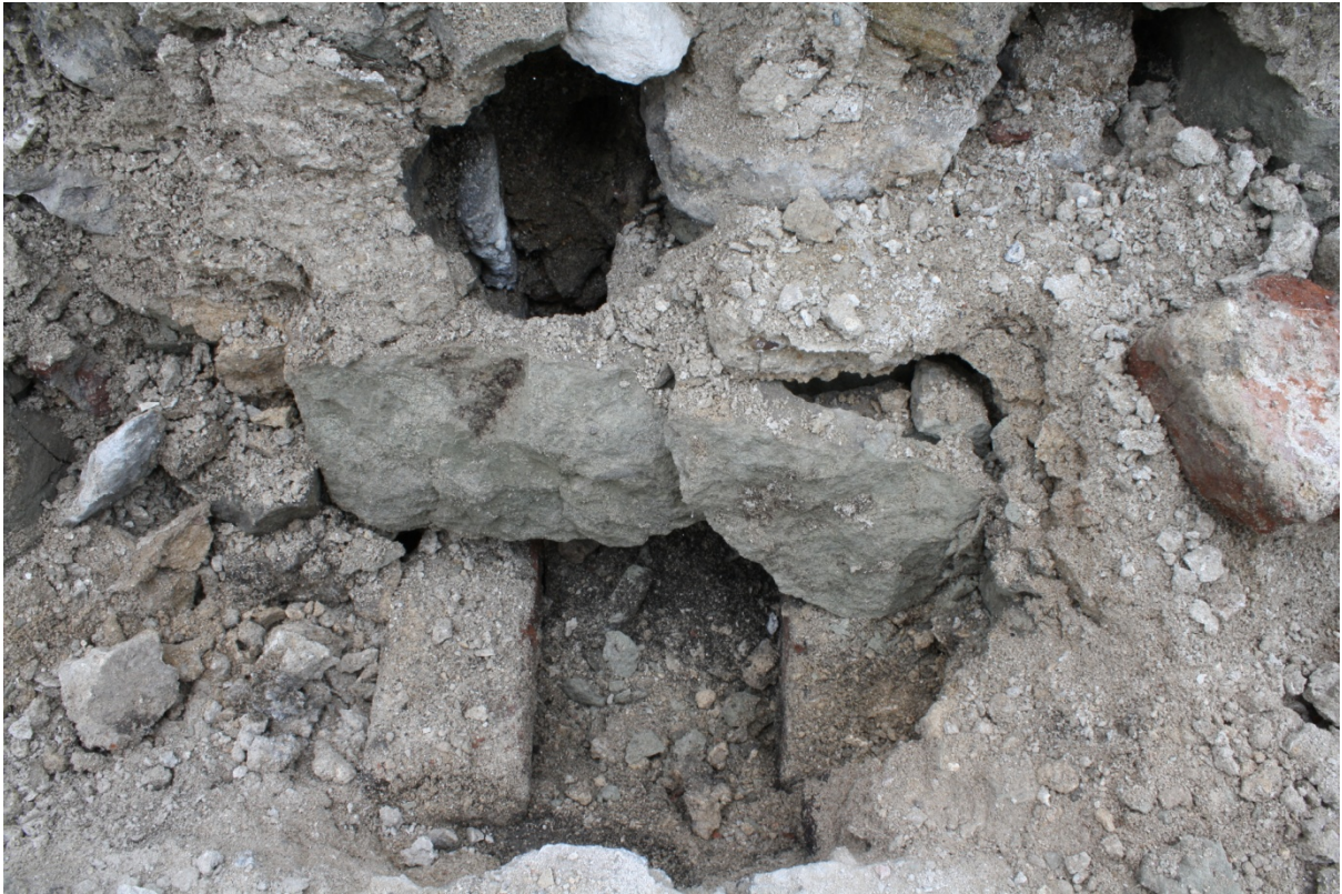
Plate 29: Plan view of Flue 2 during dismantling, looking down and south
