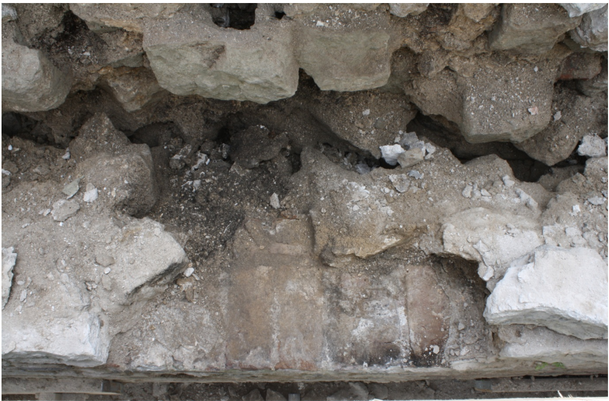
Plate 30: Plan view of Flue 2 during dismantling, looking down and south
