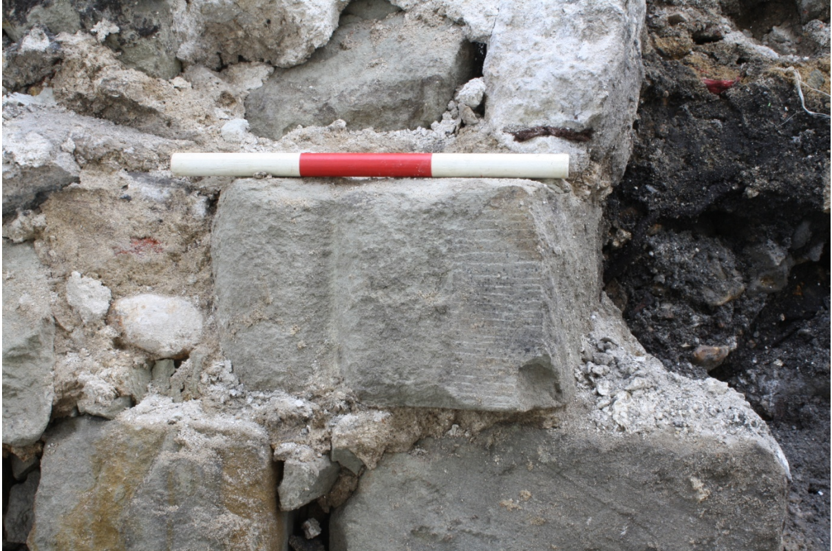
Plate 14: Reigate stone with medieval roll-holl moulding within the inner rubble core to the east of Flue 1, looking south
