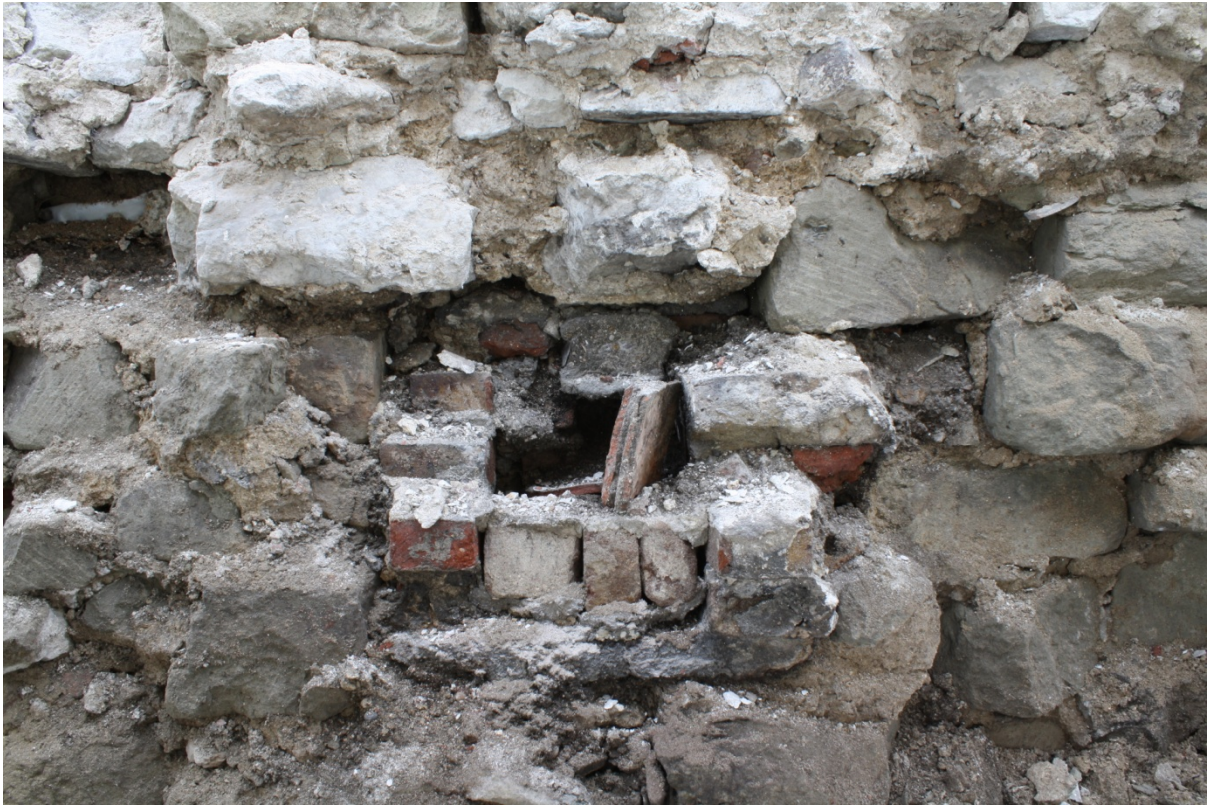
Plate 31: Flue 3 during dismantling, looking south
