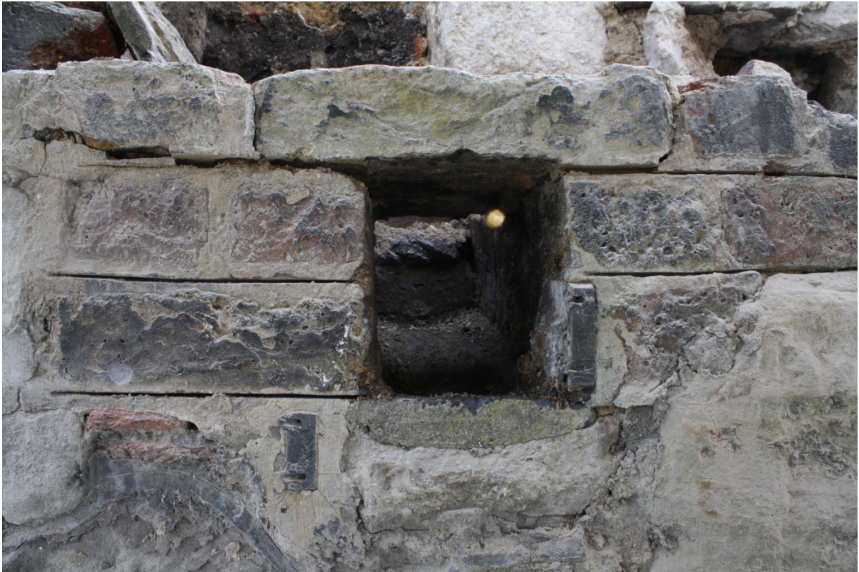
Plate 23: North elevation of Flue 1 during dismantling, looking south
