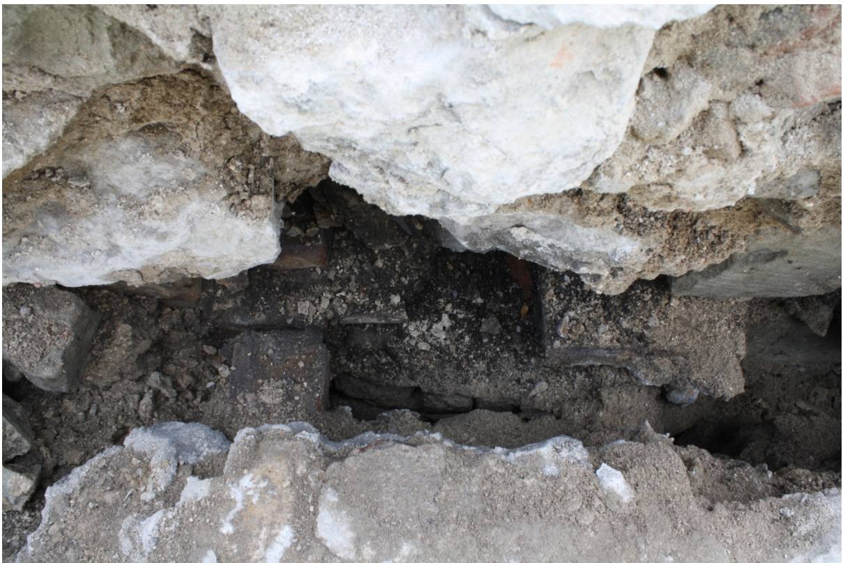
Plate 28: Plan view of Flue 2 during dismantling, looking down and south
