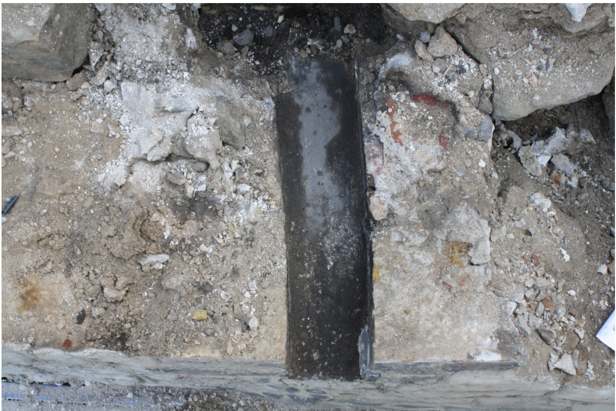
Plate 24: Plan view of Flue 1 during dismantling, looking down and south
