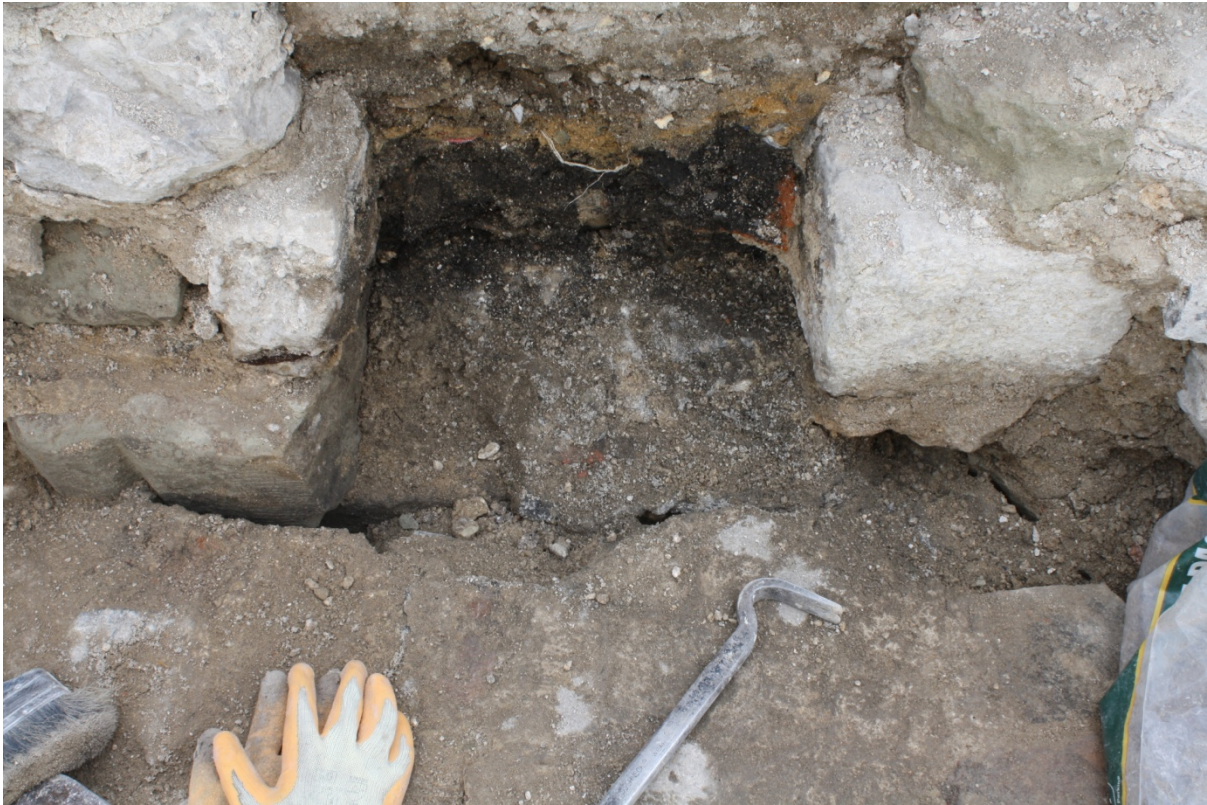
Plate 19: Plan view of Flue 1 during dismantling, looking down and south
