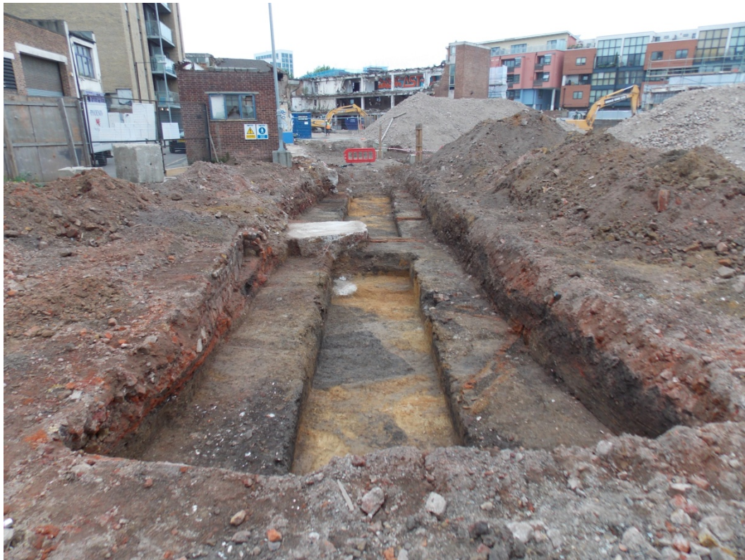
Plate 3: Overview of Trench 4, Looking West.
