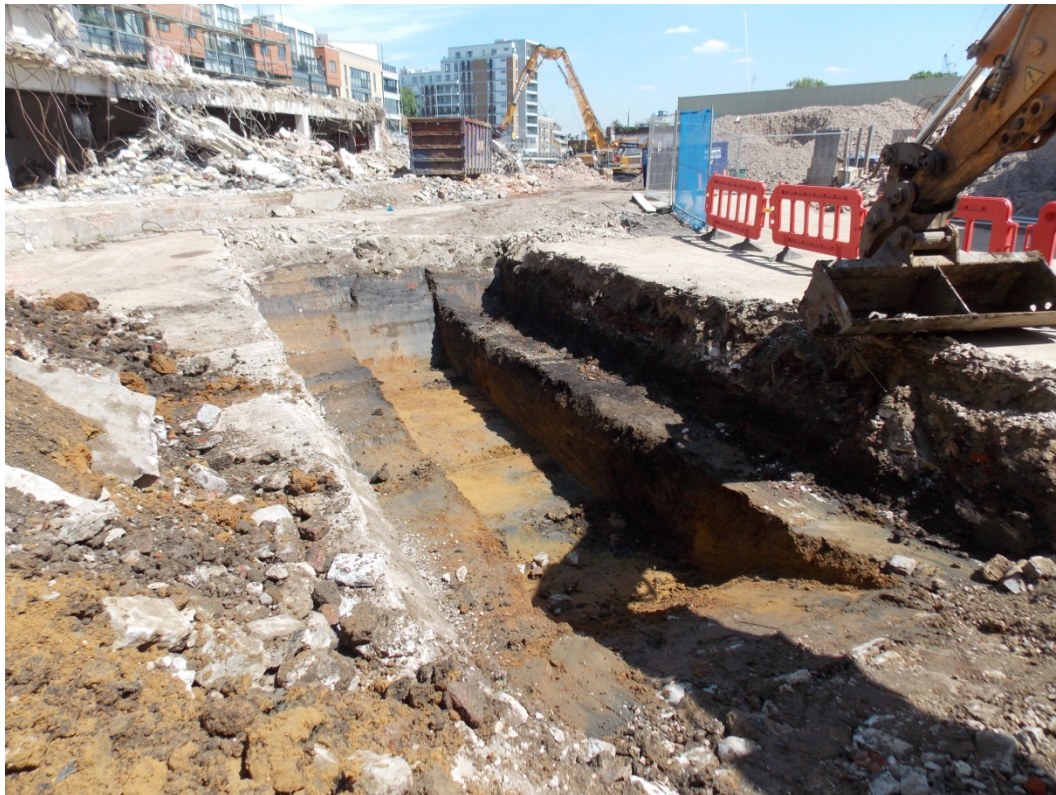
Plate 1: Overview of Trench 1, Facing Northeast.
