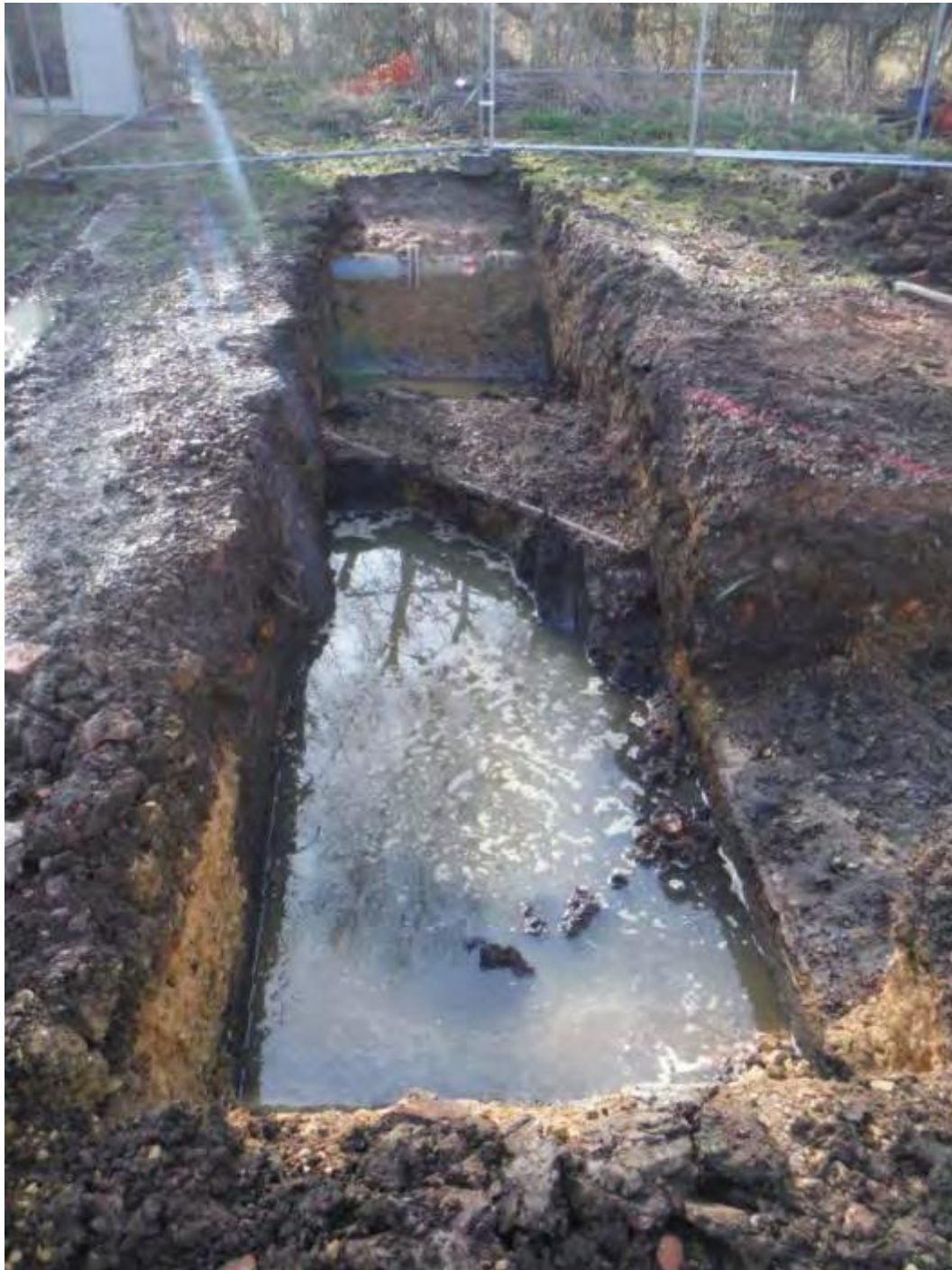
Plate 10 Looking south along initial trench (Trench 1). Modern disturbance and pipes visible in the background.
