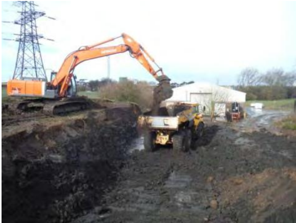
Plate 3: Ground reduction in area of deep sand bed, looking N
