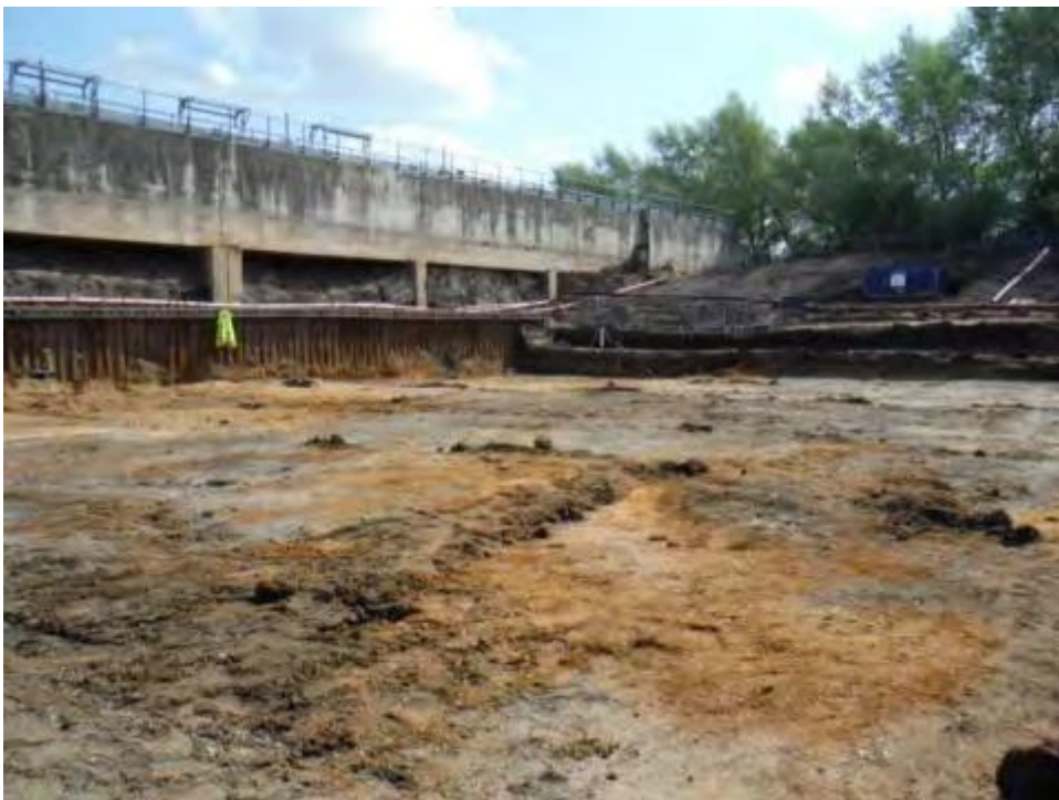
Plate 6 Final excavation level showing terrace gravels looking SE
