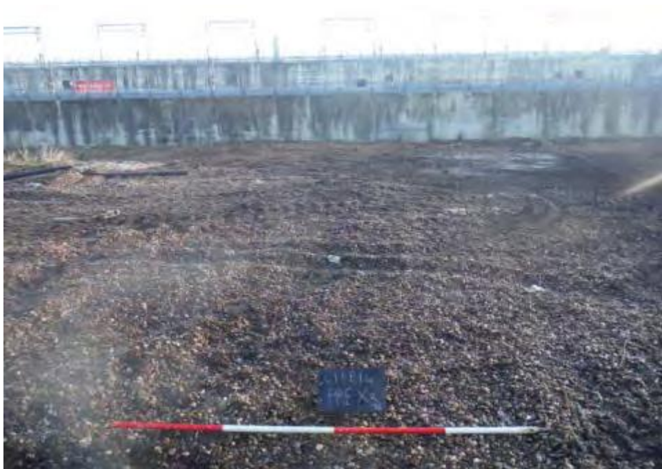
Plate 4 Pre-excavation looking north east toward water treatment tanks
