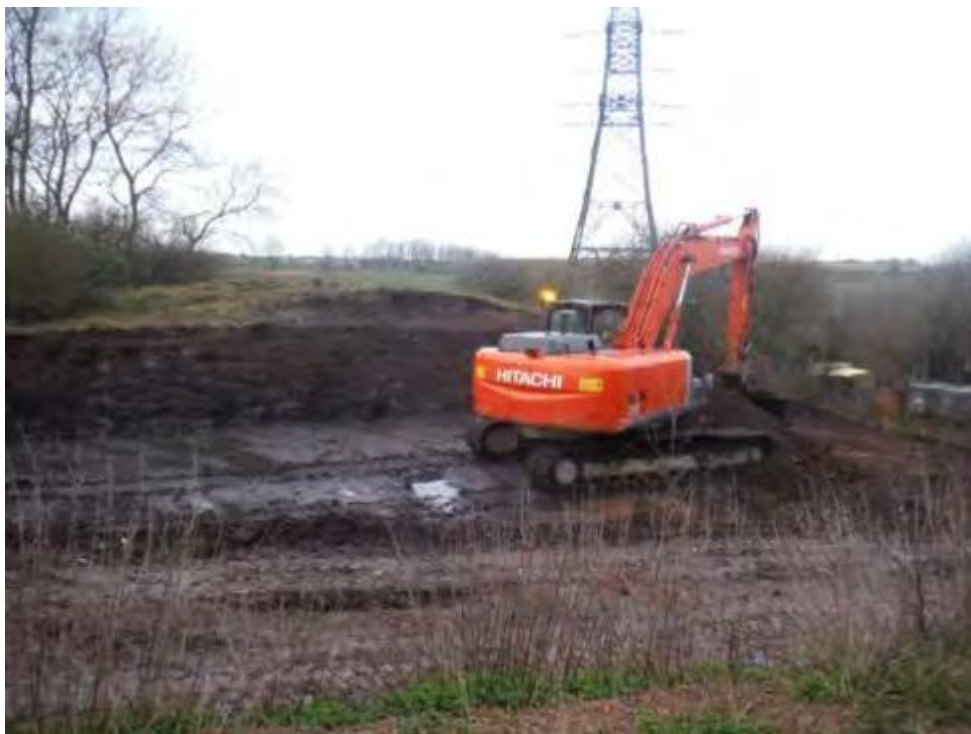
Plate 2: Initial removal of modern overburden looking NW.
