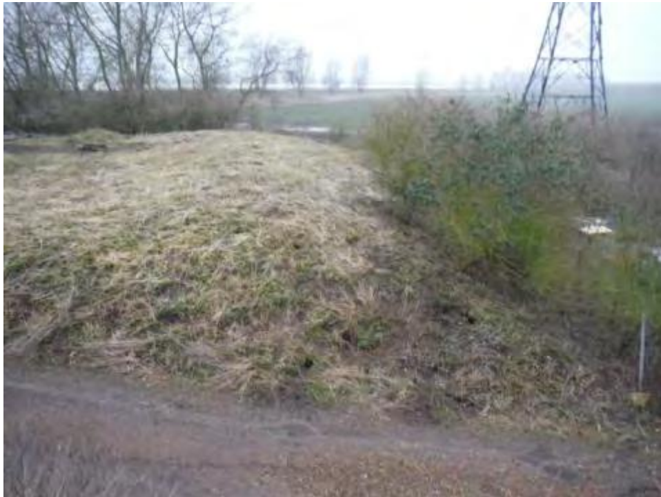
Plate 1: The location of the deep bed sand filter overlain by a modern soil bank.
