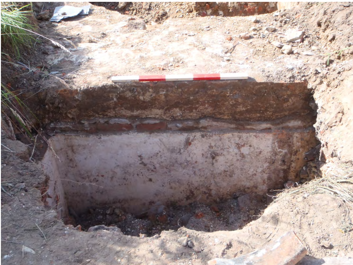
Plate 8 South facing elevation of internal face of [12] (showing plastering dropping down into cellar)
