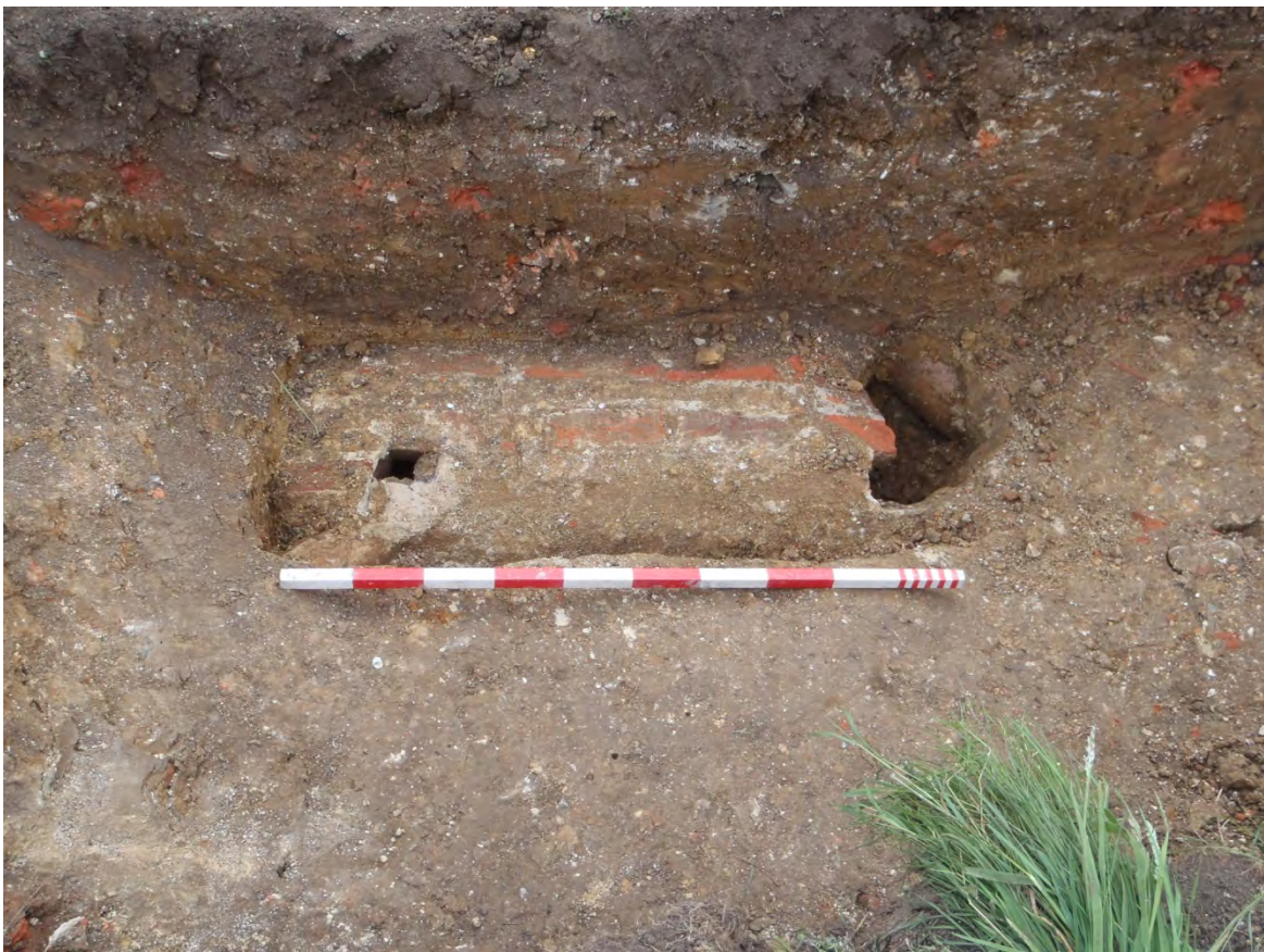
Plate 6 South facing plan shot of brick culvert [5]
