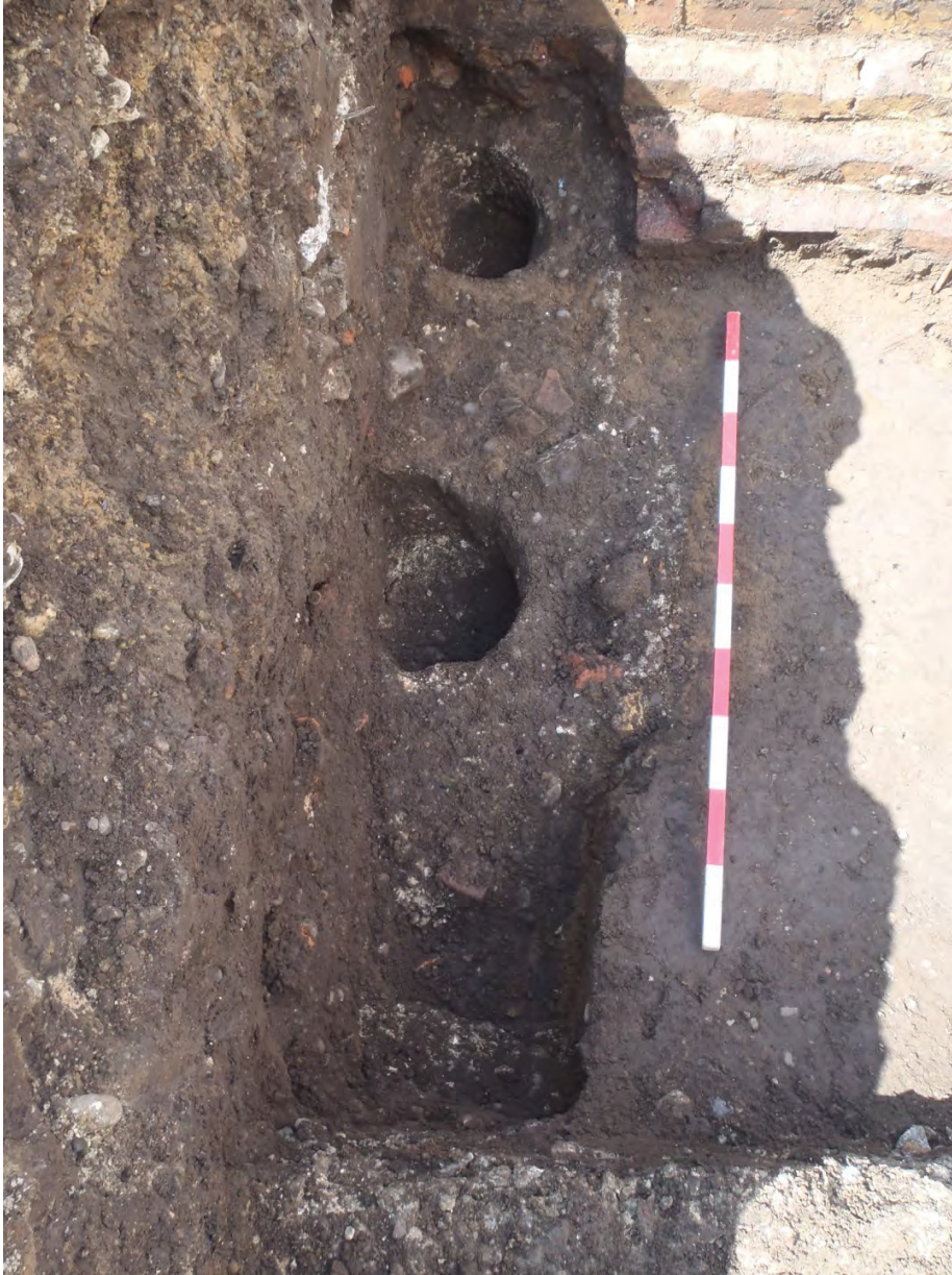
Plate 5: Concrete foundation [13] in Trench 3 facing west, 1m scale
