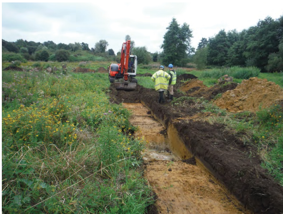
Plate 3: Trench 4, view south
