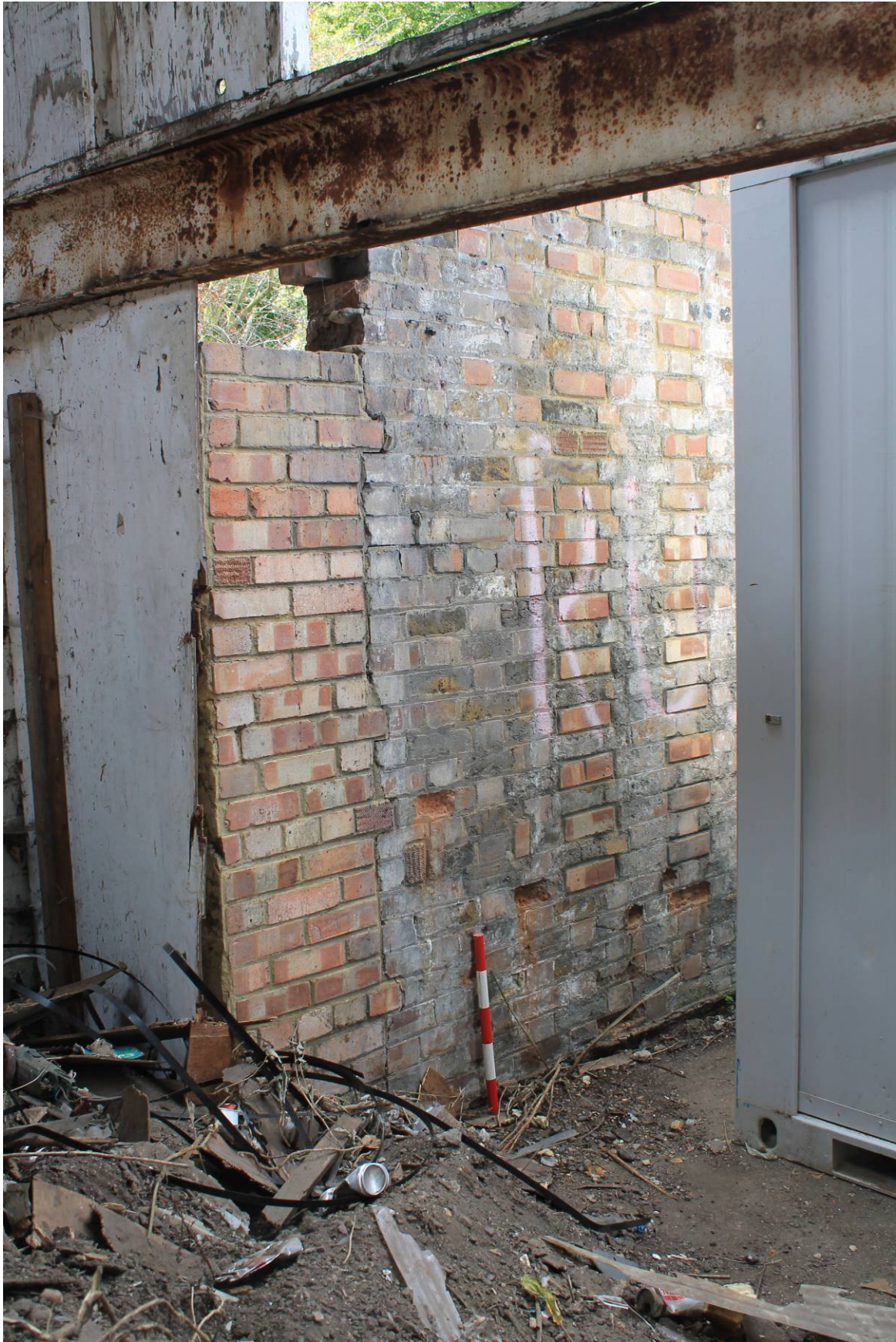
Plate 10 Fletton and re-used brickwork of Wall B, looking south-west
