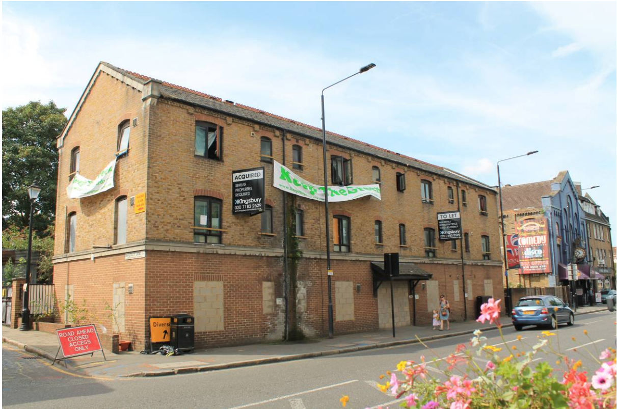
Plate 3 Building 4 No. 301 Creek Road, looking south-west
