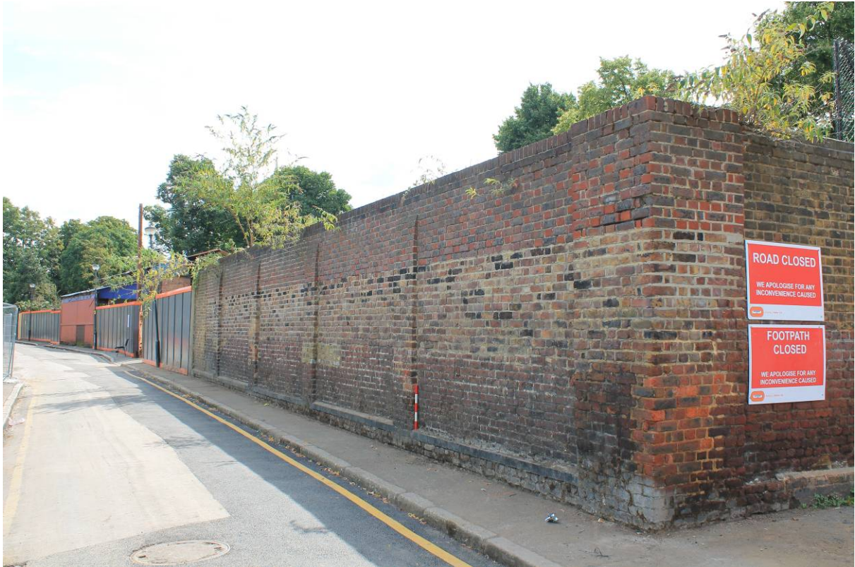
Plate 13 Wall A, looking south-east
