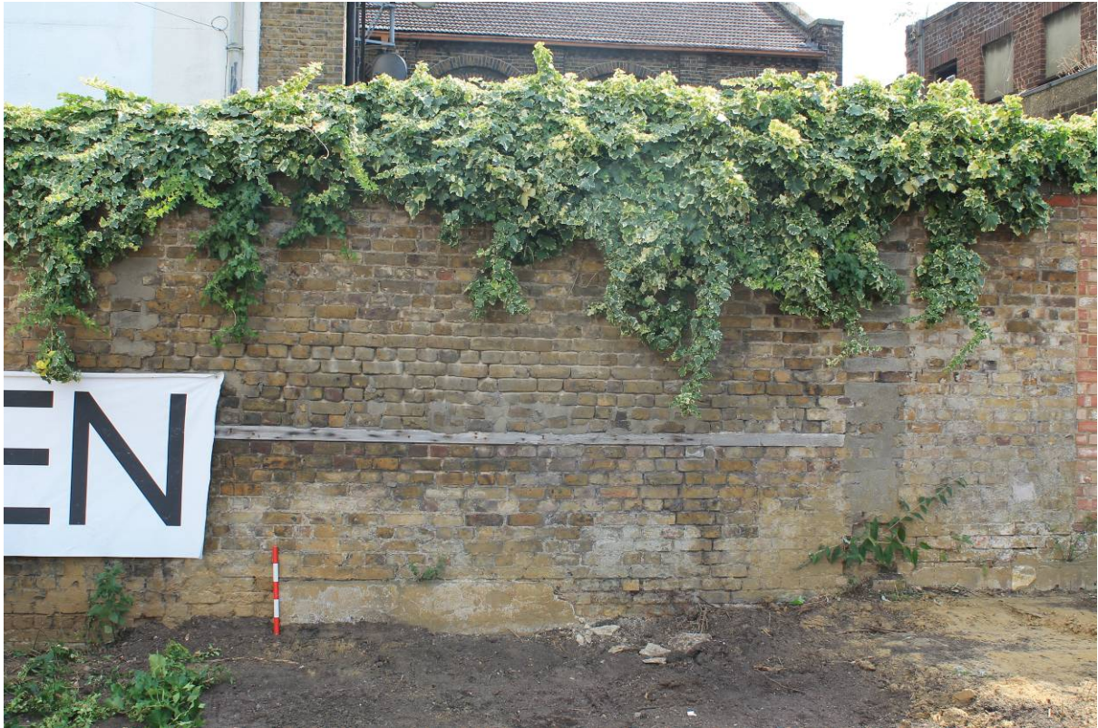
Plate 16 Wall C northern section, looking east
