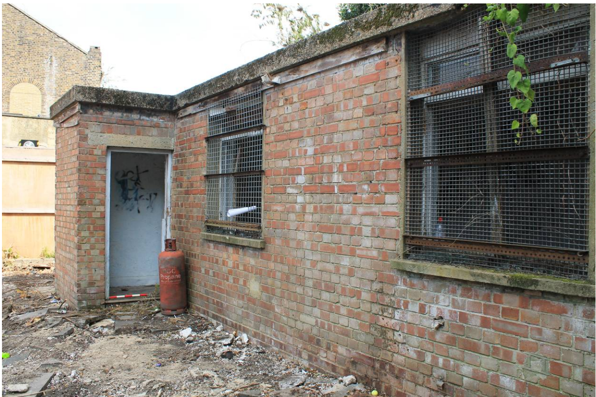
Plate 6 Building 5, looking north
