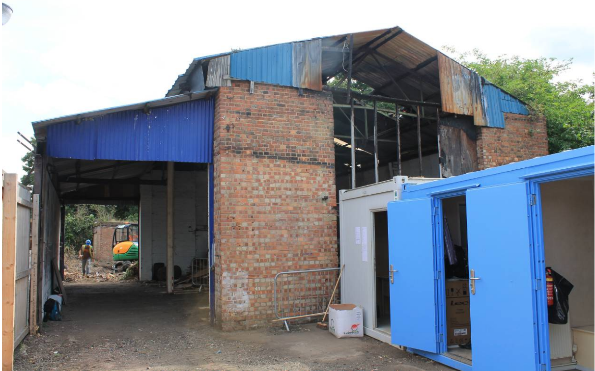
Plate 7 Building 6, looking east
