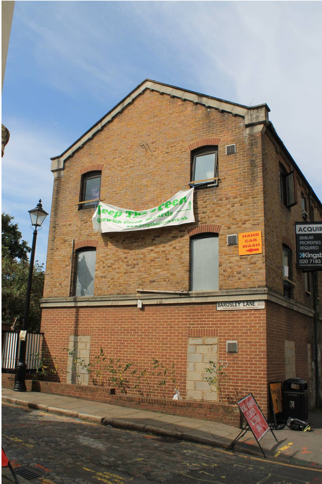
Plate 4 Building 4 No. 301 Creek Road, gable end wall, looking west
