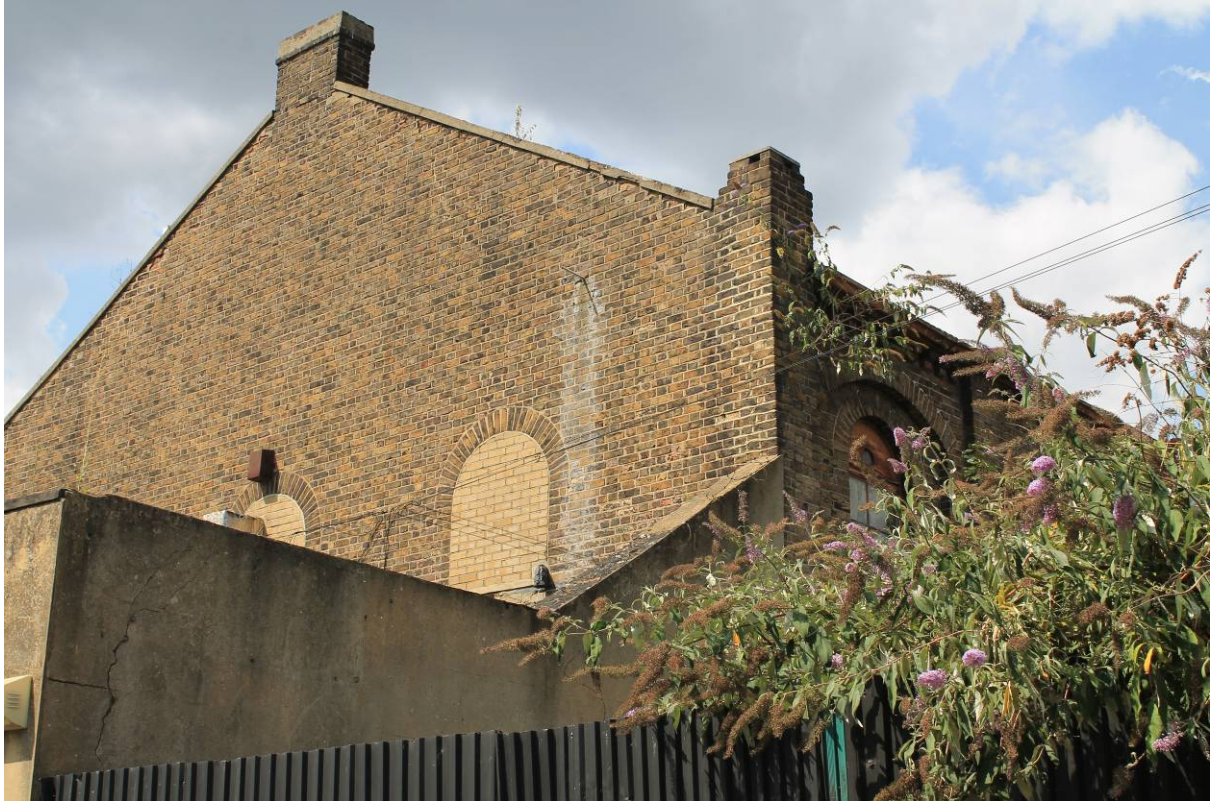
Plate 24 The Comedy Club rear southern elevation, looking north-west
