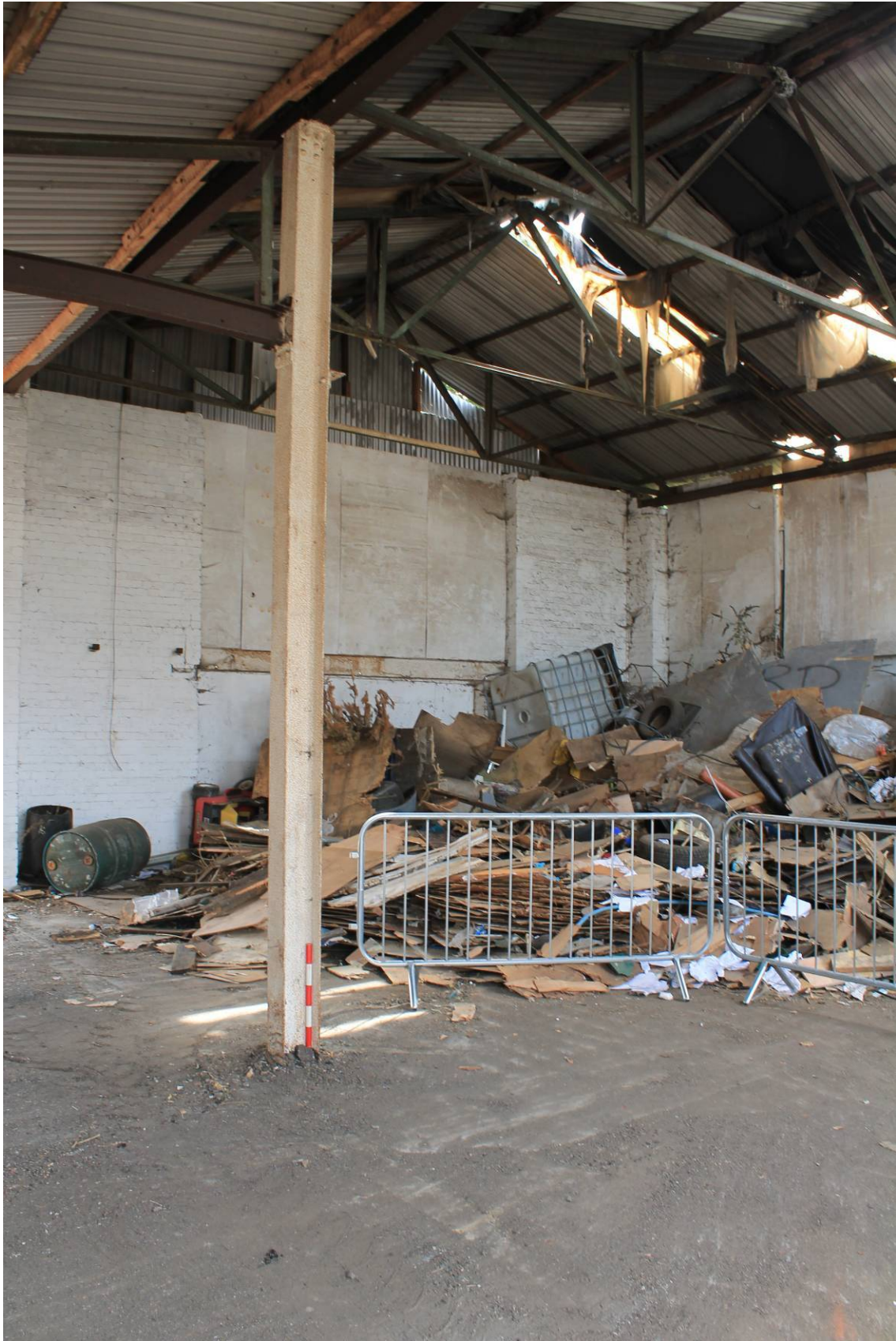
Plate 9 Building 6 internal view, looking south-east
