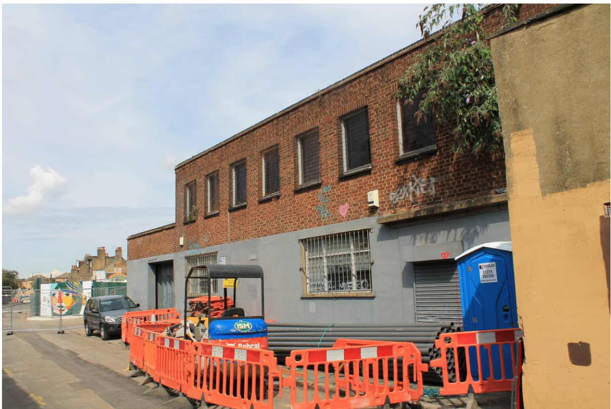
Plate 2 Building 2 south elevation, looking north-west
