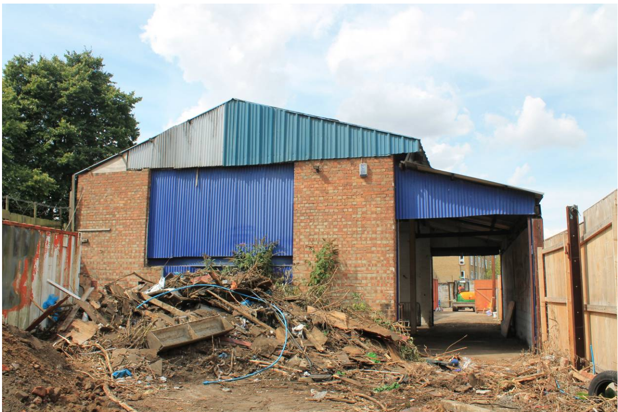
Plate 8 Building 6, looking west
