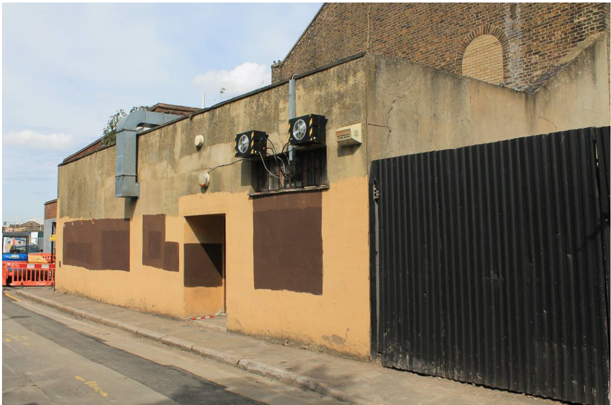
Plate 21 Building 3 extension, looking north-west
