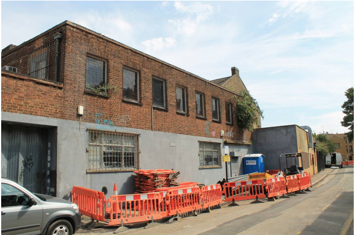
Plate 1 Building 2 south elevation, looking north-east
