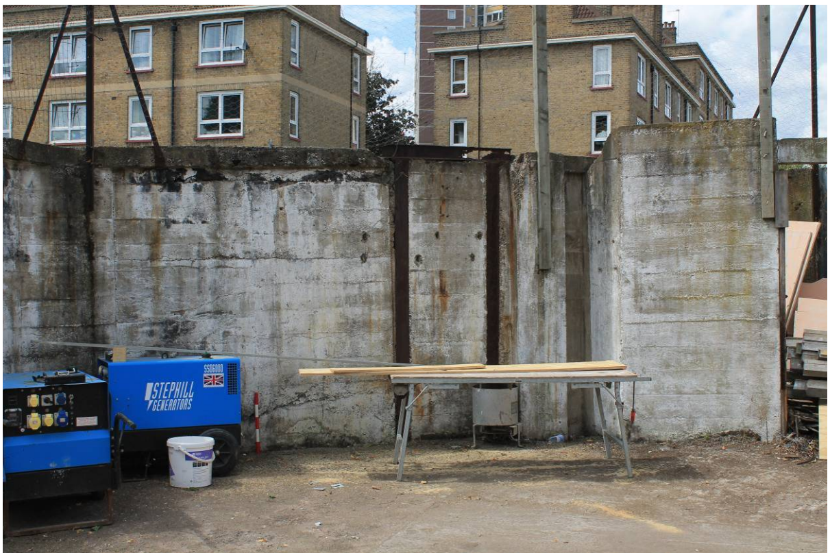
Plate 12 Concrete shuttered section of wall B(i), looking west
