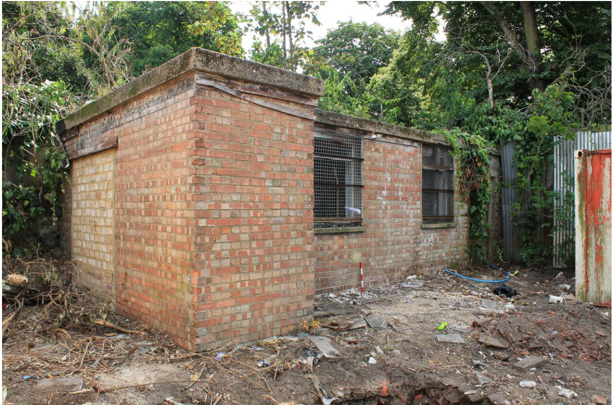
Plate 5 Building 5, looking south-east
