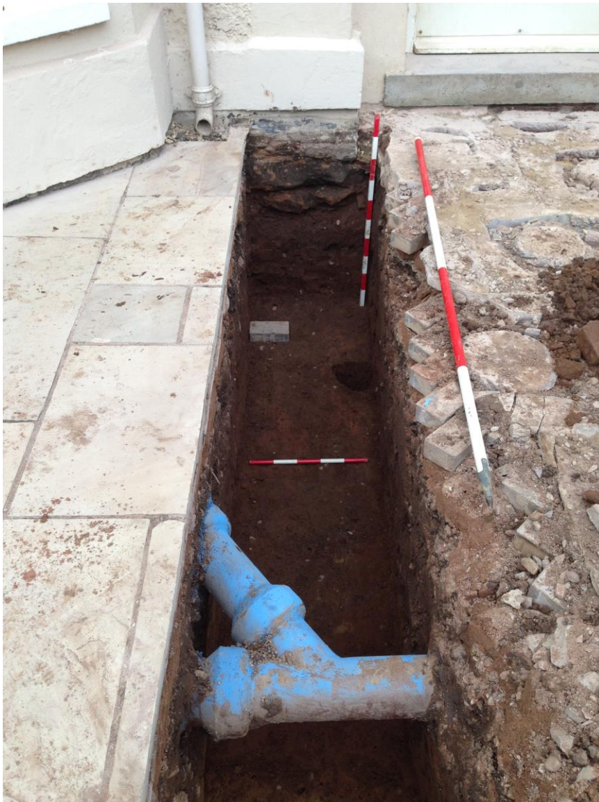
Plate 1: Stone wall footings (17) and post-hole [15] looking west.
