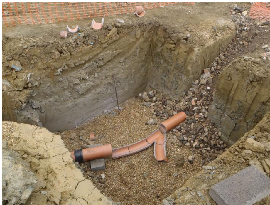
Plate 5: Excavation for manhole construction during drain-laying in north of site.
