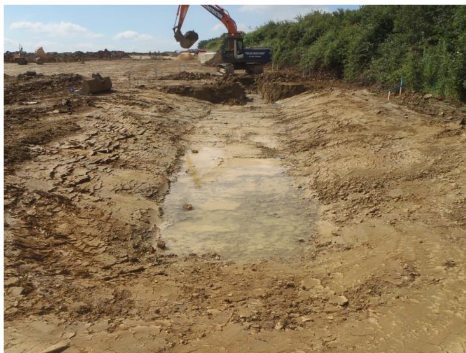
Plate 2: Excavation of Swale 1, looking south.
