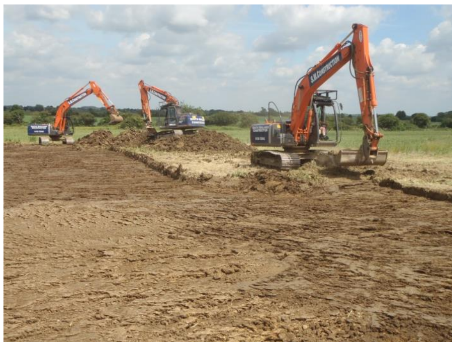
Plate 1: Topsoil strip, looking northeast
