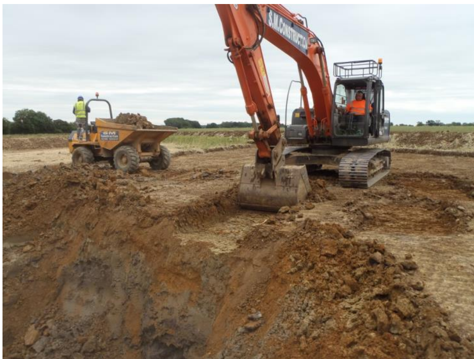
Plate 3: Excavation of swale 2, looking northeast
