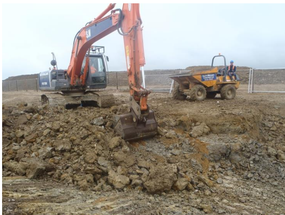
Plate 4: Excavation of swale 3, looking southeast.
