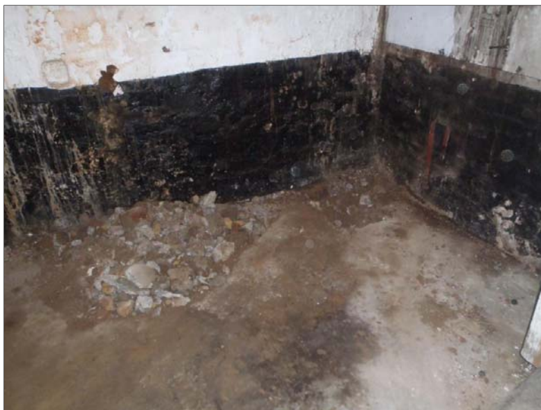
Plate 10: TP6 Original (left) and Relocated (right) Positions, Looking South-East
