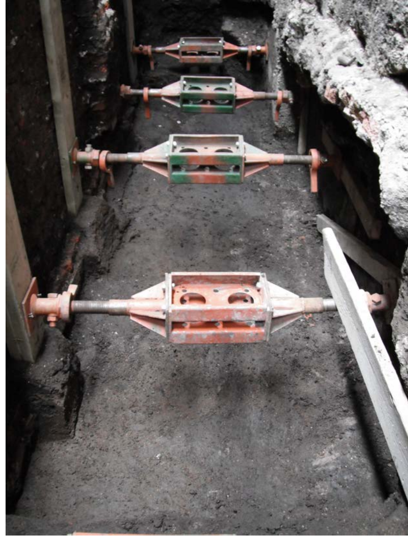
Plate 2: View to south illustrating excavation area.
