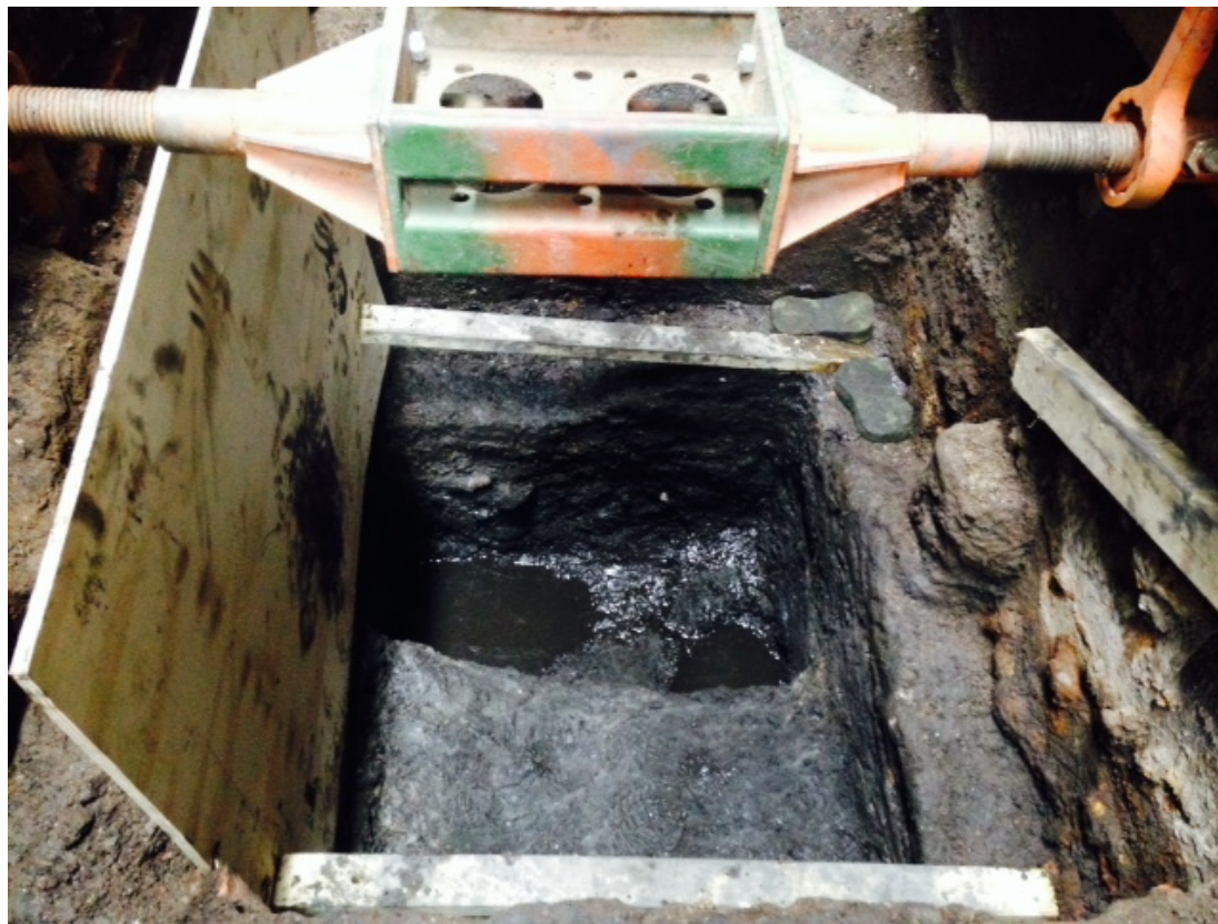
Plate 3: View to south illustrating sump area excavations.
