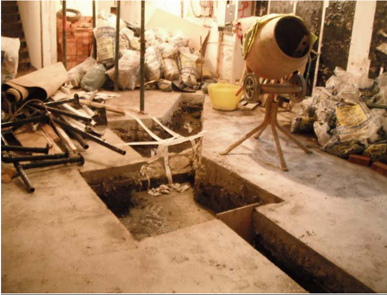
Plate 1: View to north-west illustrating basement area trenches.
