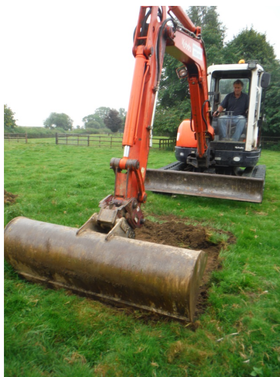
Plate 2: Machine excavation Trench 2
