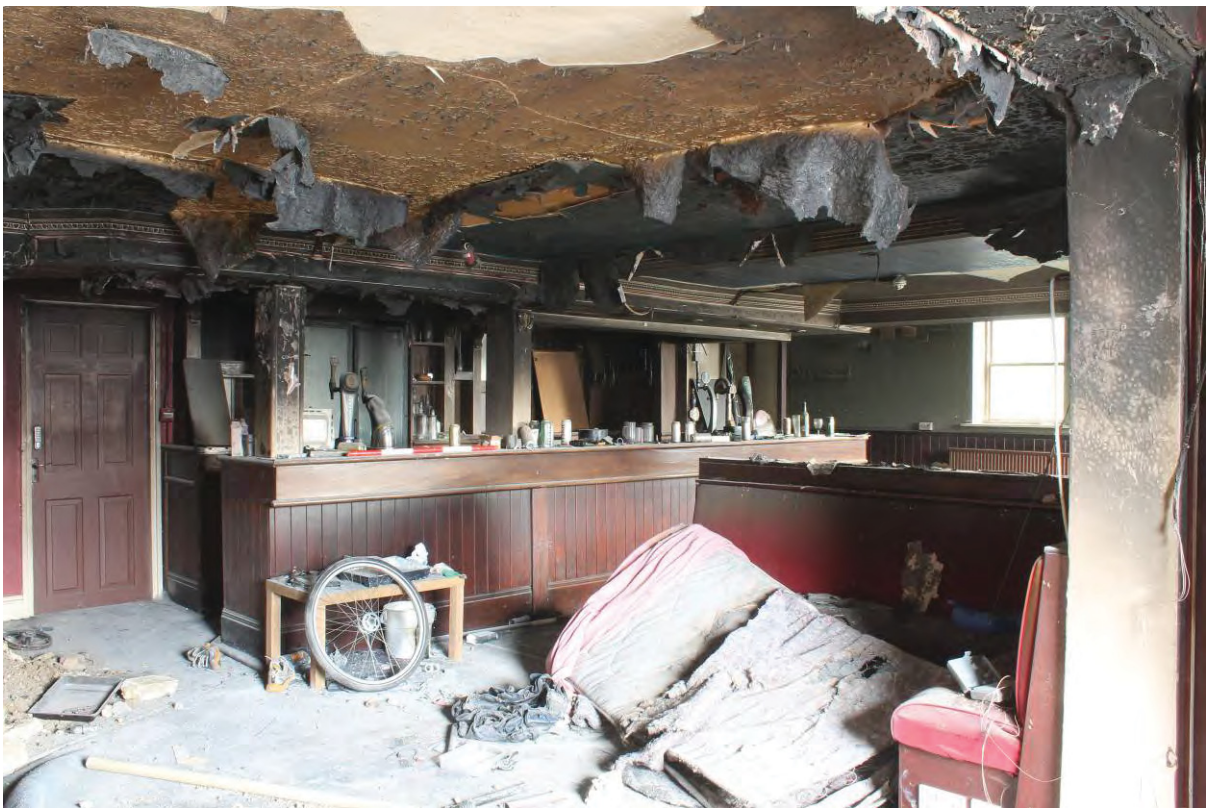
Plate 7 Bar Area G1 looking North-East
