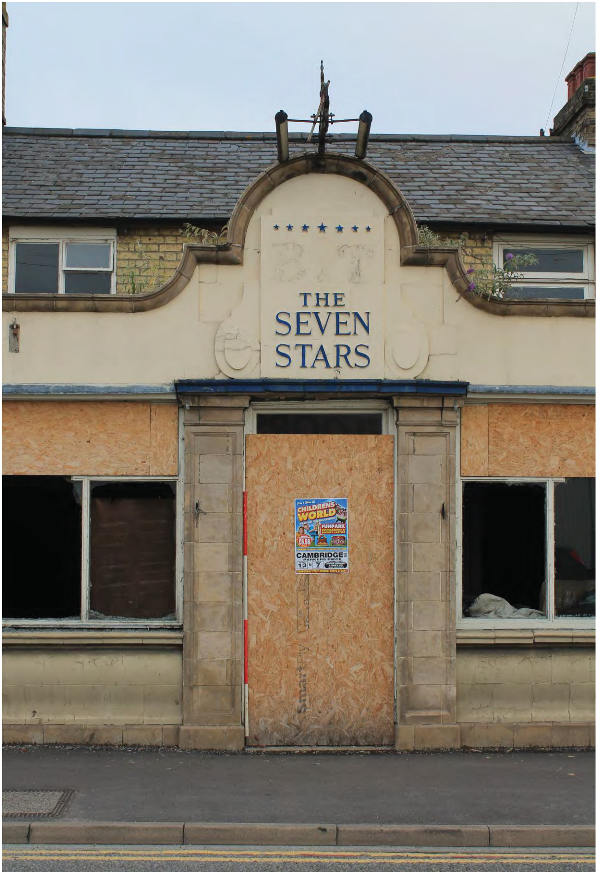
Plate 3 Detail of Entrance Bay looking North
