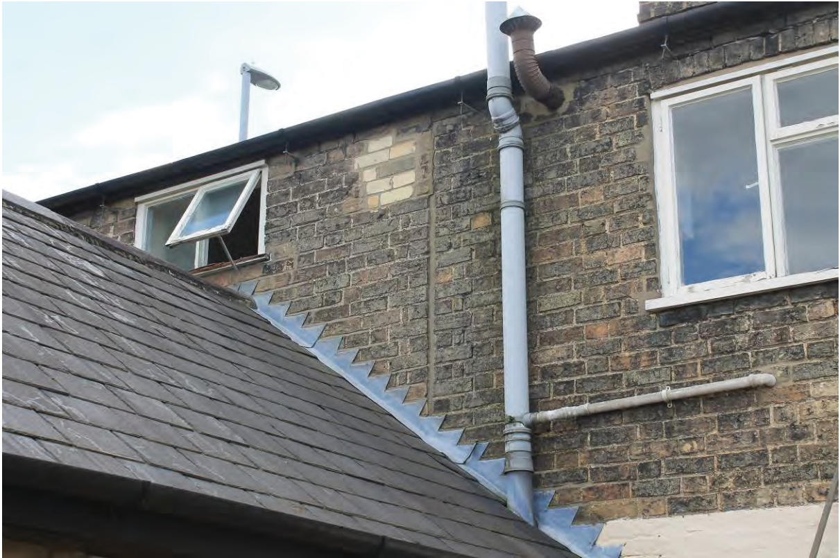
Plate 6 Straight Joint in Northern Elevation showing addition of Carriageway
