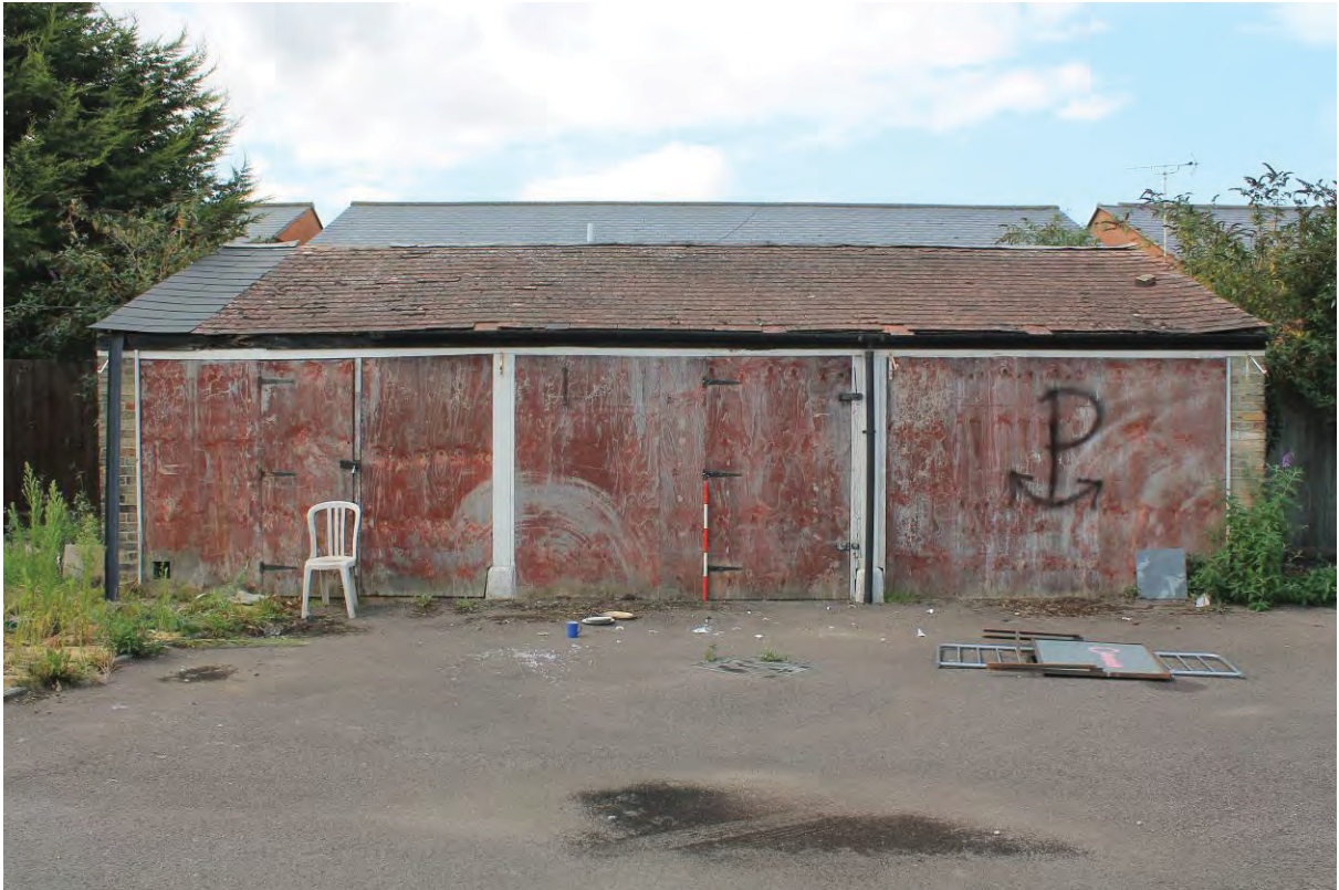
Plate 23 Outbuilding (2) looking North
