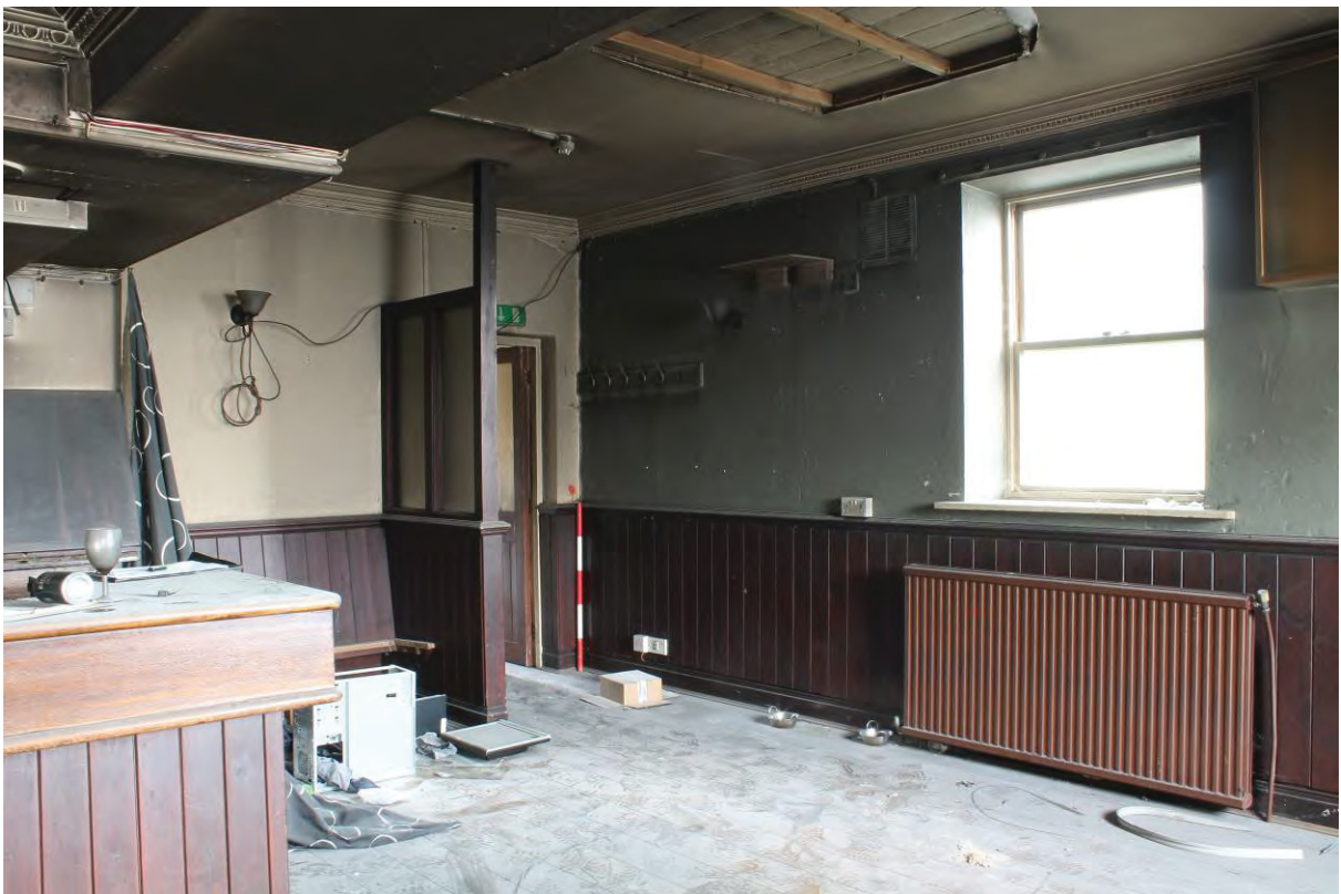
Plate 9 Bar Area G2 looking North-East
