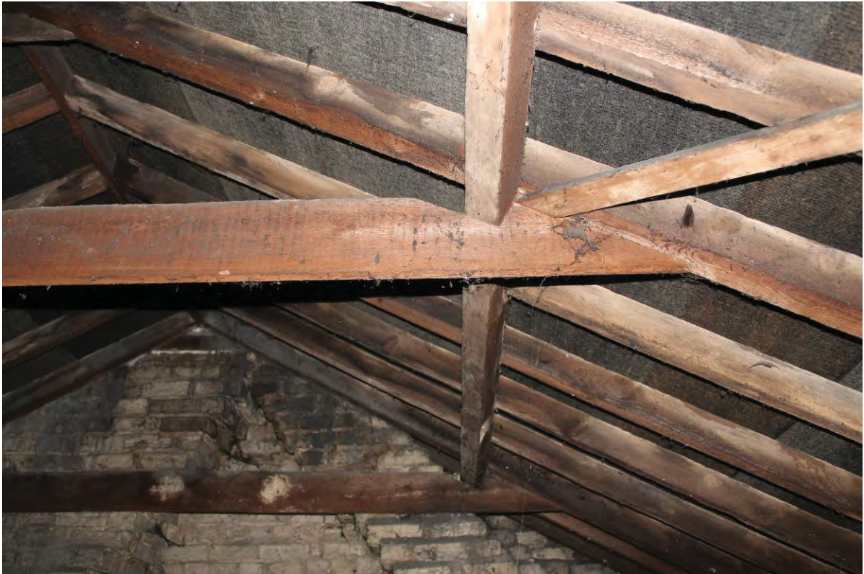
Plate 19 Clapped Purlin Roof over Western Bays
