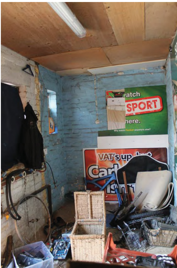
Plate 22 Interior of (1) looking South
