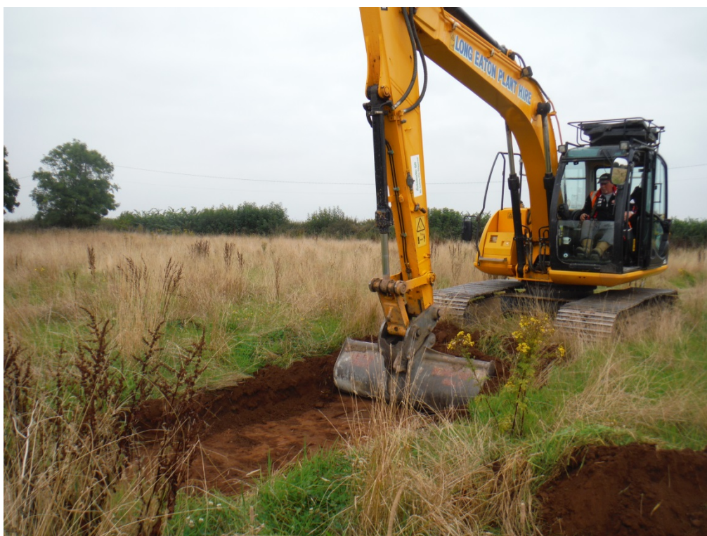
Plate 2: Machine Excavation, Trench 2
