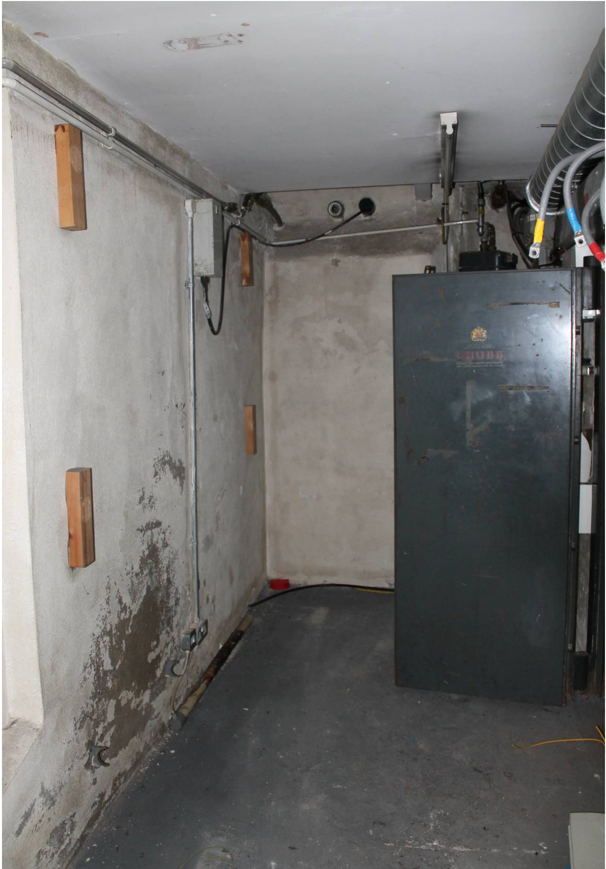
Plate 29 Room (11) looking east and showing door to strong room (10)
