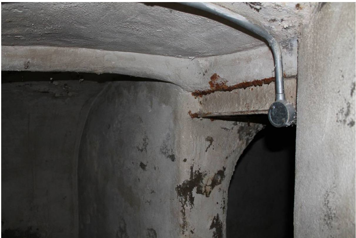
Plate 28 Barrel vault (8) looking east and showing RSJ bridge
