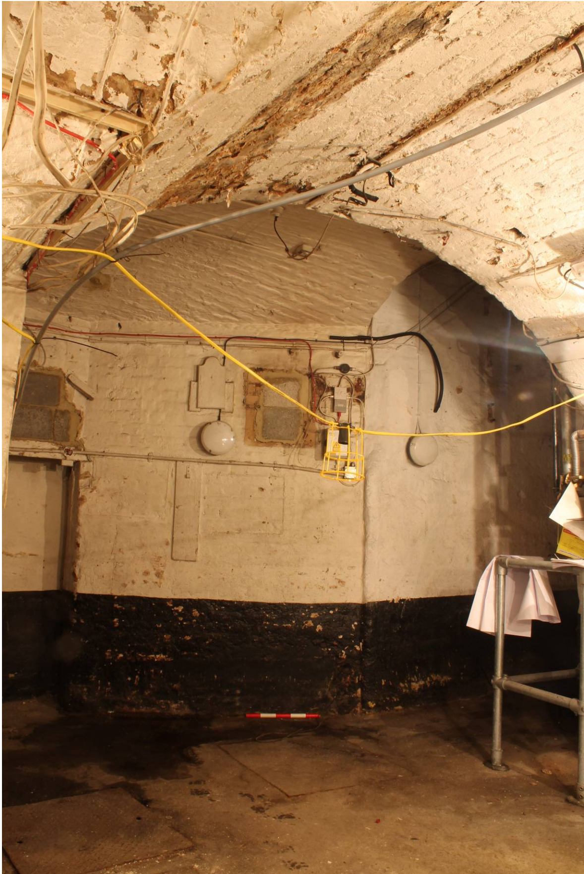
Plate 22 View from area (3) towards vaulted area (4) and barrel drop
