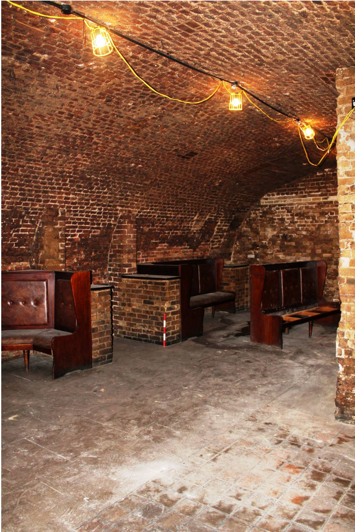
Plate 12 Basement Bar (1) showing barrel vaulted cellar, looking north-east
