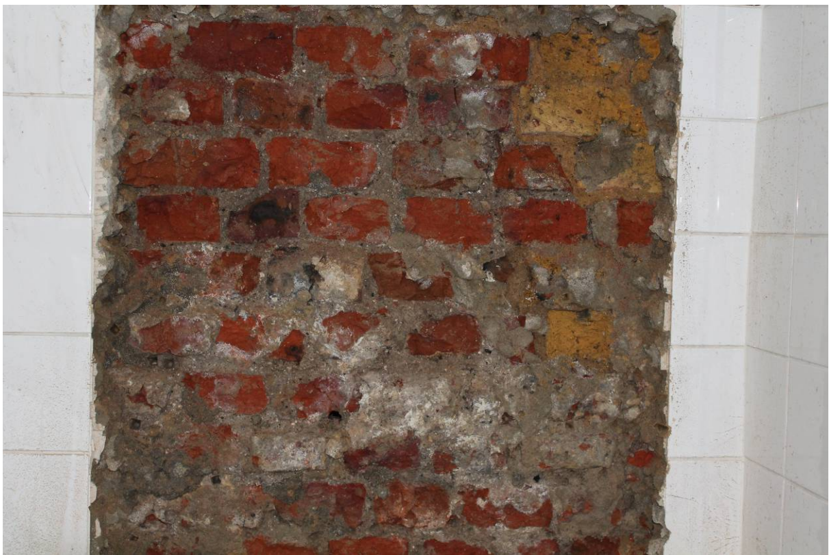
Plate 33 Observation panel in toilet cubicle (15) looking south
