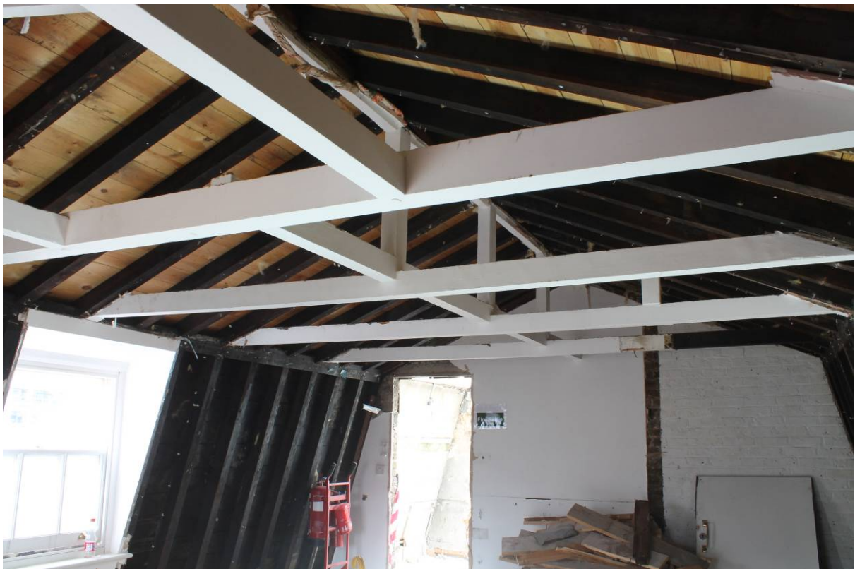
Plate 38 Later bracing to Mansard Roof structure, looking south-west towards stairwell
