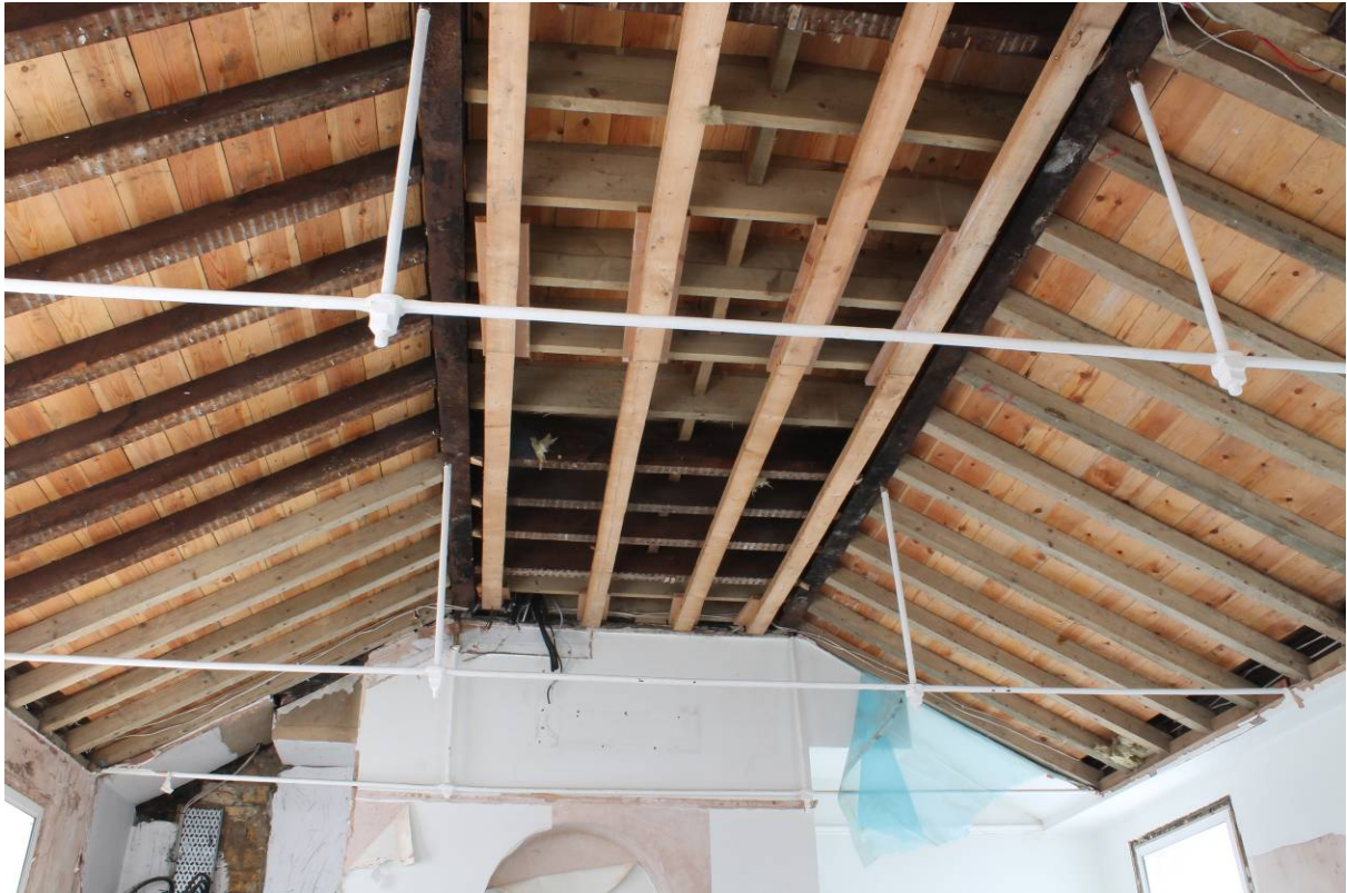
Plate 42 Rebuilt Platform Roof over 19th century west extension, looking west
