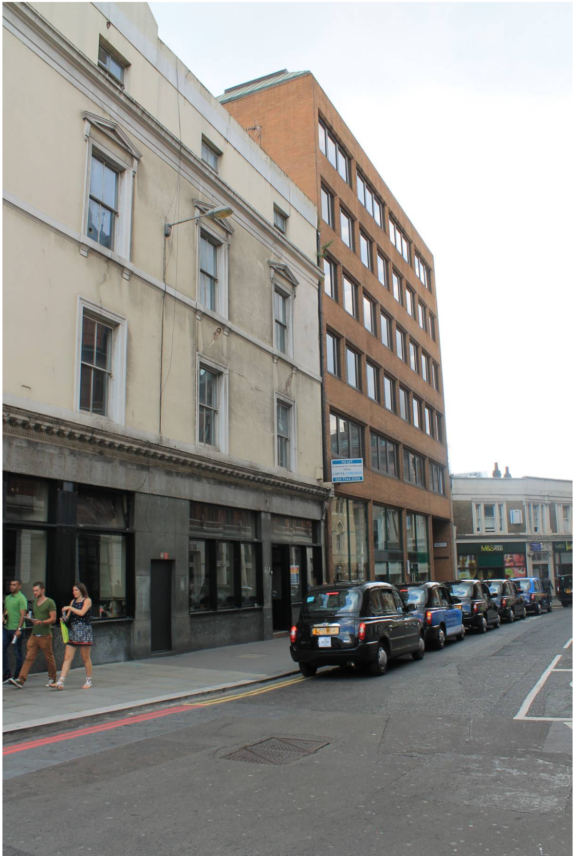
Plate 6 The White Hart Inn and Nos. 34-37 Liverpool Street, looking south-west
