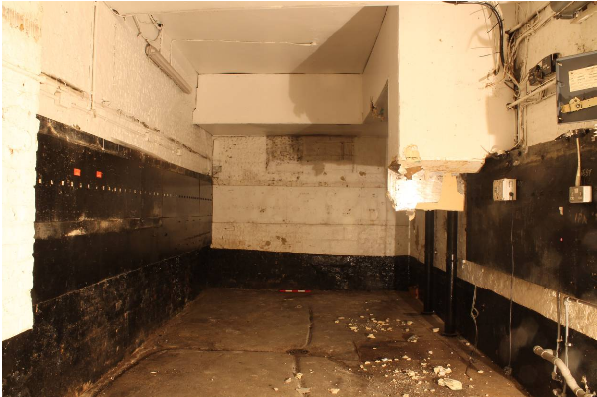
Plate 24 Cellar below No. 119 (area 7) looking west
