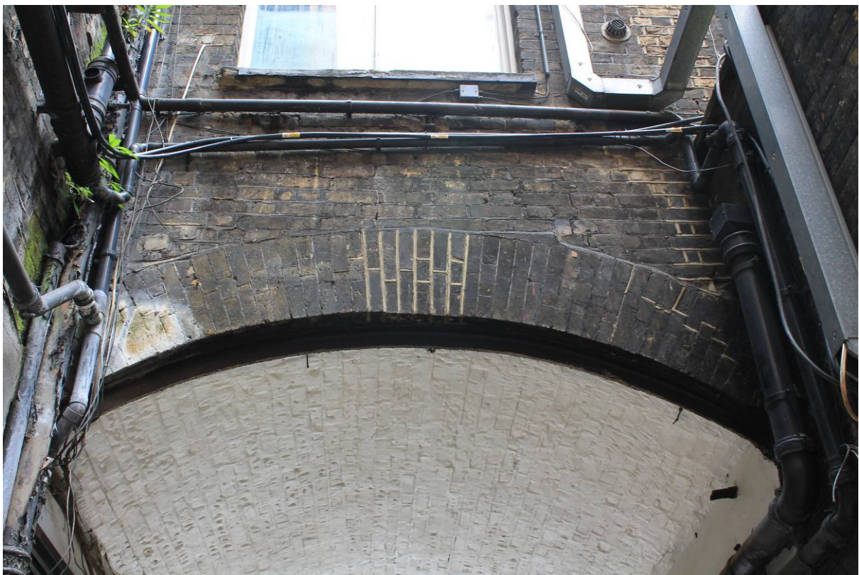
Plate 11 Brick voussoirs to rear (west/court side) of carriageway, looking east
