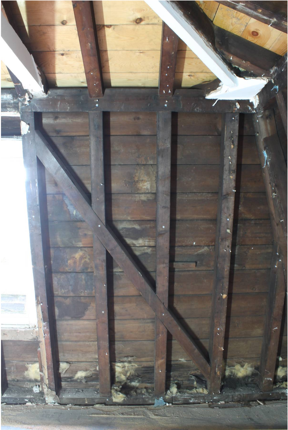
Plate 39 Detail of primary bracing, looking east
