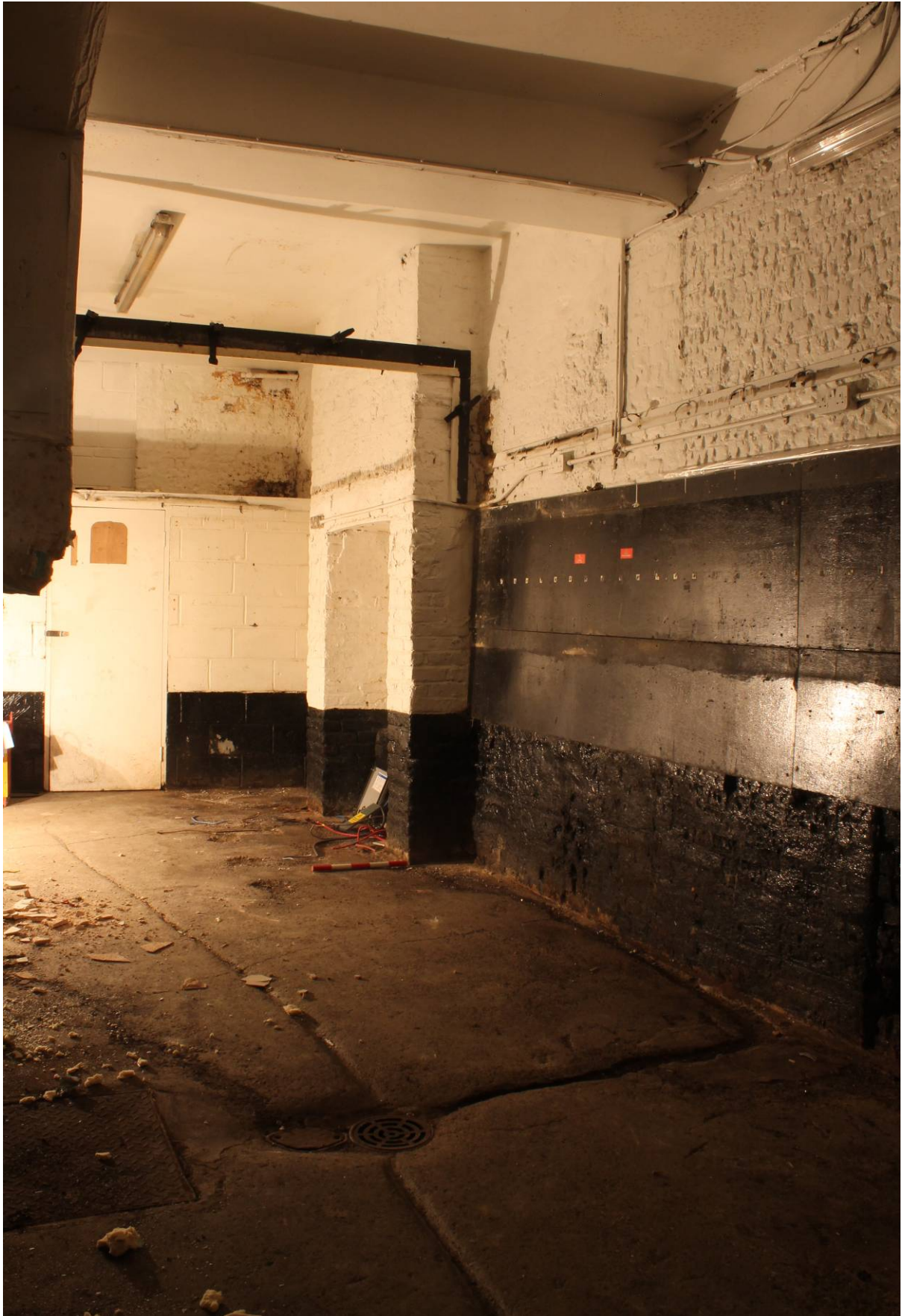
Plate 26 Cellar (7) looking south-east toward stack base and modern bottle store
