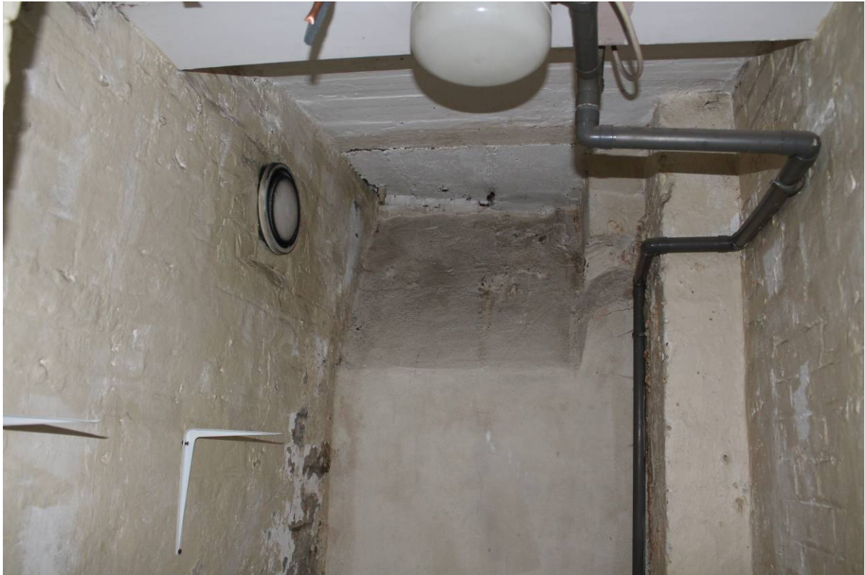
Plate 32 Jack arch and blocked coal chute or light in room (13)
