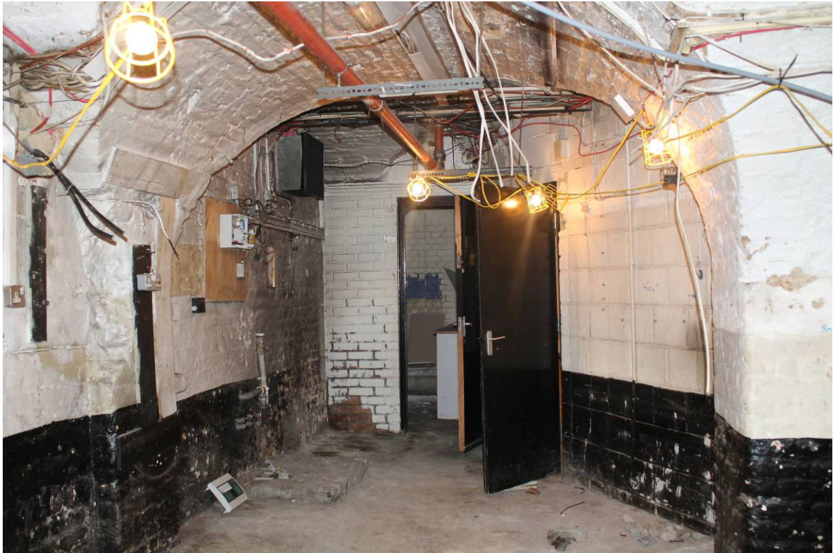
Plate 19 Vaulted basement area (3), looking west
