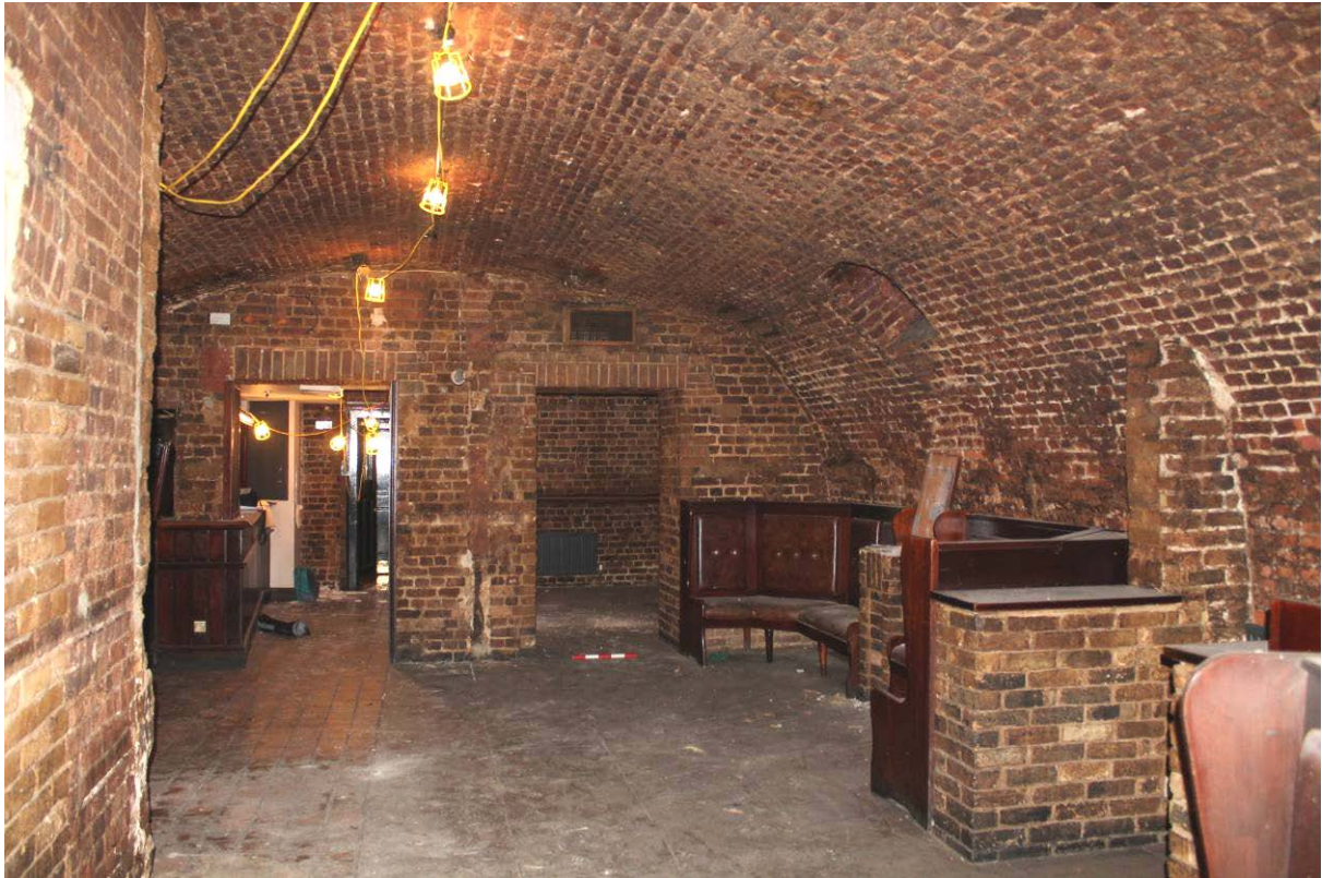
Plate 13 Basement Bar vault (1), looking west toward Bar Area (2), looking west
