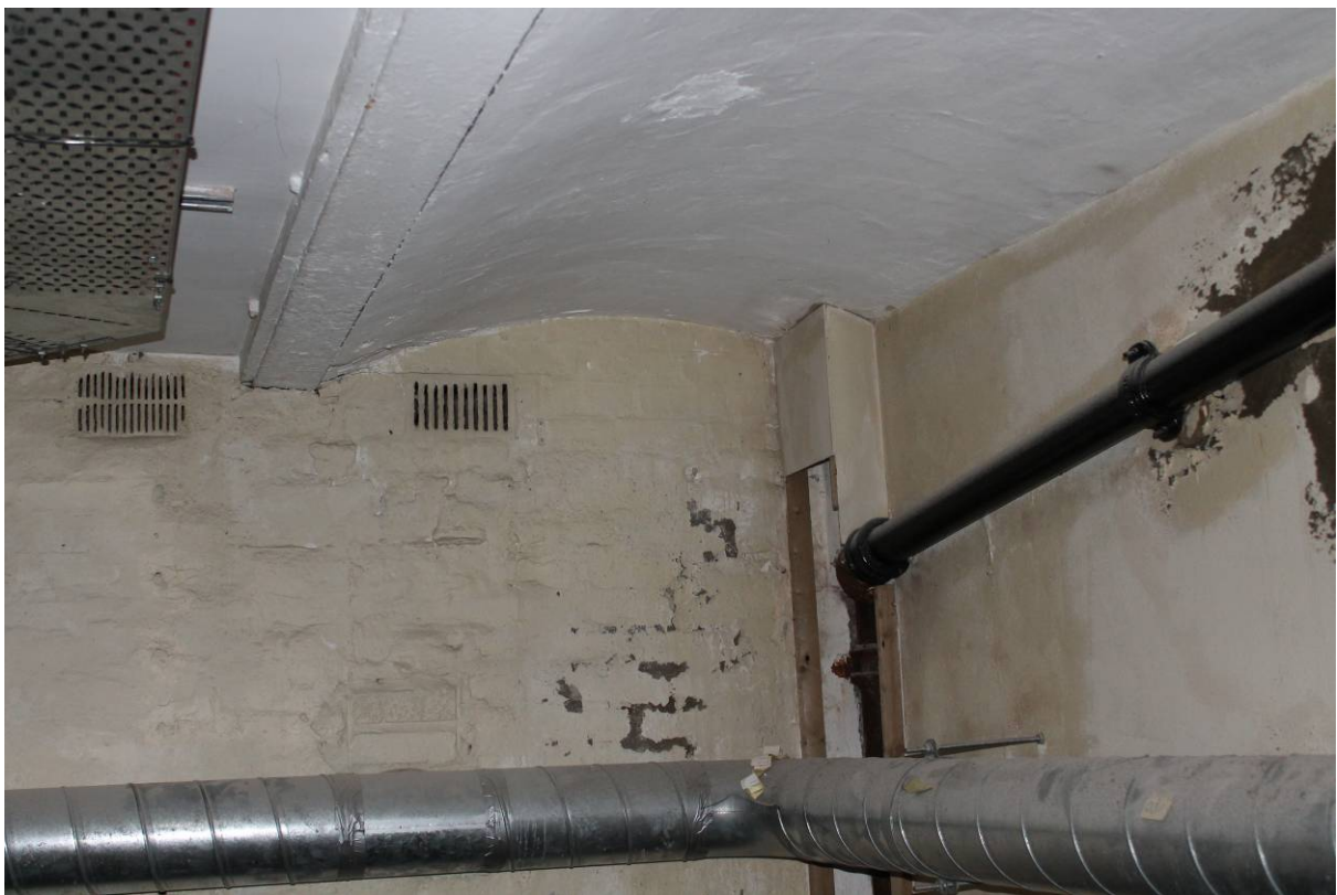
Plate 31 Jack arch vault in (12) looking east
