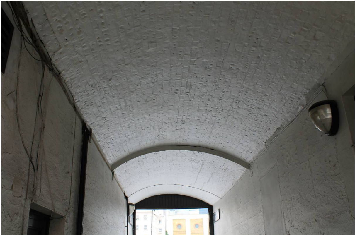
Plate 10 Carriageway arch looking east towards Bishopsgate
