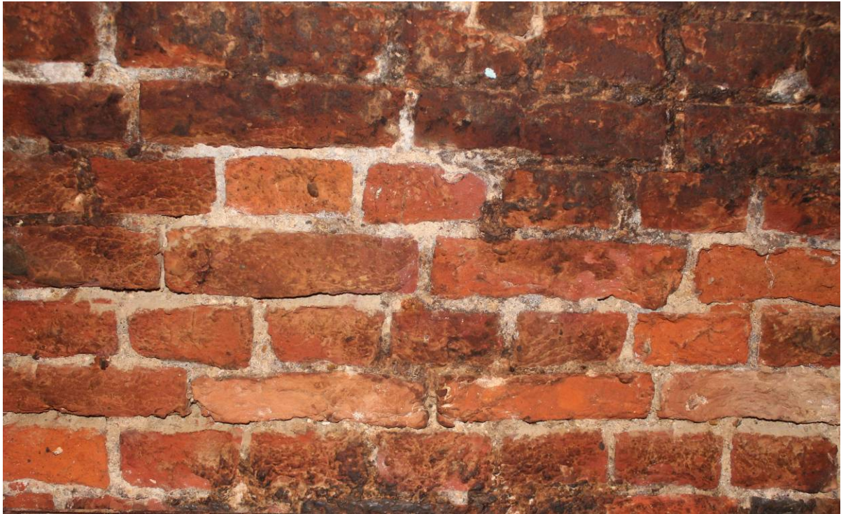
Plate 16 Detail of 17 th century brickwork (BB) to barrel vault, looking north.
