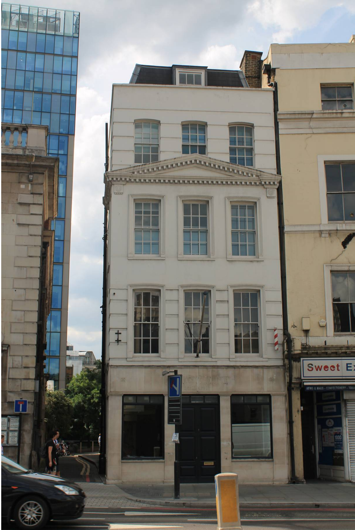
Plate 4 Facade of No. 117, looking west
