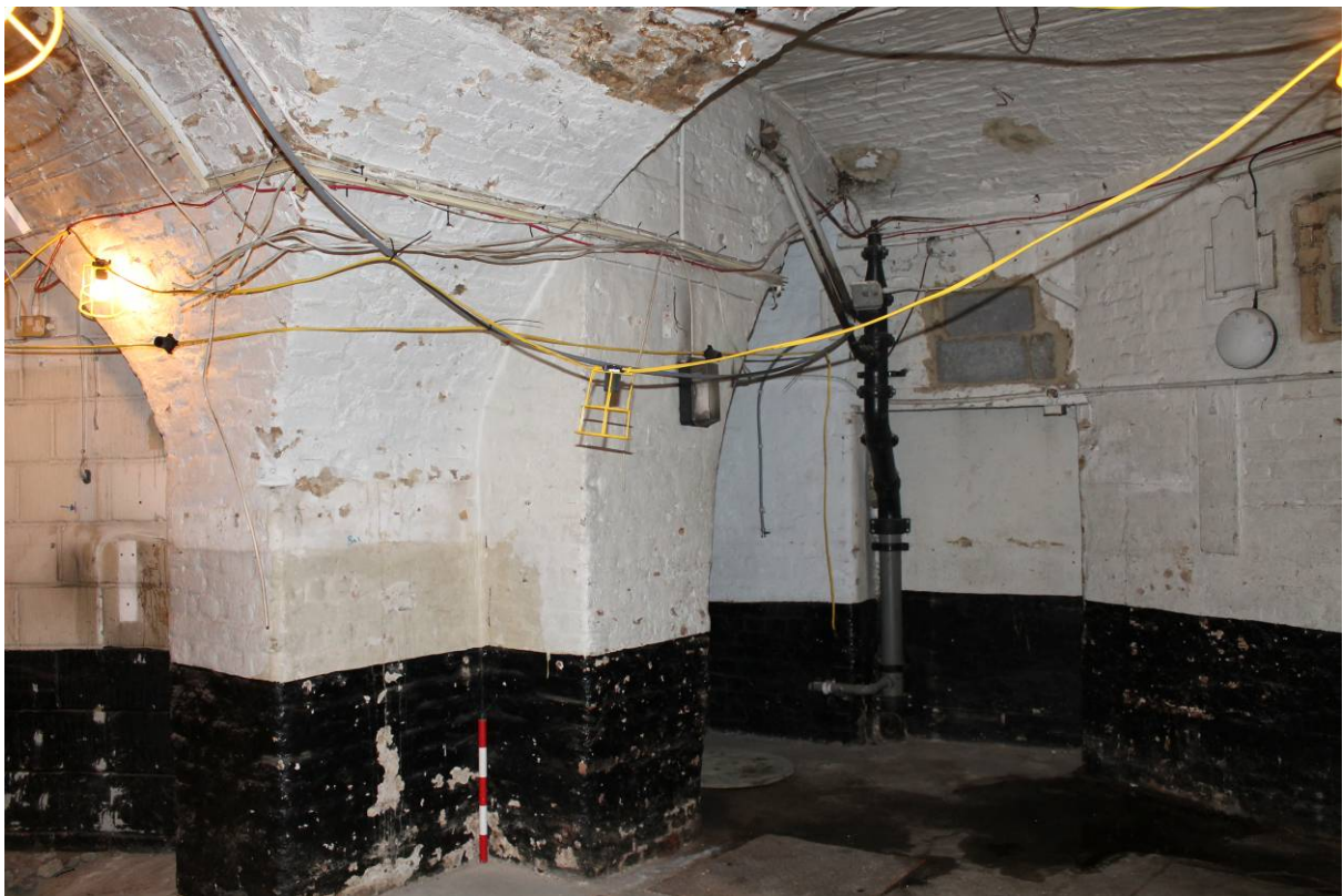
Plate 20 Basement (3) looking north-west towards vaulted area (4)
