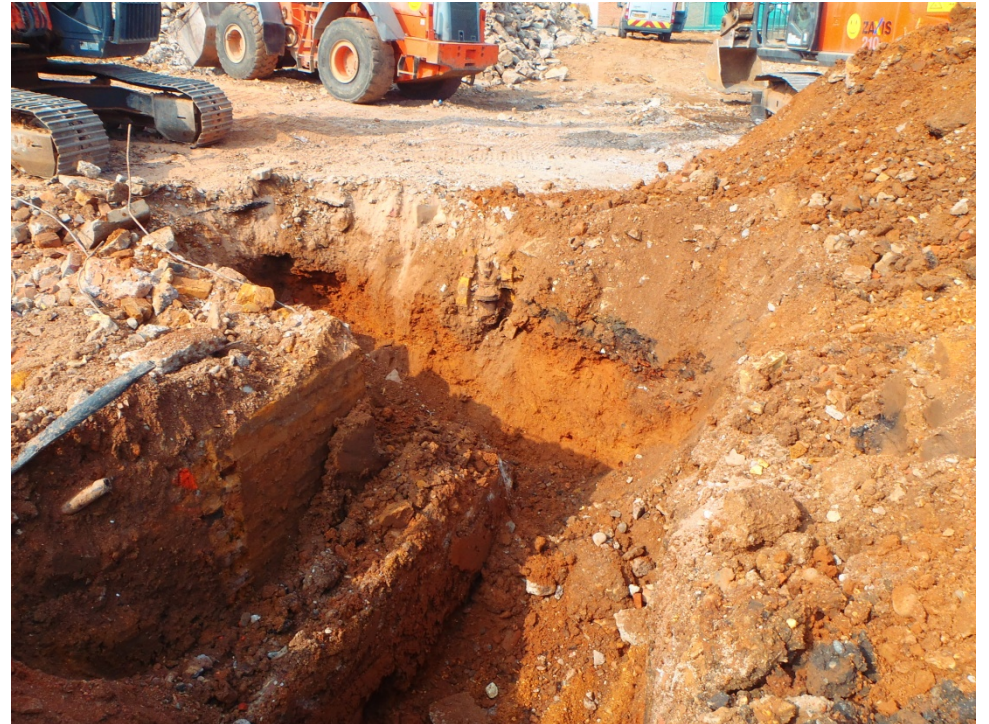
PLATE 2: SOUTH FACING SHOT OF SECTION 6
