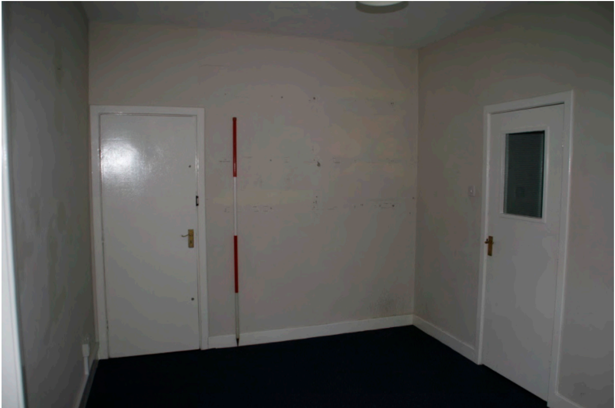
Plate 48: South wall of room AHF2, looking south (TRC14 BHD100 (55))
