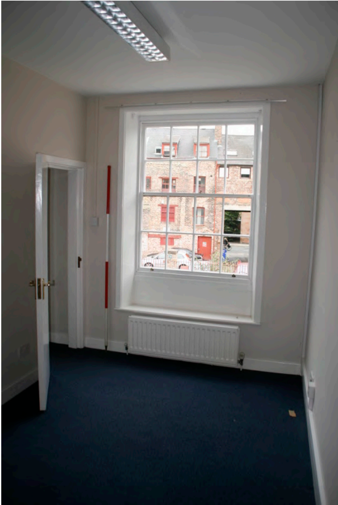
Plate 46: East wall of room AHF4, looking east (TRC14 BHD100 (51))
