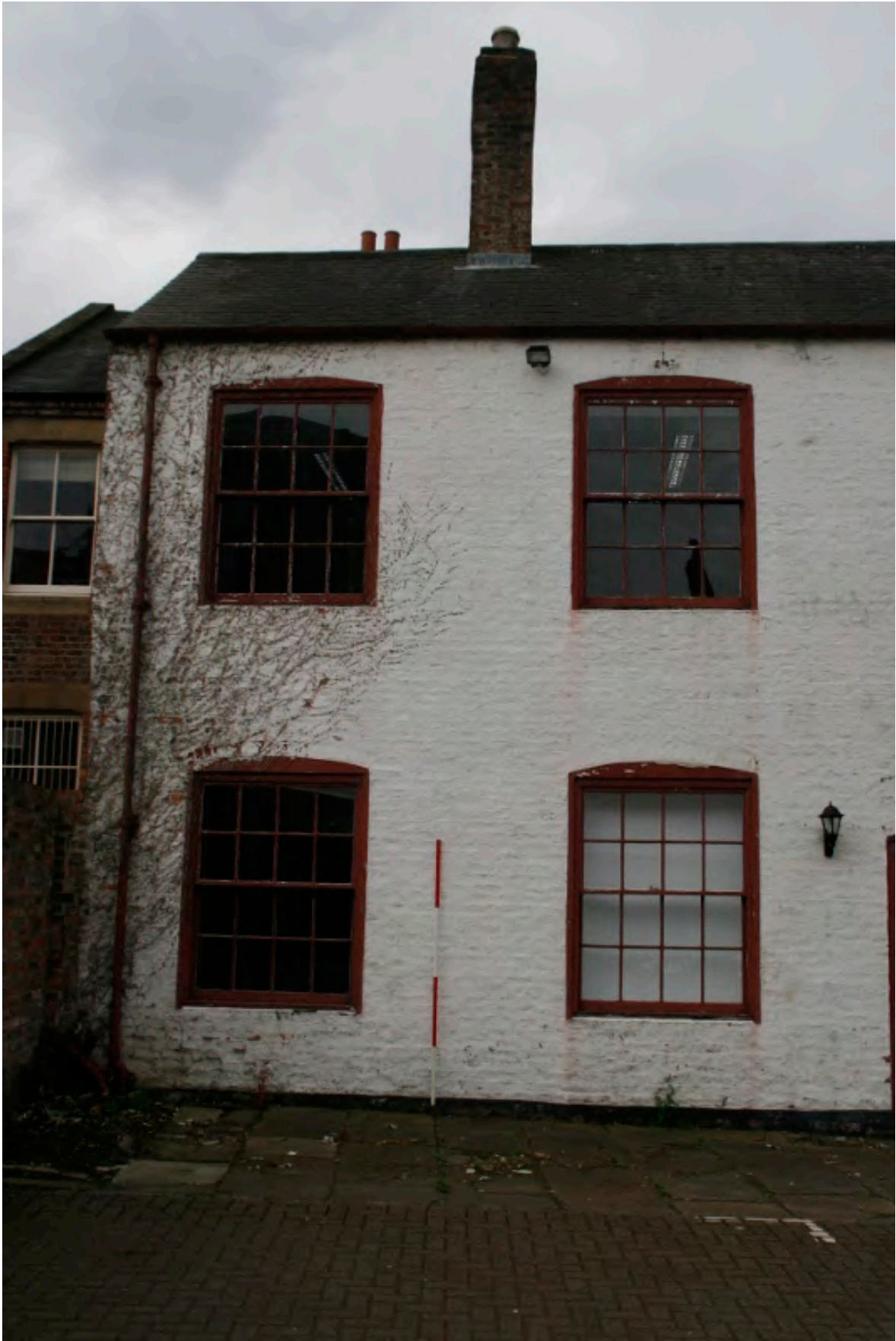
Plate 14: South end of the front (east) elevation of the almshouses, looking west (TRC14 BHD100 (17))
