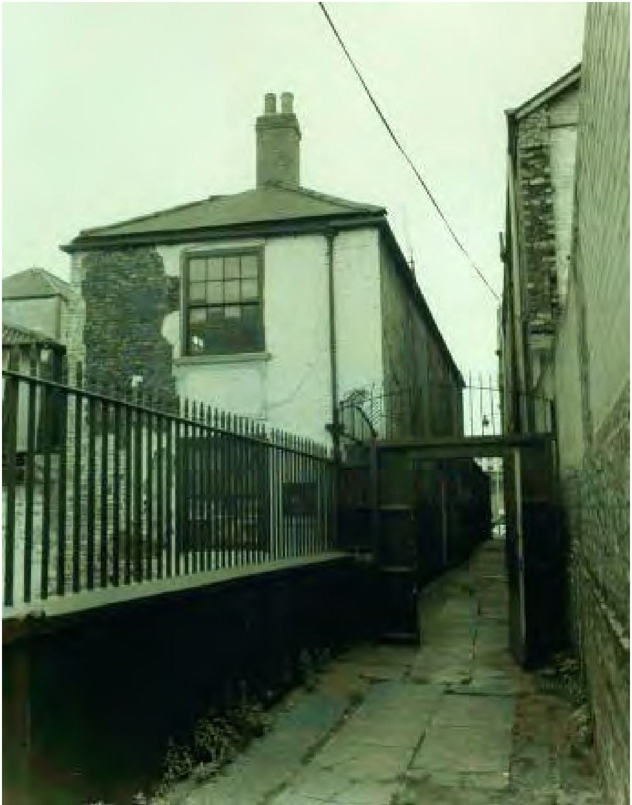
Plate 1a: Photograph taken in the 1970s showing the north elevation of Nos 9 and 10 Trinity Chare, looking south (© Tyne and Wear Archives).
