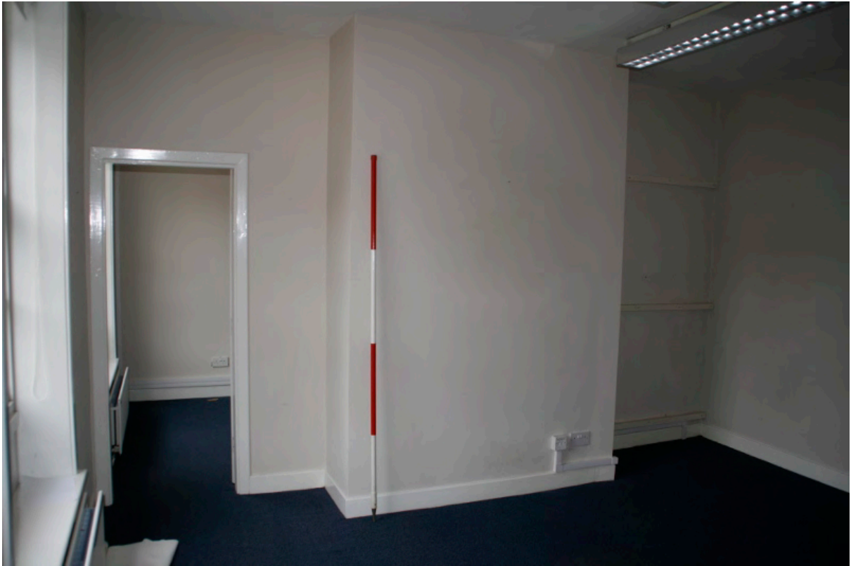
Plate 45: South wall of room AHF3, looking south (TRC14 BHD100 (52))
