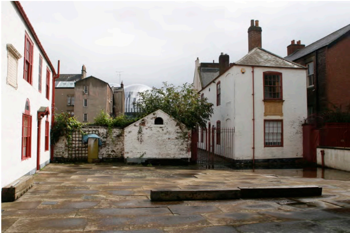
Plate 8: North elevations of the sandstone wall, outdoor toilet and almshouses, looking south (TRC14 BHD100 (76))
