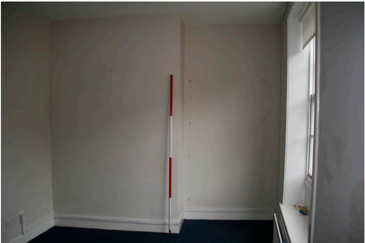
Plate 49: North wall of room AHF2, looking north (TRC14 BHD100 (56))
