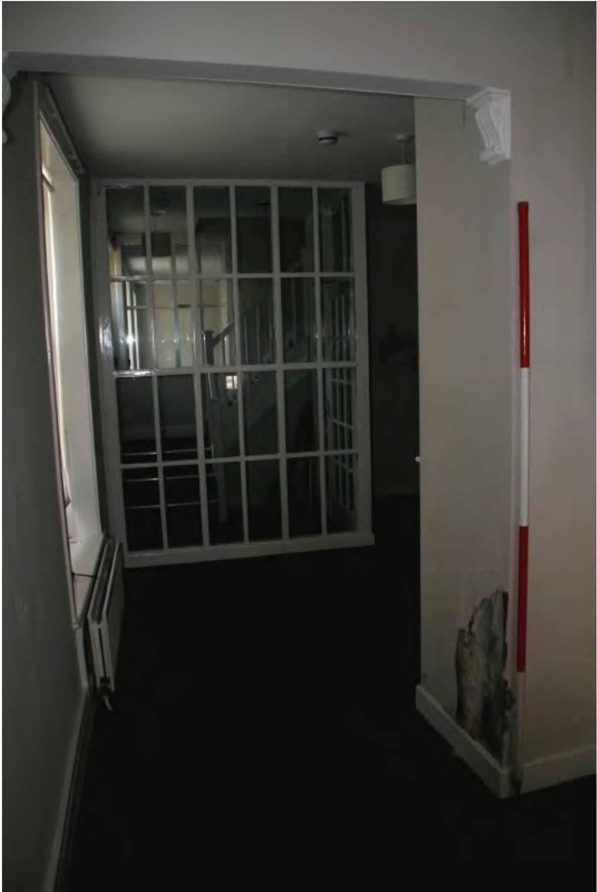
Plate 31: Room AHG2, looking south (TRC14 BHD100 (37))
