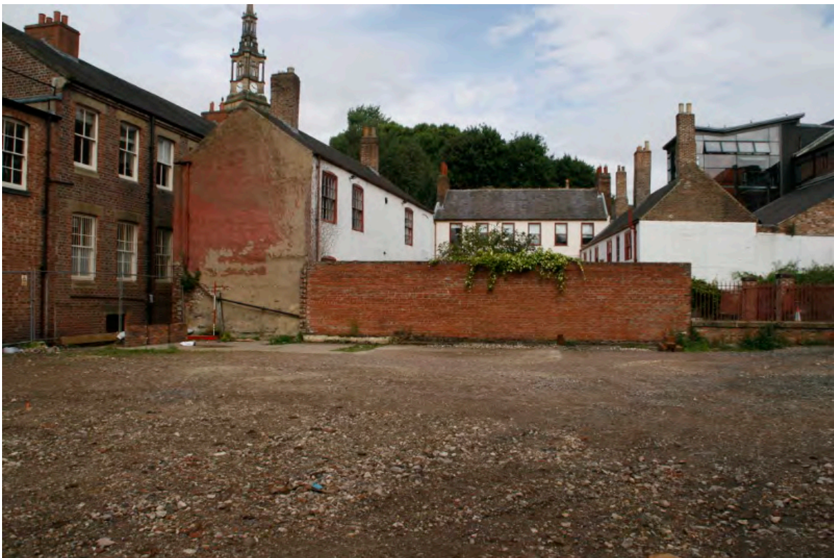
Plate 19: Side (south) elevation of the almshouses, looking north (TRC14 BHD100 (22))
