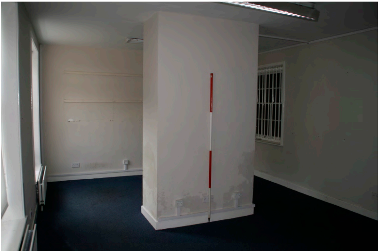
Plate 37: Original chimney breast/stack in room AHG3, looking south (TRC14 BHD100 (27))
