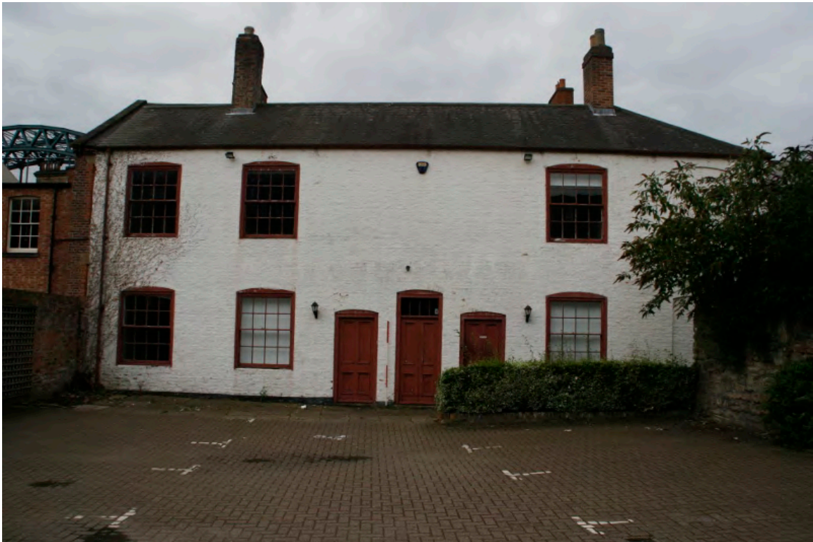
Plate 12: Front (east) elevation of the almshouses, looking west (TRC14 BHD100 (14))
