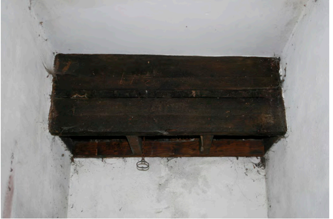
Plate 11: Wooden housing for toilet cistern (TRC14 BHD100 (11))
