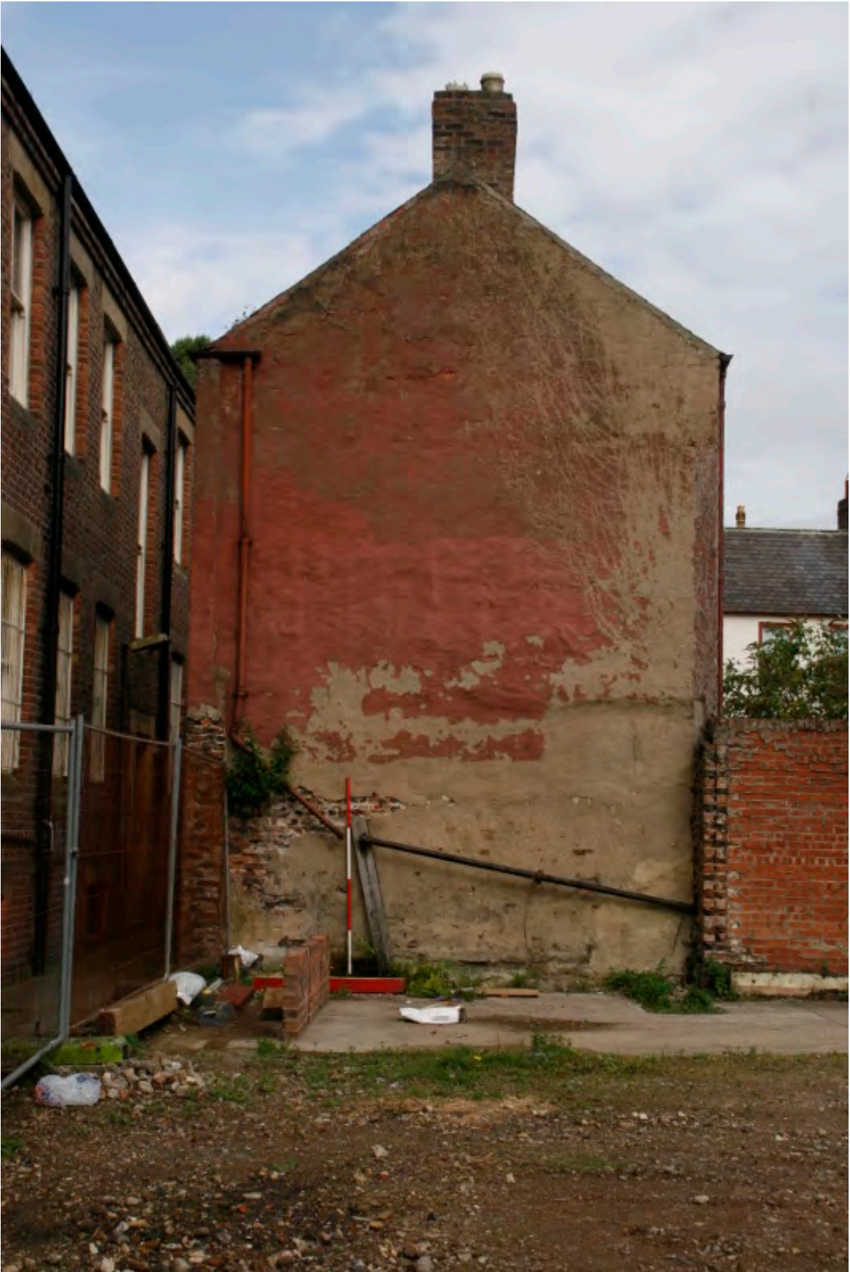
Plate 20: Side (south) elevation of the almshouses, looking north (TRC14 BHD100 (21))
