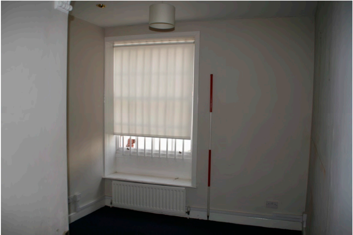
Plate 32: Sash window in east wall of room AHG1, looking north north-east (TRC14 BHD100 (36))
