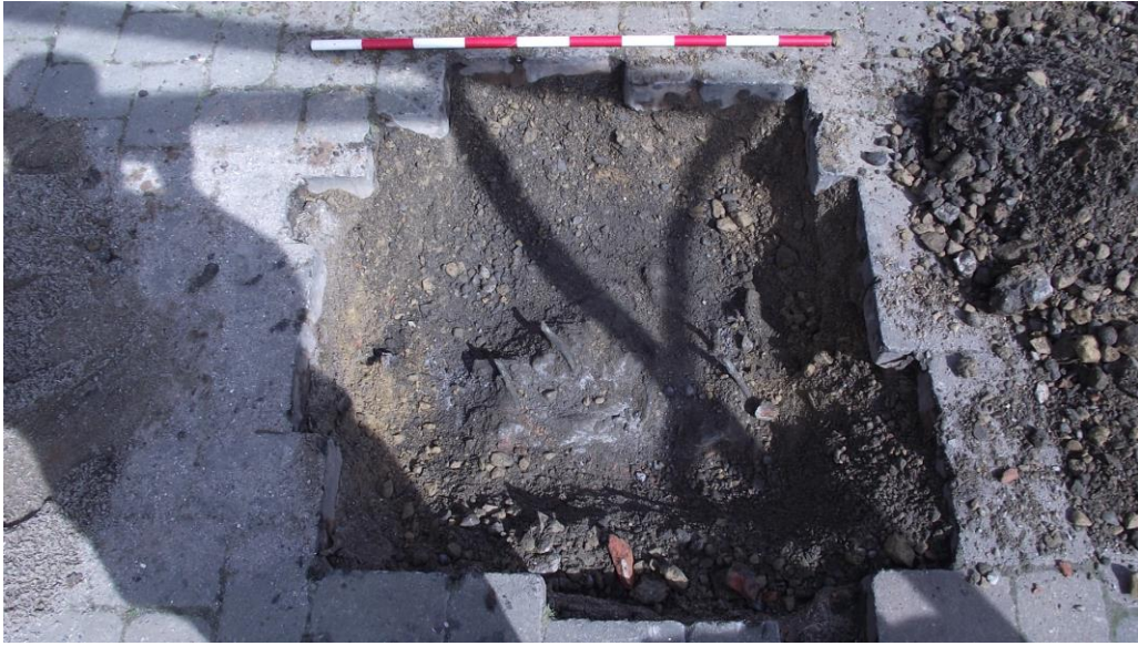
Plate 4: Test Pit 3 concrete pile capping [9], facing east (scale 1m)
