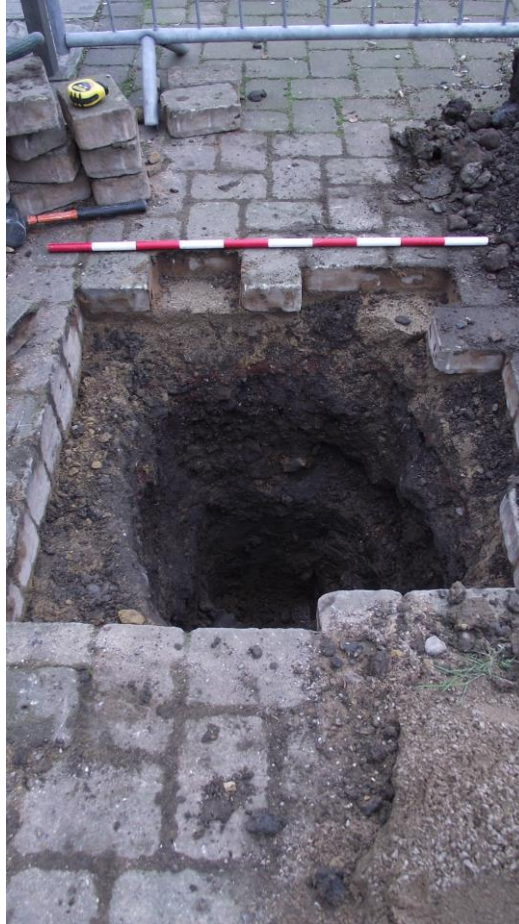
Plate 1: Test Pit 1 west facing section (scale 1m)
