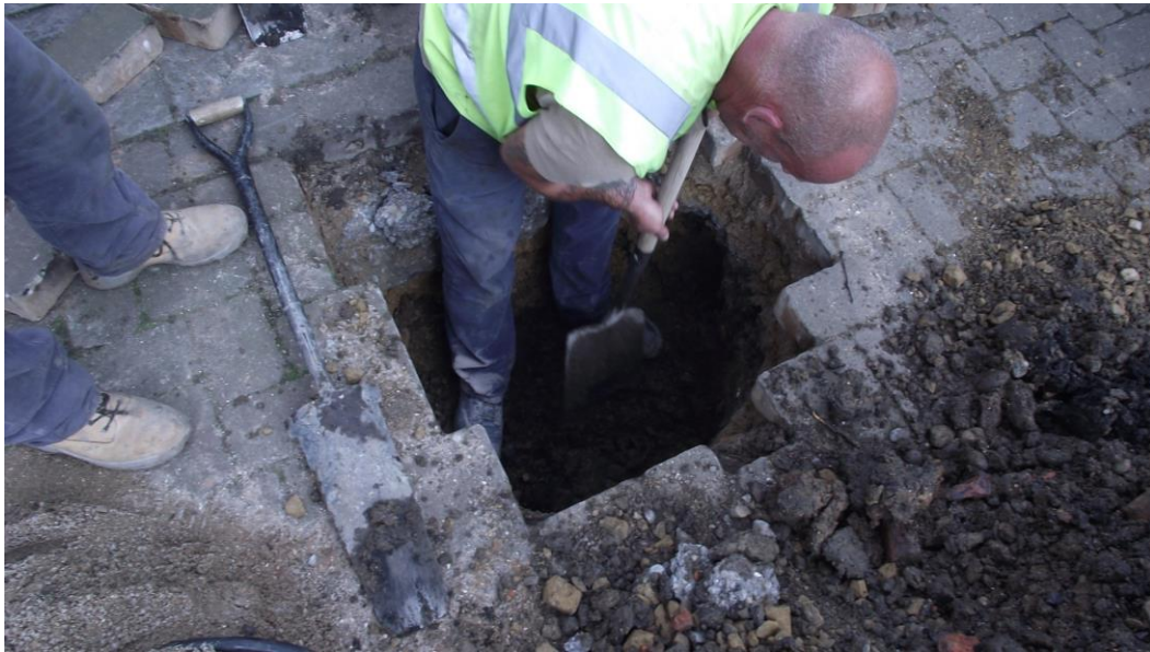
Plate 2: Test Pit 2 working shot
