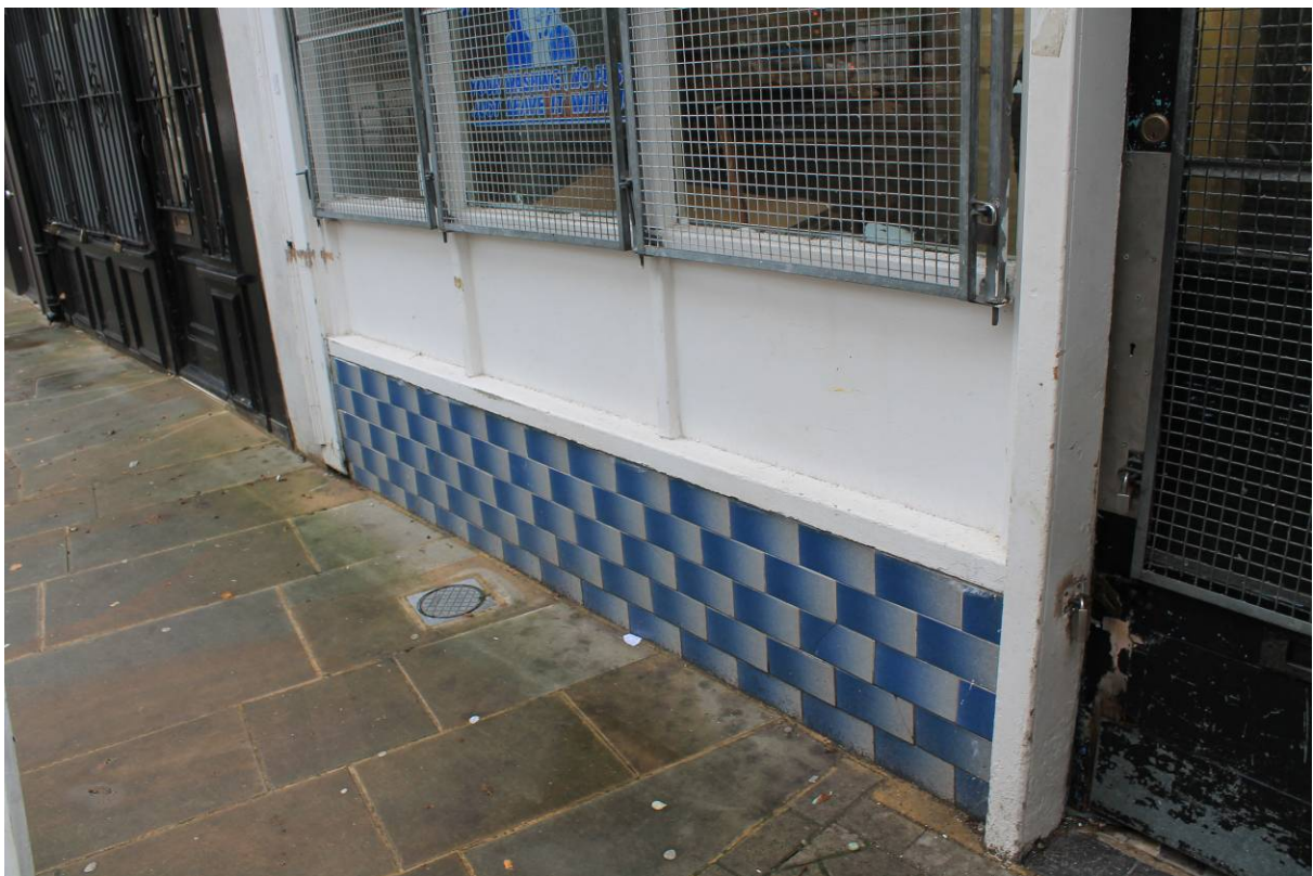
Plate 3 Detail of tiled apron and shop front, looking east
