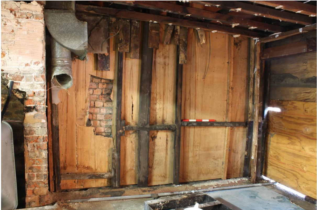
Plate 15 Modern, lightweight framing and boarding of eastern flank wall
