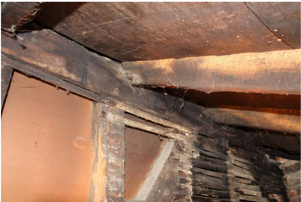
Plate 12 Detail of nailed-on batten/ledge supporting lean-to roof rafters
