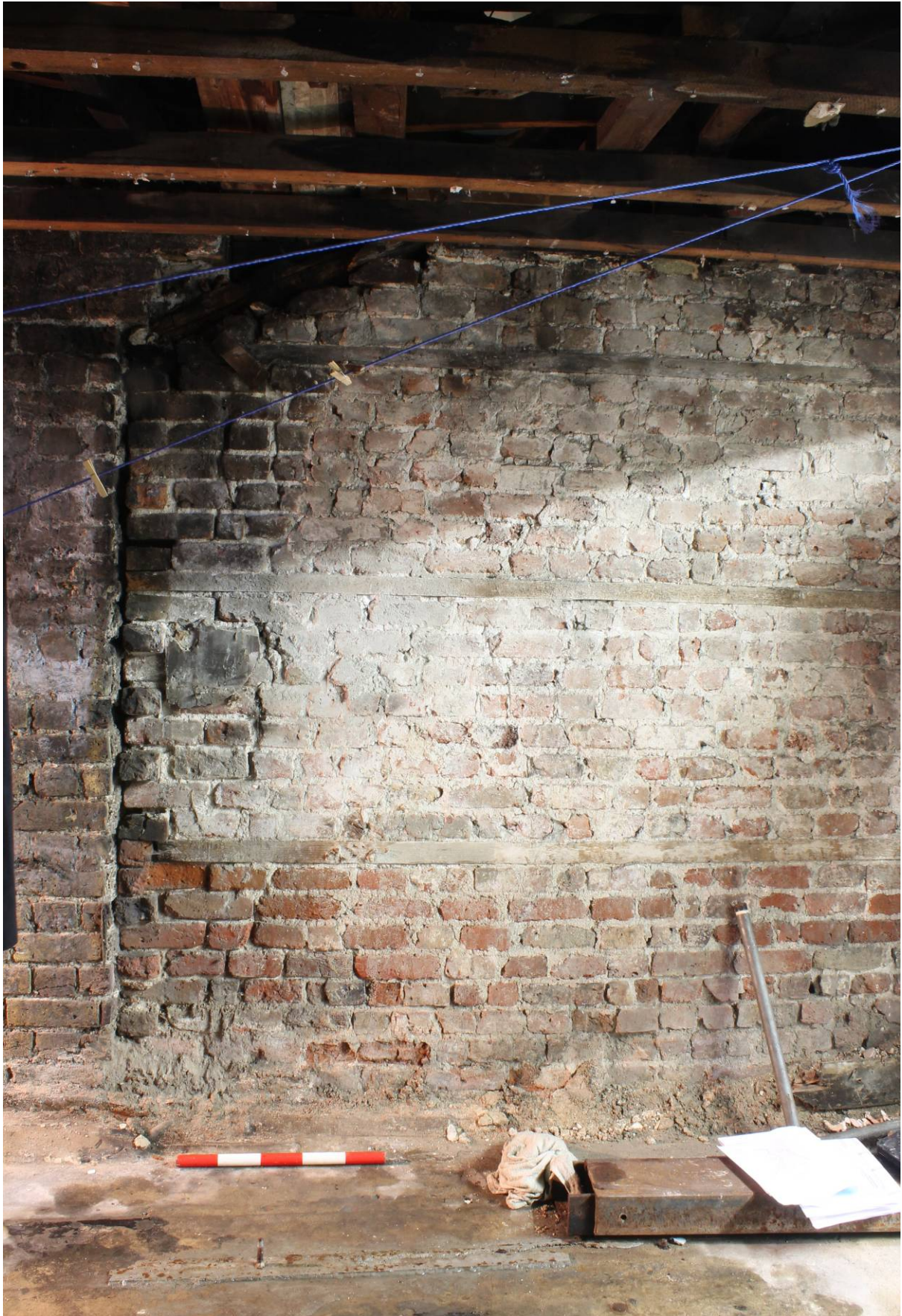
Plate 13 Brickwork A of lean-to extension showing timber bearers
