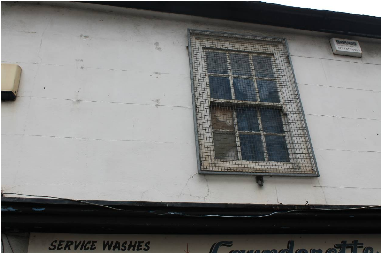
Plate 2 No. 29 facade with line out render and horned sash window at first floor level, looking south
