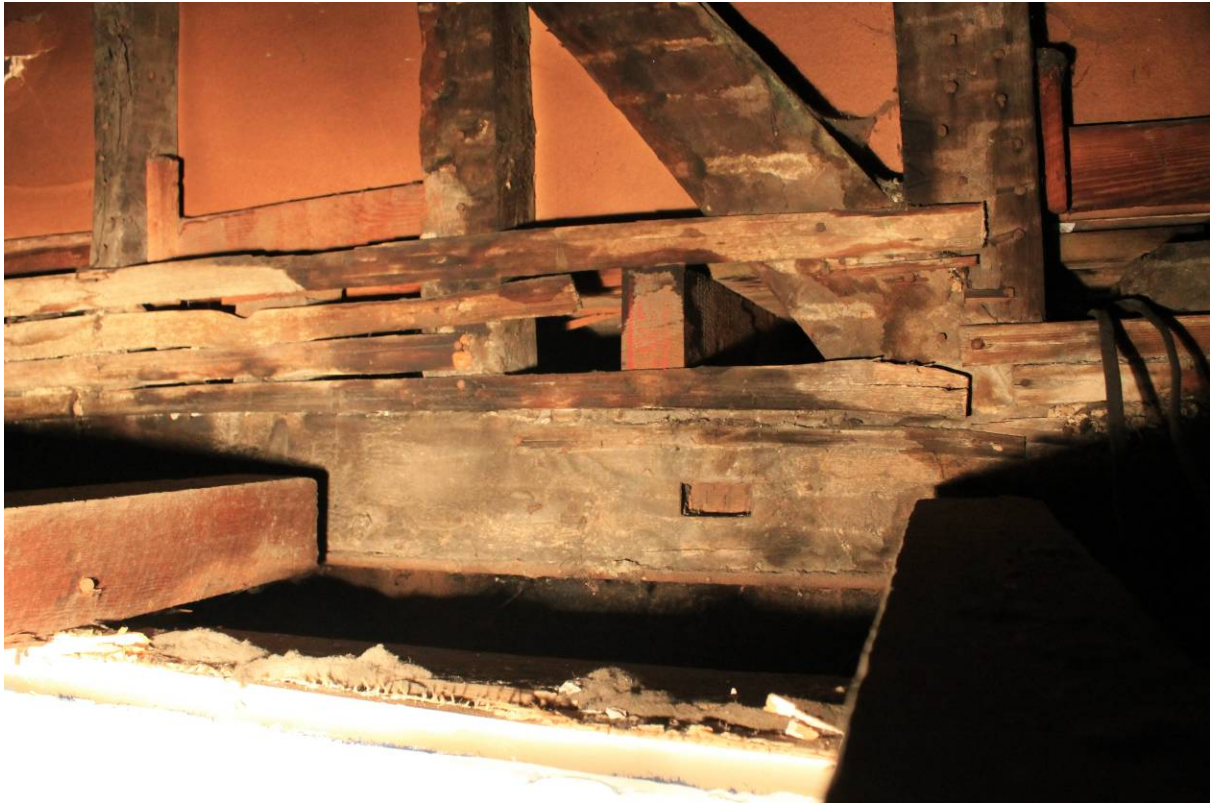
Plate 11 Detail of empty mortise in mid-rail (for ceiling joist)
