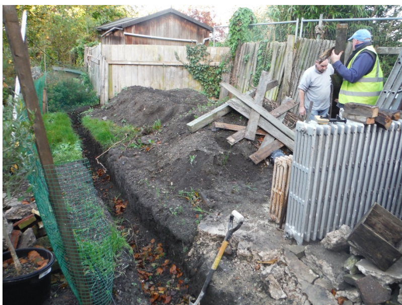
Plate 1: The site prior to excavation, view north-west
