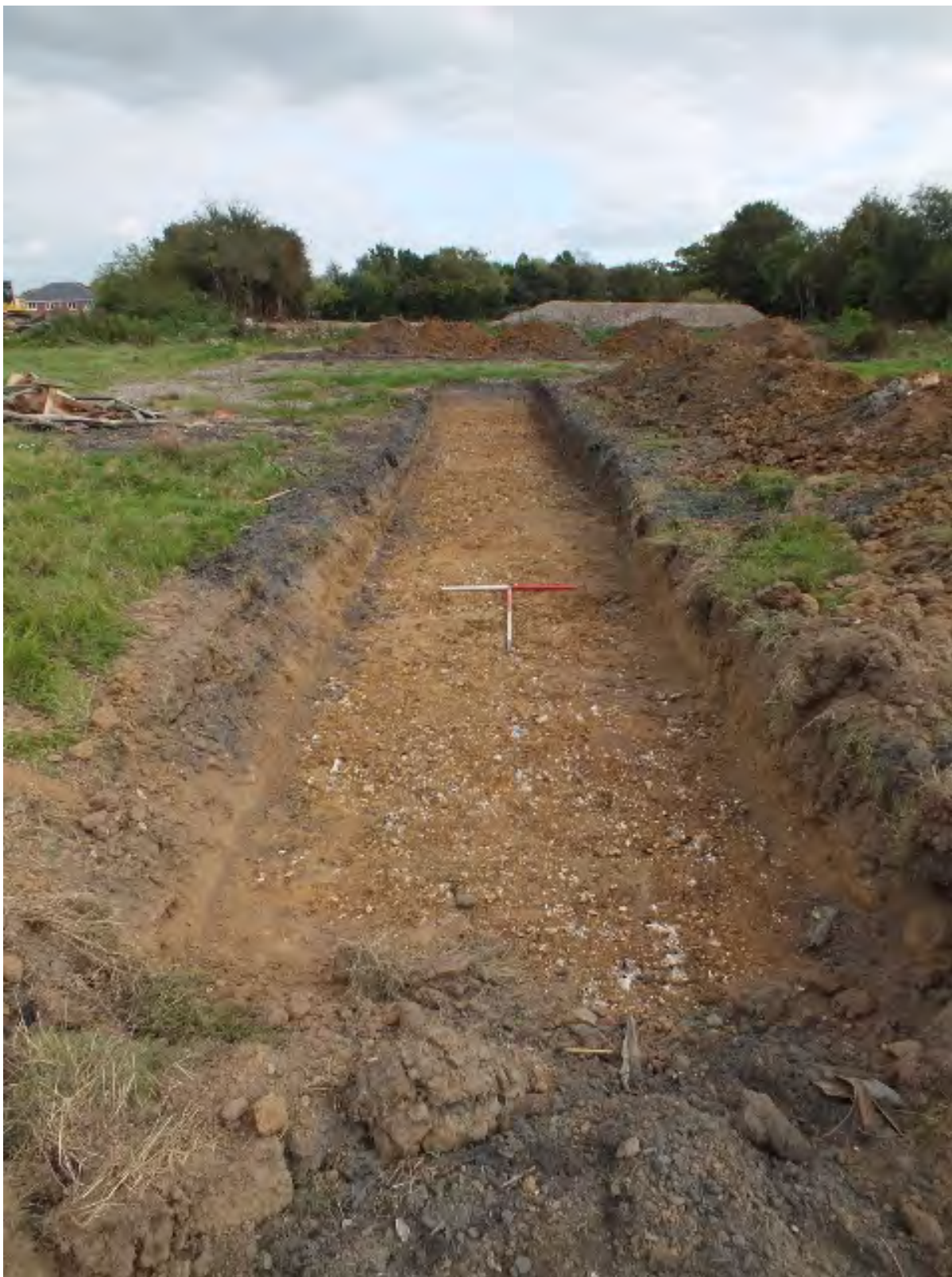
Plate 17: Overview of trench 18, looking south-east (RRHH14 D1 (1))
