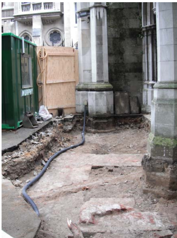
Plate 3, view west within Trench 1 showing [51], [55] and [56]
