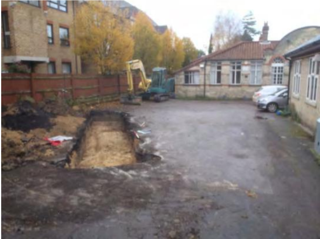
Plate 2: Trench 1, view south-west showing Trench 1 location
