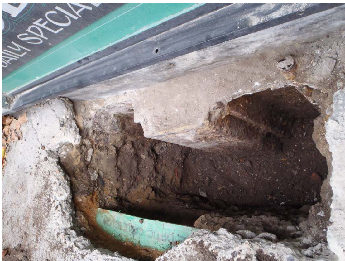
Plate 1 Northeast view of Test Pit 1; Fibre optic cable, steel sheet pile and modern backfill
