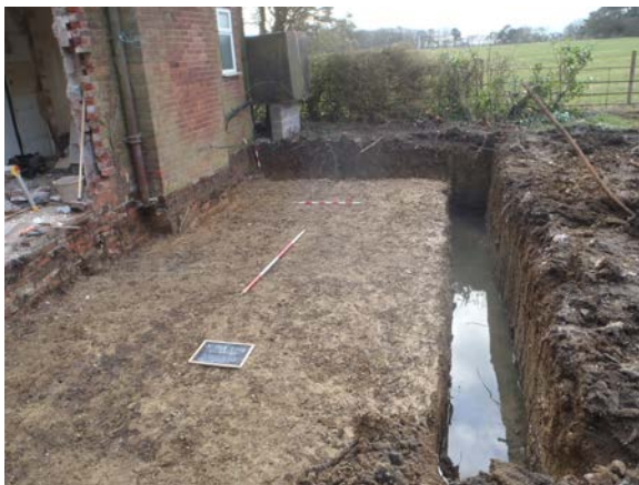
Plate 5. Rear extension foundations. View west. 2m, 1m, & 0.4m Scales
