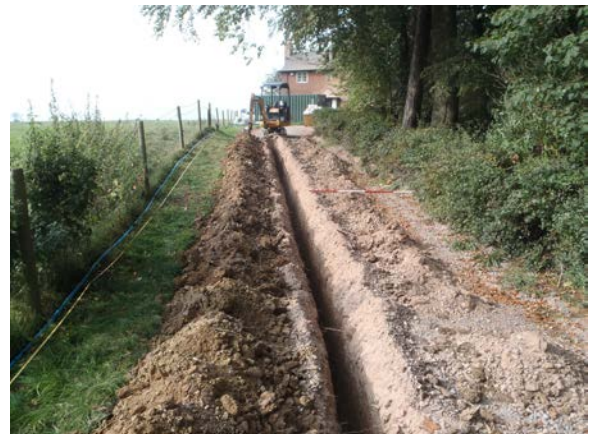
Plate 6. Water Pipe trench. View northwest. 2m scales
