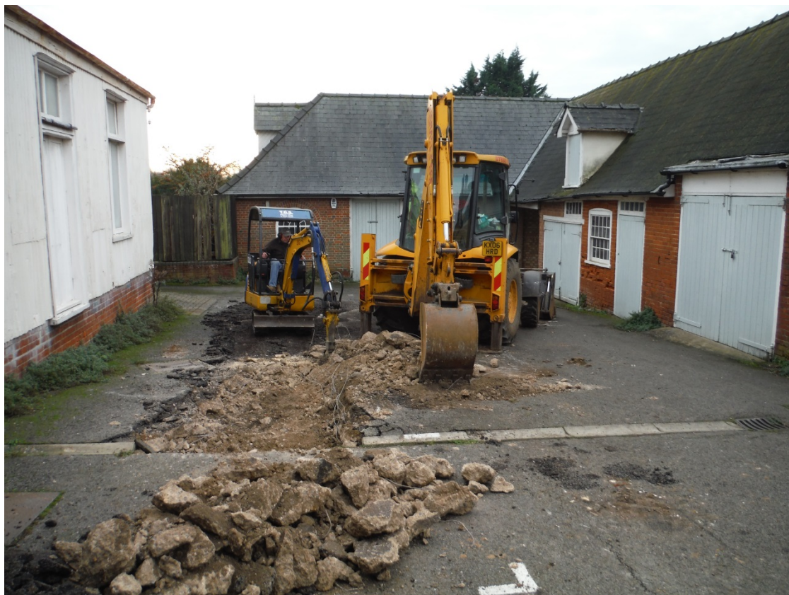
Plate 1: Trench 1 during breaking of reinforced concrete, view south
