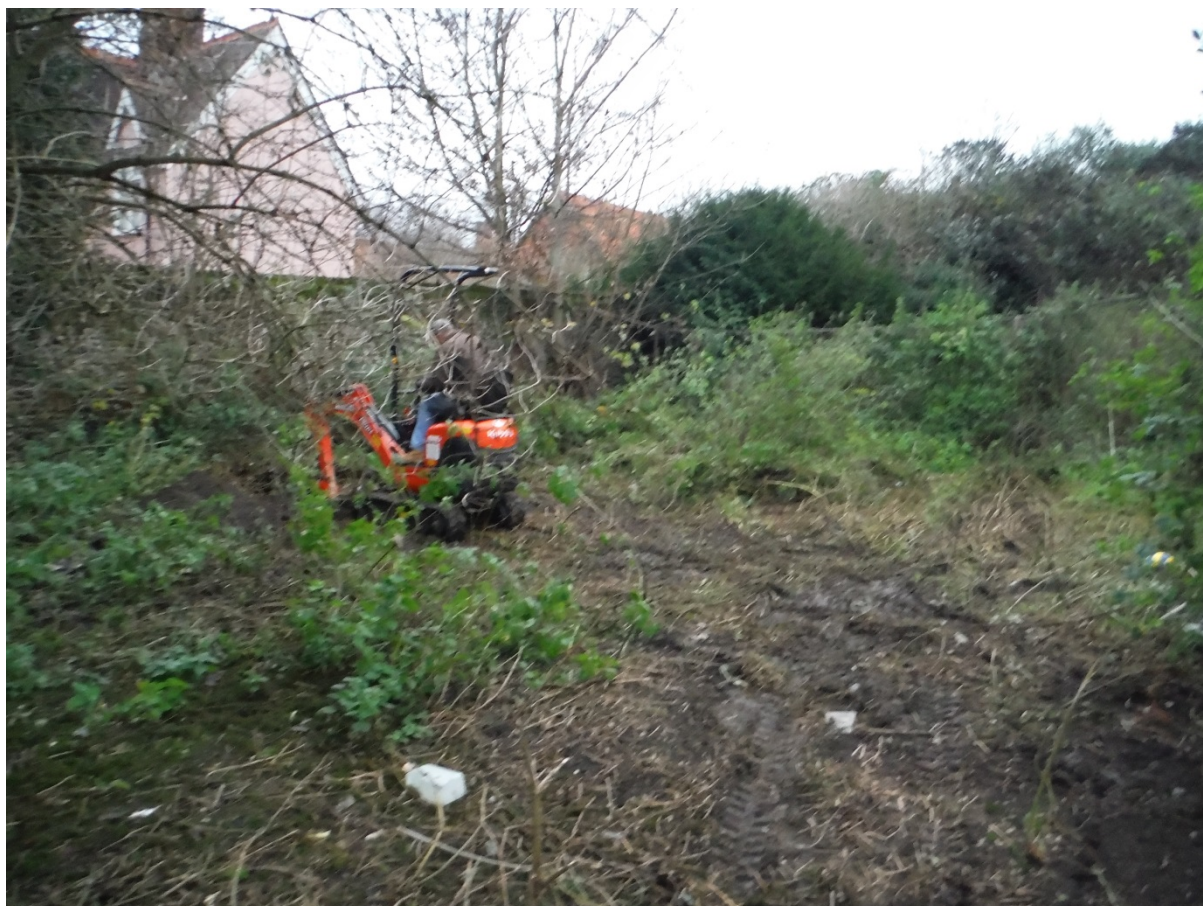
Plate 6: Machining Trench 2, in walled garden, view north-west
