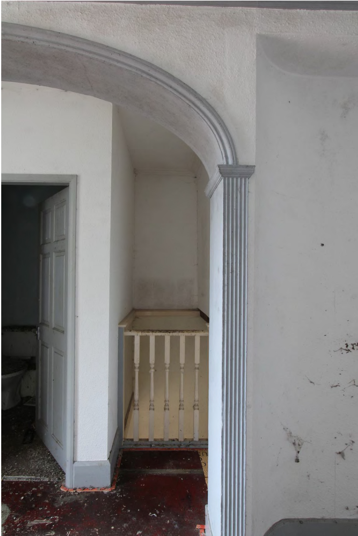
Plate 19 Detail of elliptical arch, WC (FF3) and stairwell
