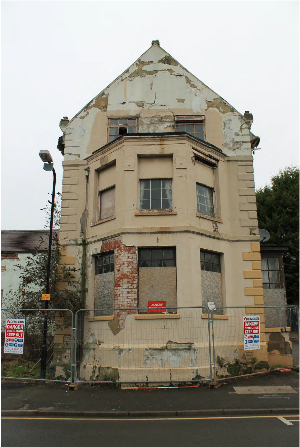
Plate 6 Southern elevation, looking north
