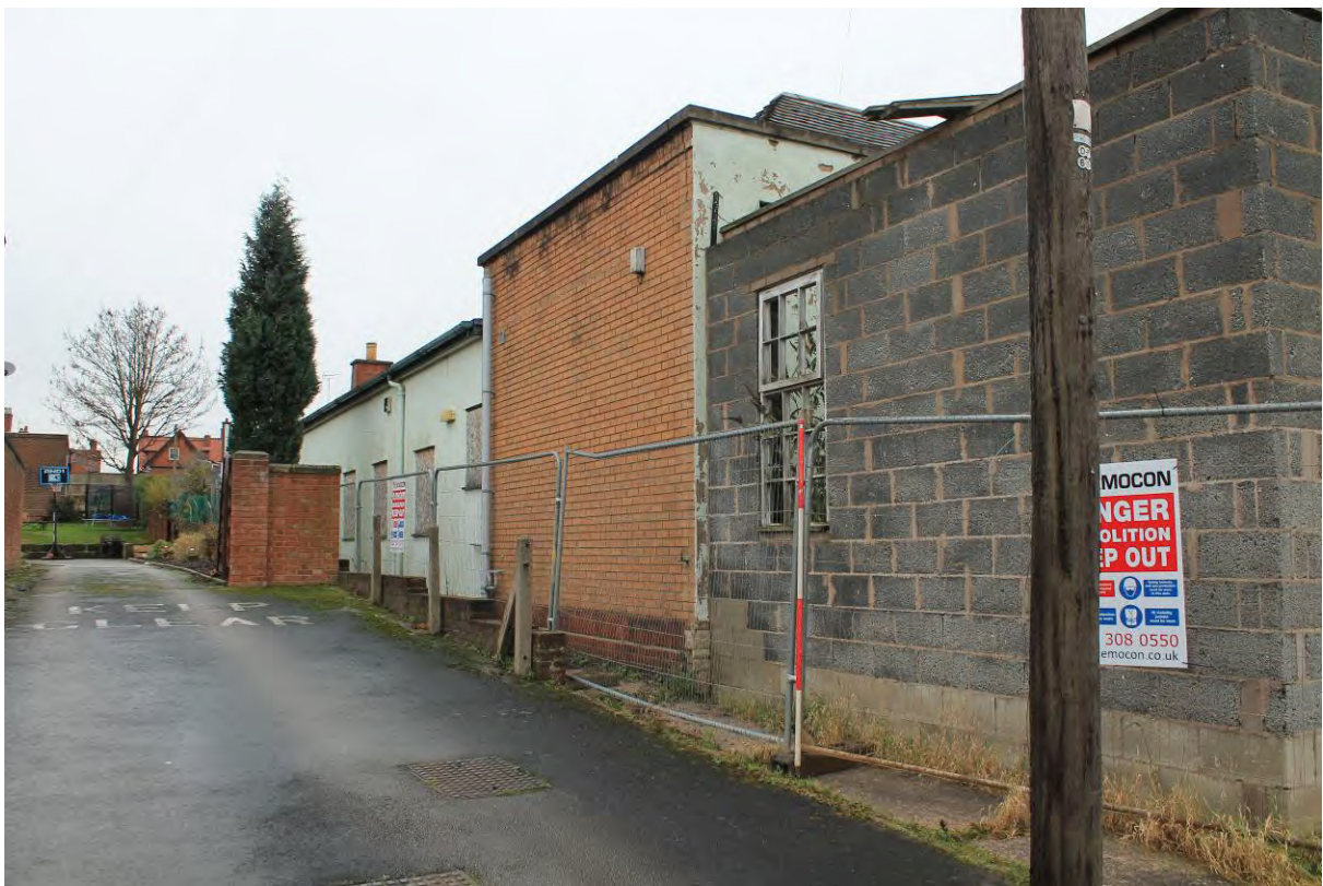
Plate 29 Western elevations of Care Home, looking north
