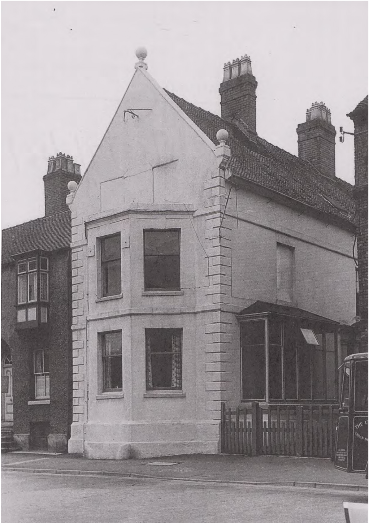
Historic Plate 1 Balance House, looking north-west (note blocked attic and first floor windows)
