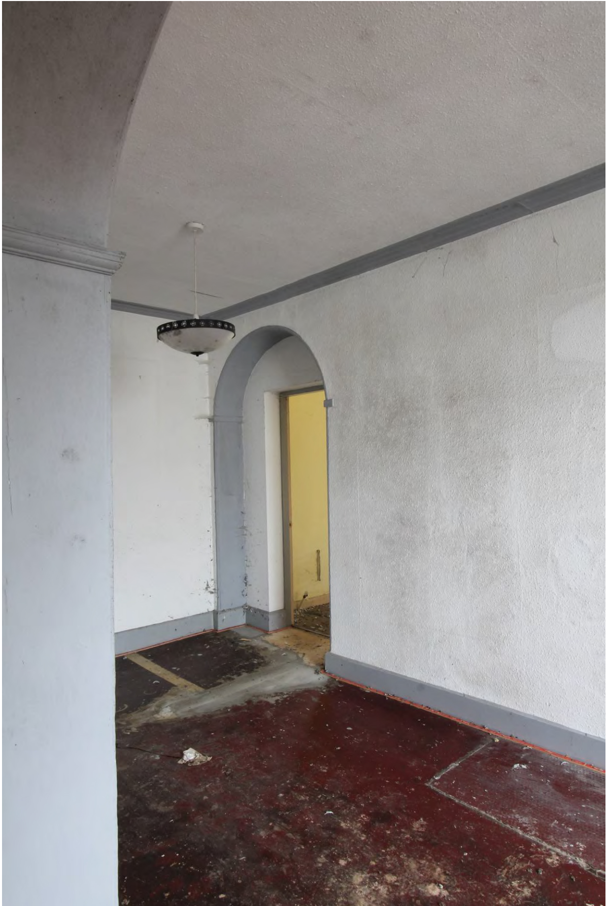
Plate 18 First floor landing (FF4) looking north-west
