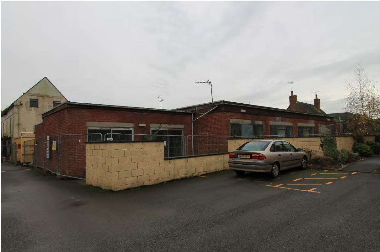
Plate 30 Northern elevations of the Care Home, looking south
