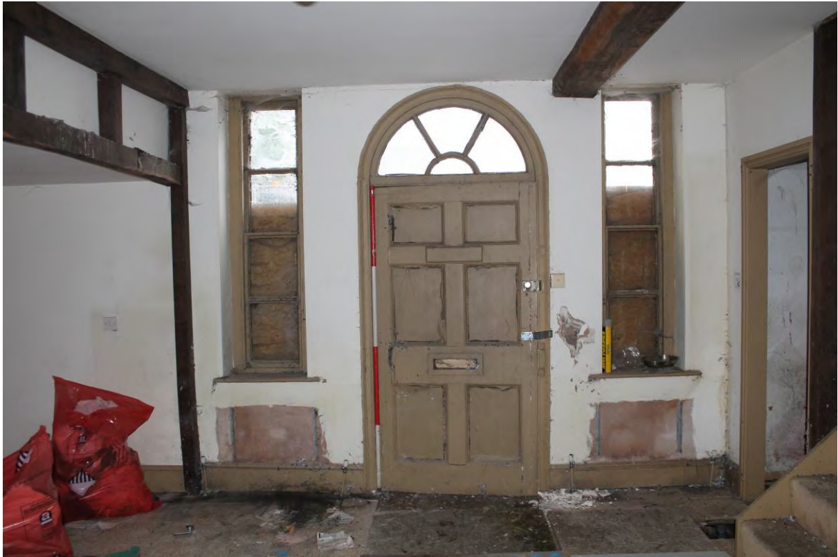
Plate 12 Detail of Principal Door and side lights, looking east
