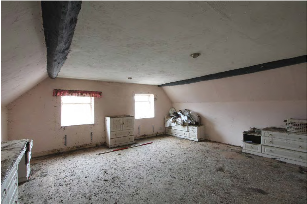
Plate 26 Bedroom (SF4) looking north
