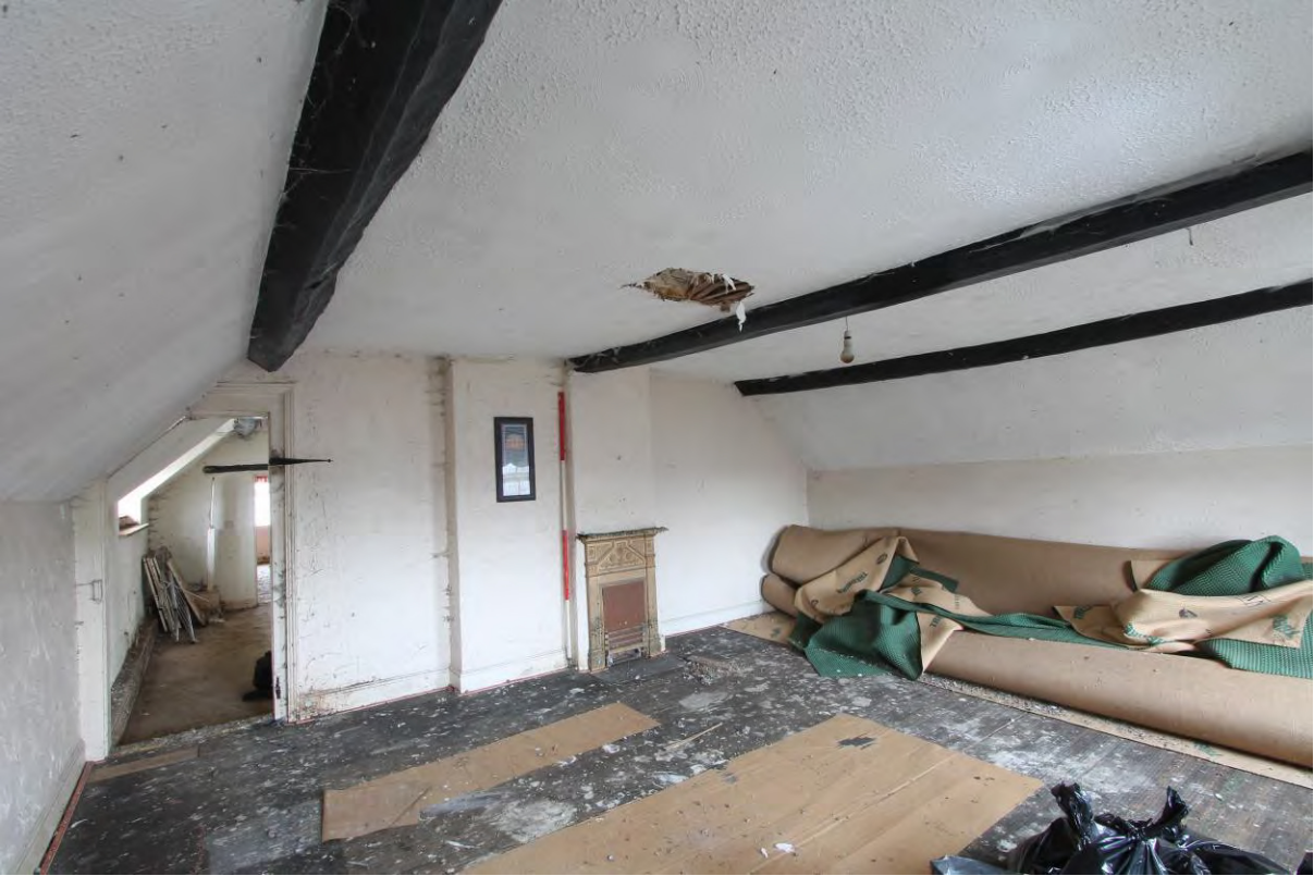
Plate 22 Bedroom (SF1) looking north
