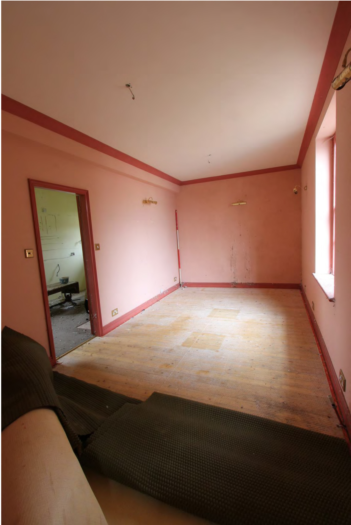
Plate 21 Bedroom (FF6) looking north
