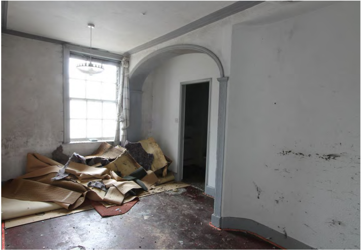
Plate 17 First floor landing (FF4) looking south-east
