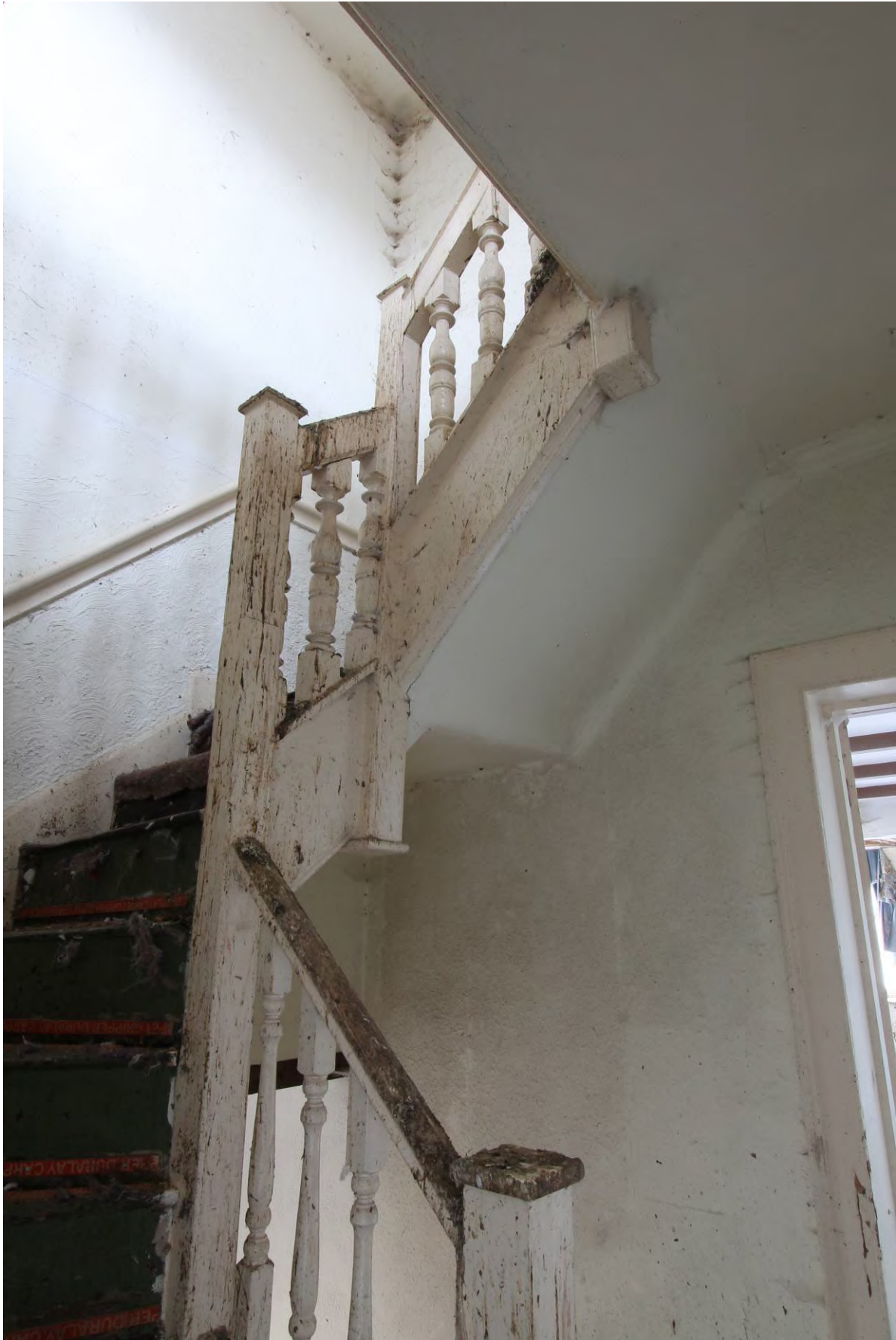
Plate 16 Newel stair to attic storey, looking south-east
