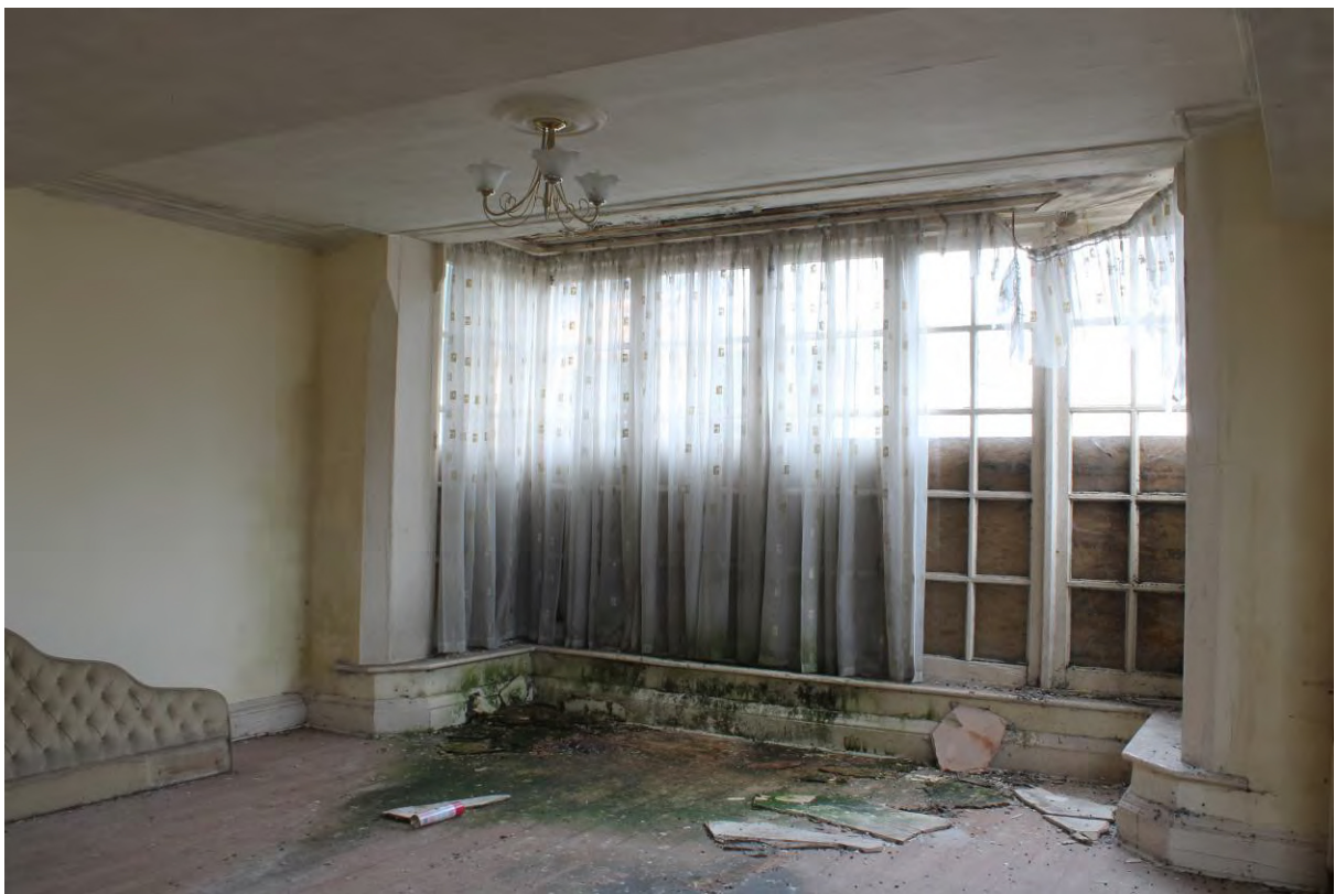
Plate 9 Ground floor front room (GF1), looking east
