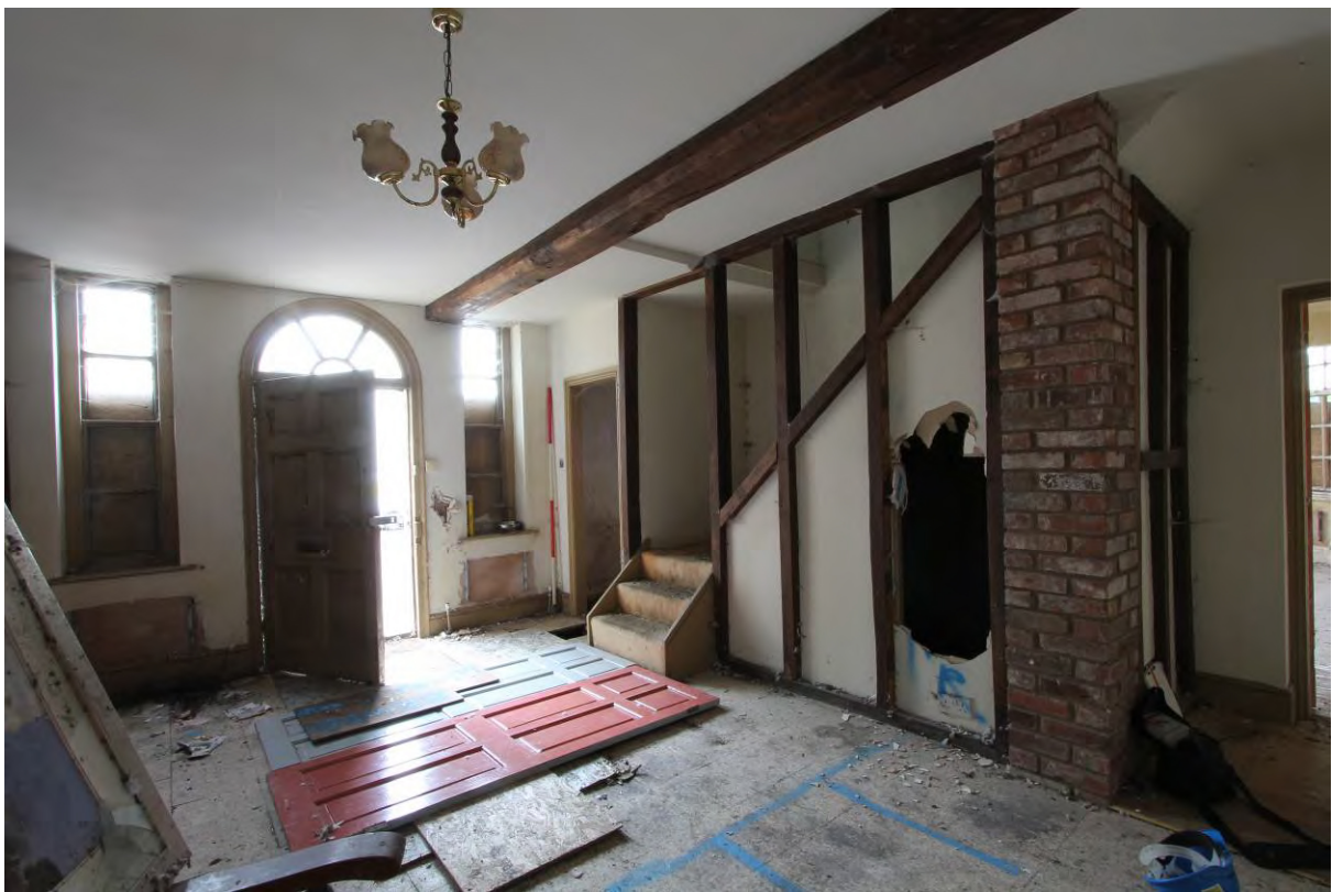
Plate 11 Entrance hall (GF2) showing boxed in stair, looking south-east
