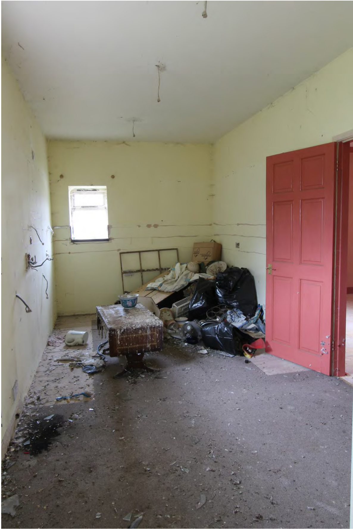
Plate 20 Bedroom (FF5) looking north
