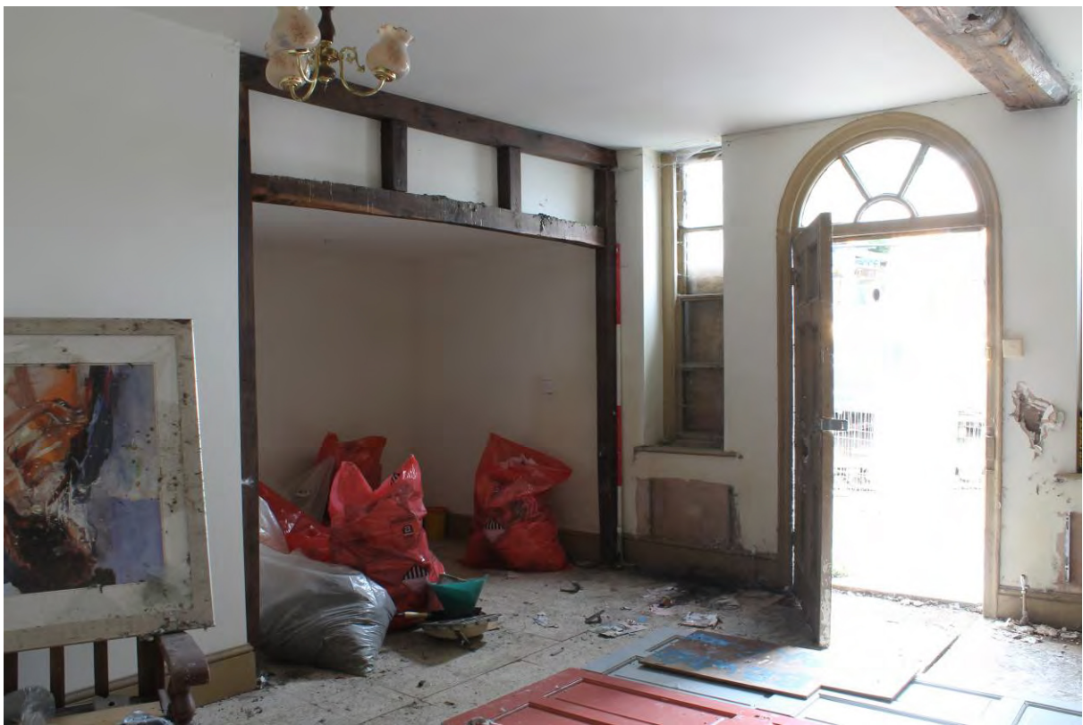
Plate 13 Entrance Hall, showing removed north wall, looking north-east
