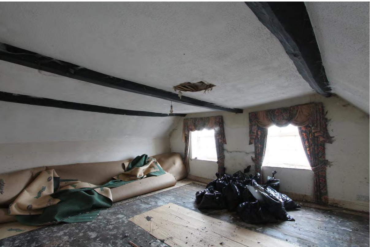
Plate 23 Bedroom (SF1) looking south-east
