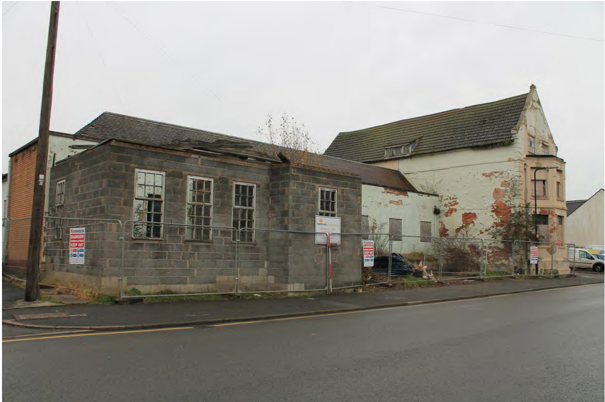
Plate 1 Modern Care Home buildings and Balance House, looking north-east
