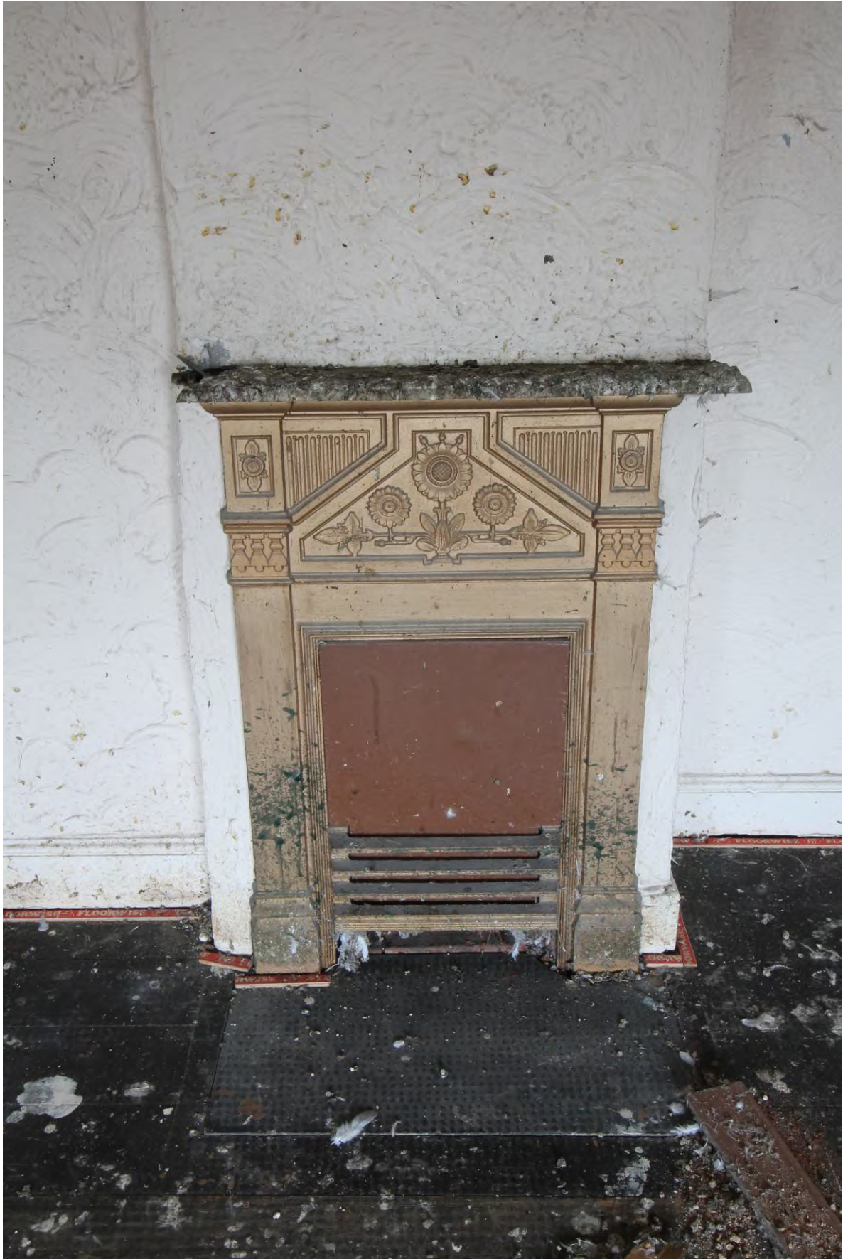
Plate 24 Cast-iron fireplace in SF1 looking north
