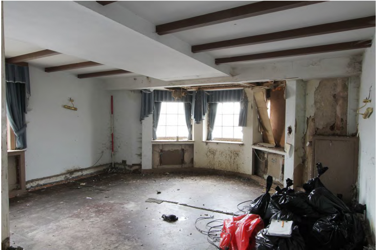
Plate 15 First floor room (FF1) looking south
