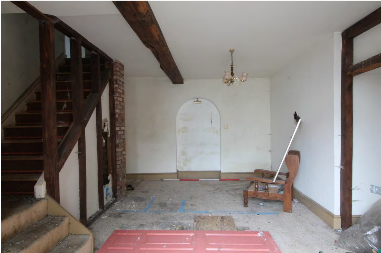
Plate 10 Entrance hall (GF2), looking west
