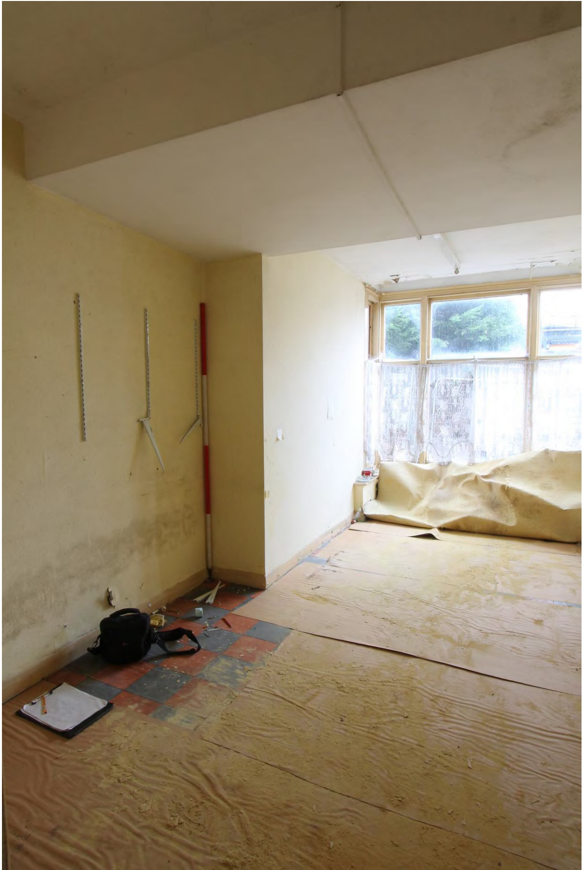
Plate 14 Room (GF3) looking east
