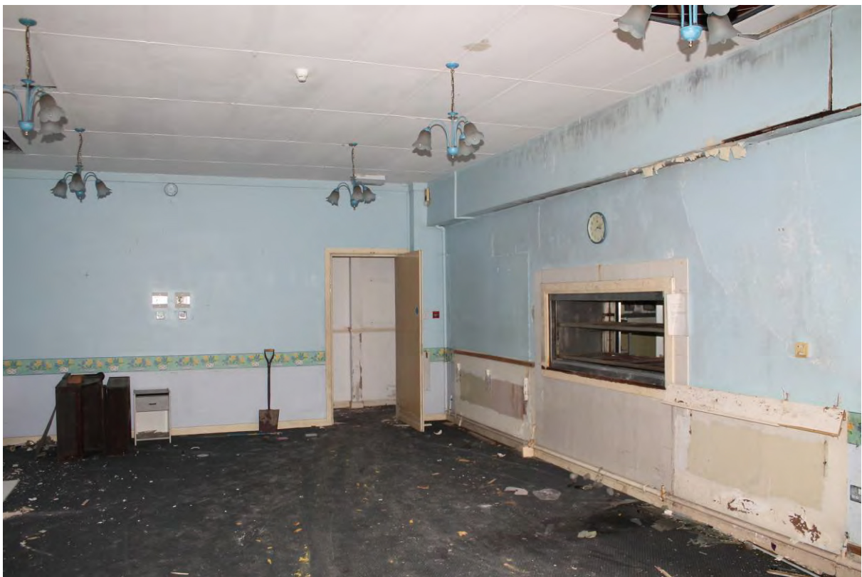
Plate 31 Dining Room in the Care Home
