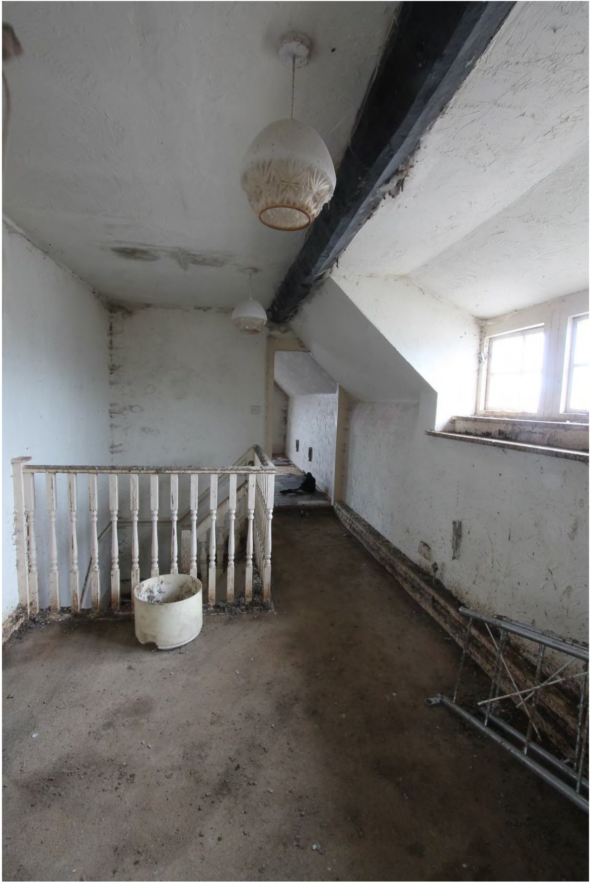
Plate 25 Second floor landing (SF2) looking south to stairwell
