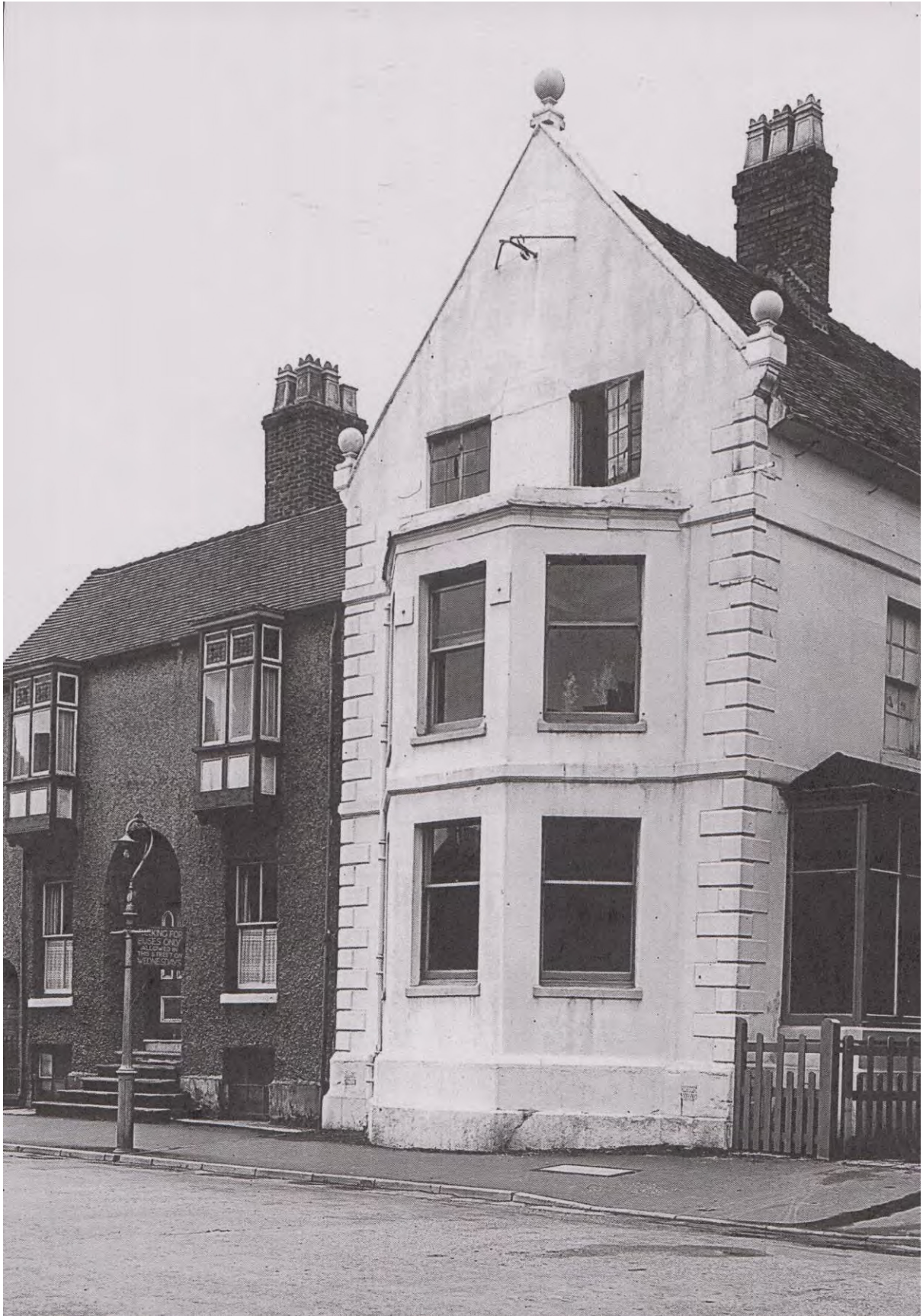
Historic Plate 2 Balance House and No. 18 Balance Street, looking north-west
