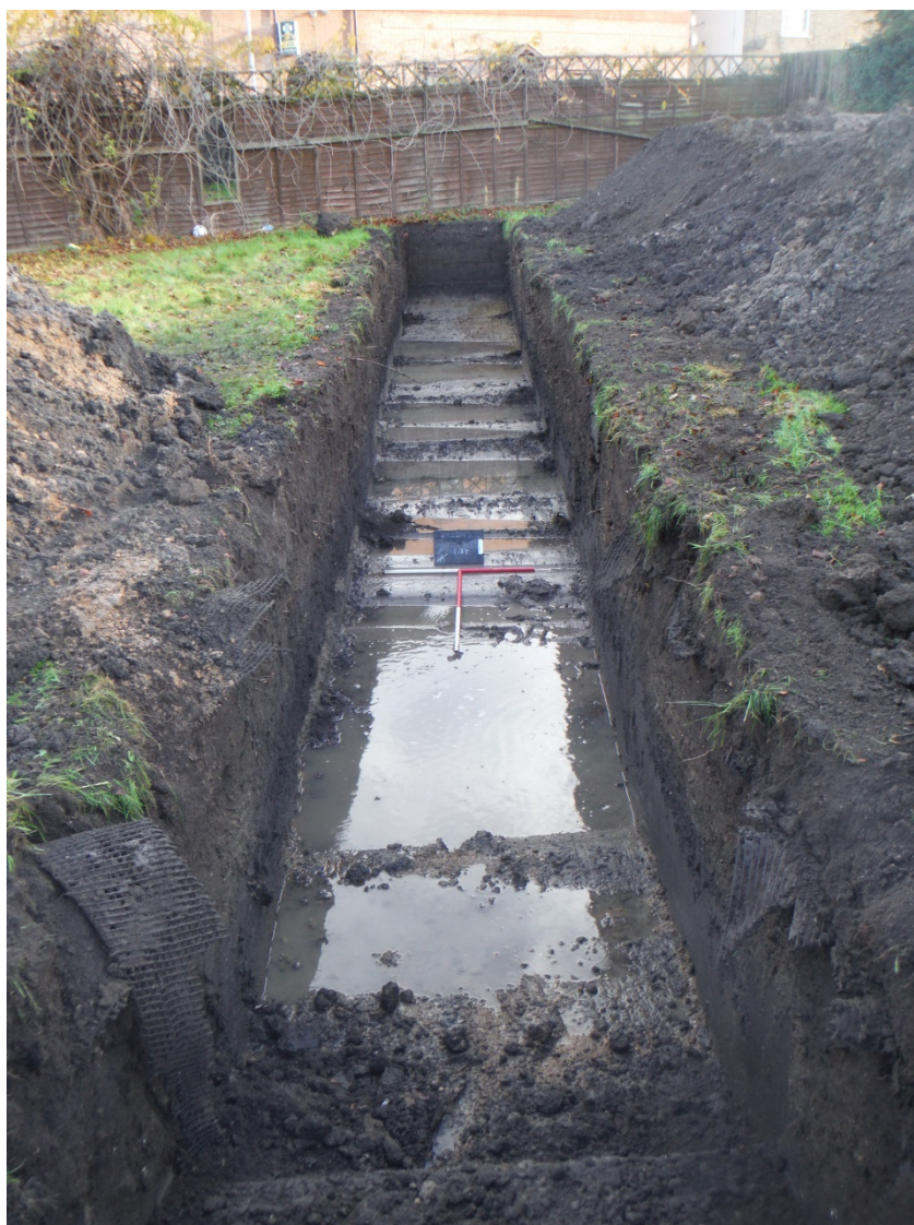
Plate 1: Trench 1, view north-east
