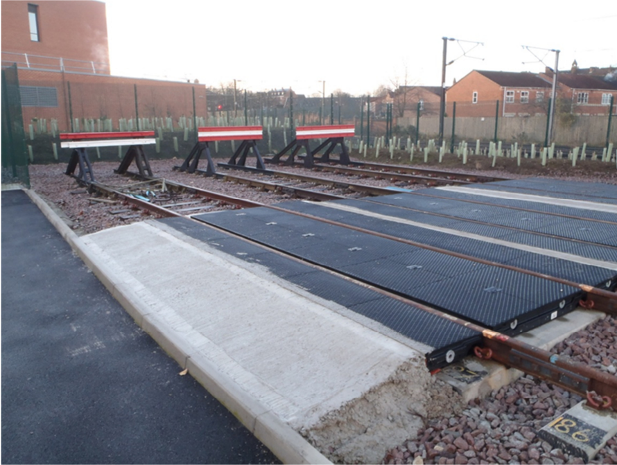
Plate 1: General site location before excavation of Trench 1, looking south
