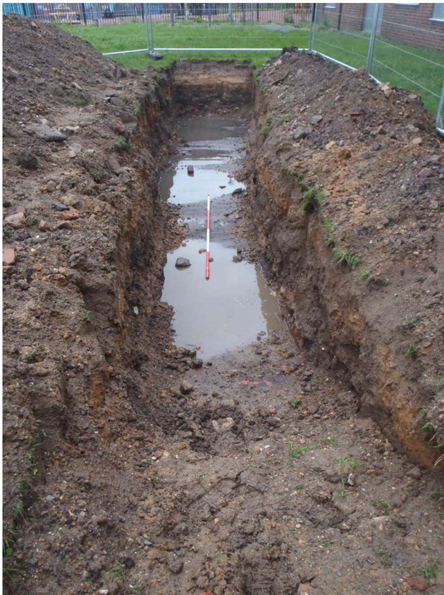
Plate 8: Trench 5 looking west
