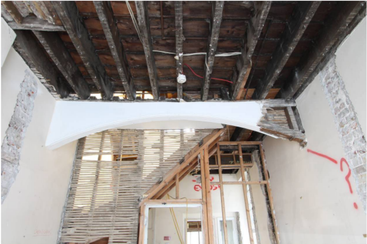
Plate 14 Detail of arch in room FF1 after soft strip, looking east
