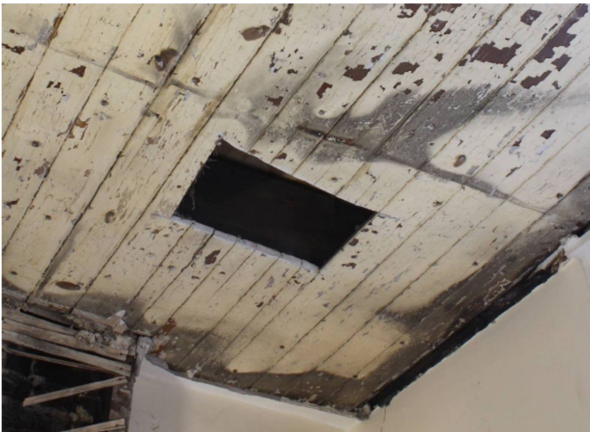
Plate 26 Timber boarded ceiling over room SF3, looking north-east
