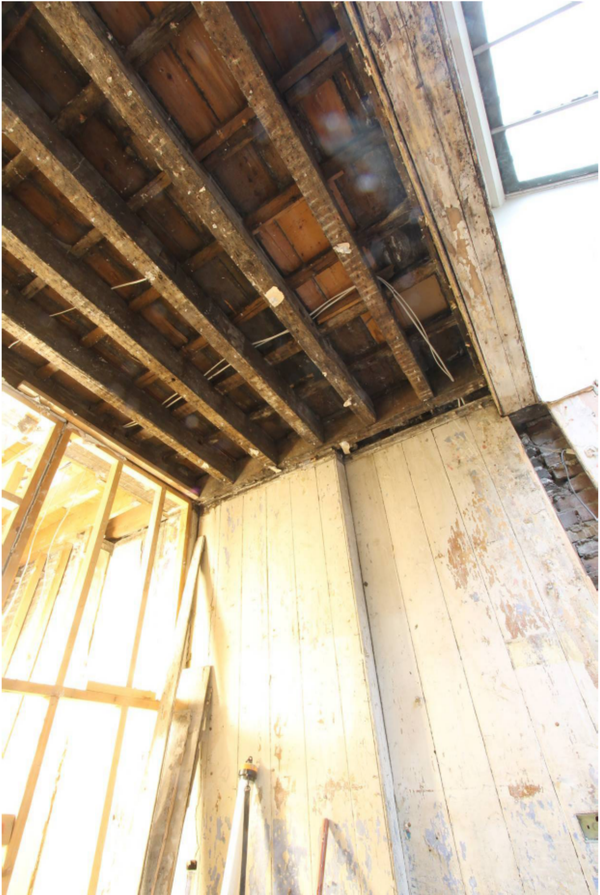
Plate 20 Mezzanine floor FF3 seen from room GF3 below, looking north
