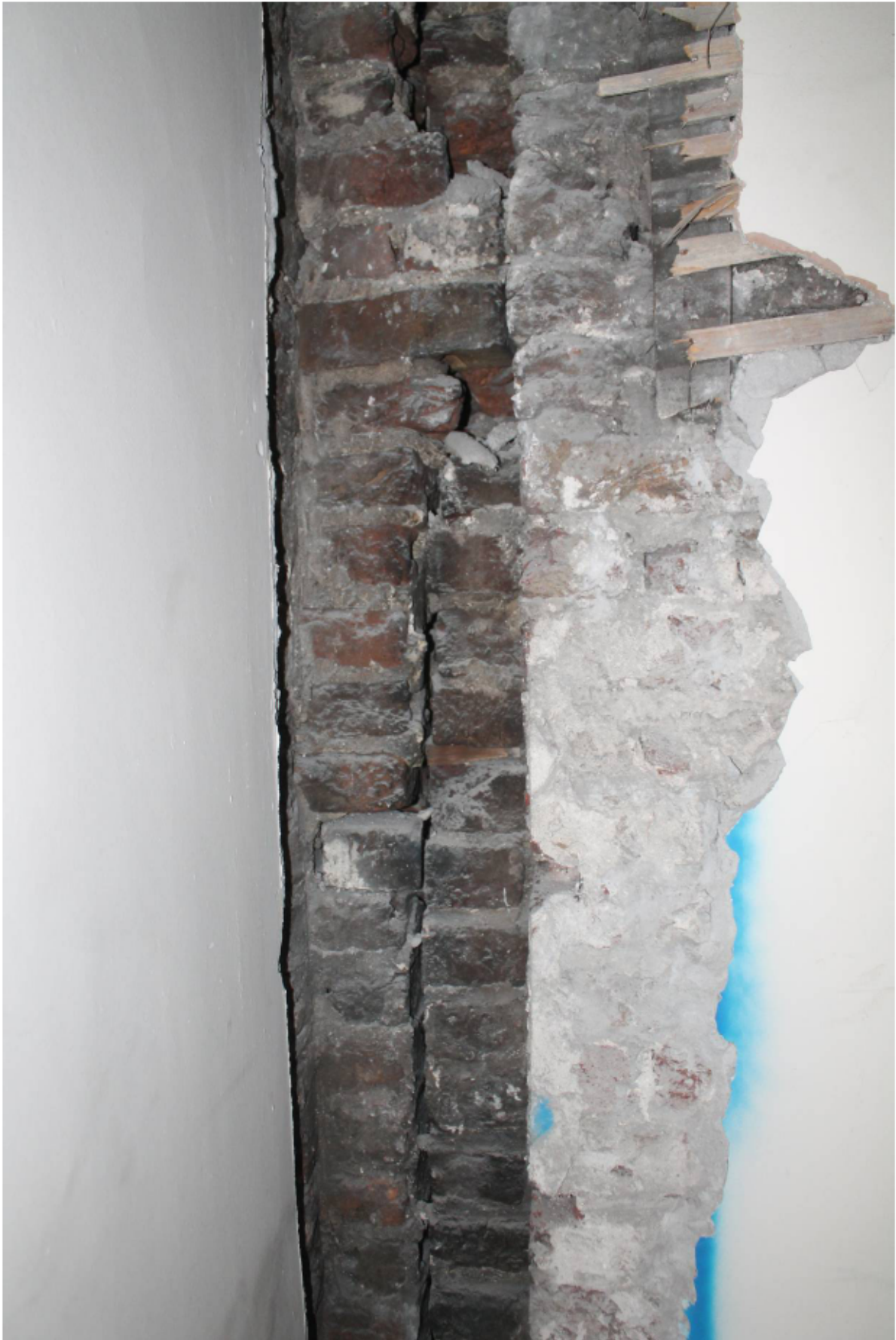
Plate 22 Straight joint in the north-west corner of room SF1, looking north
