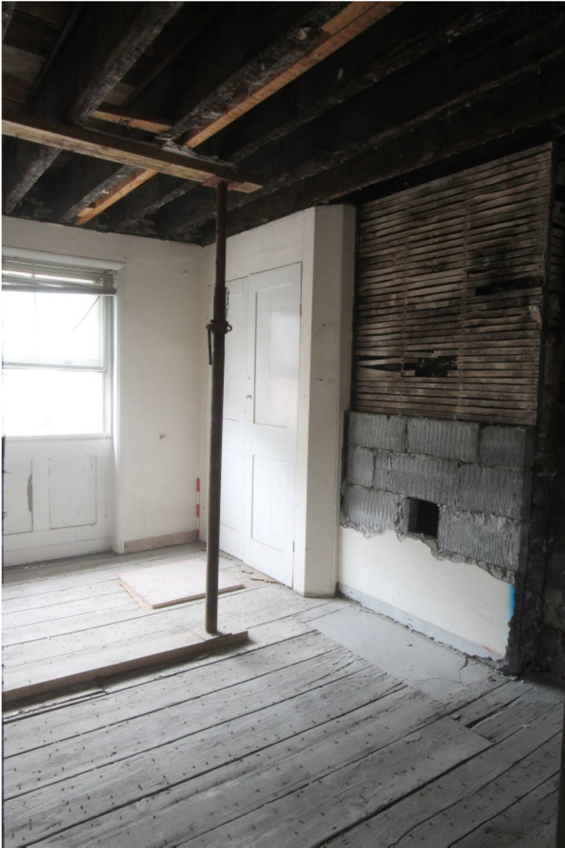
Plate 27 Room TF1 showing built in cupboard, looking south-west
