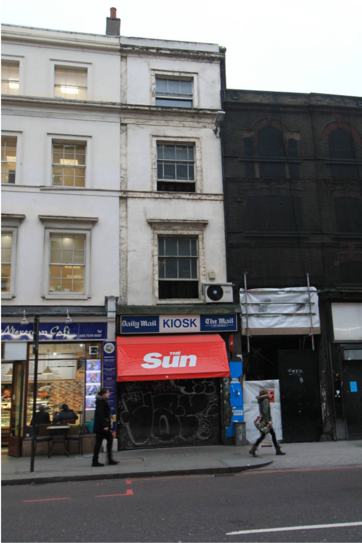
Plate 3 No. 127Borough High Street, looking east
