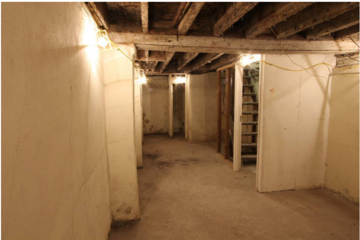
Plate 34 Basement, looking east
