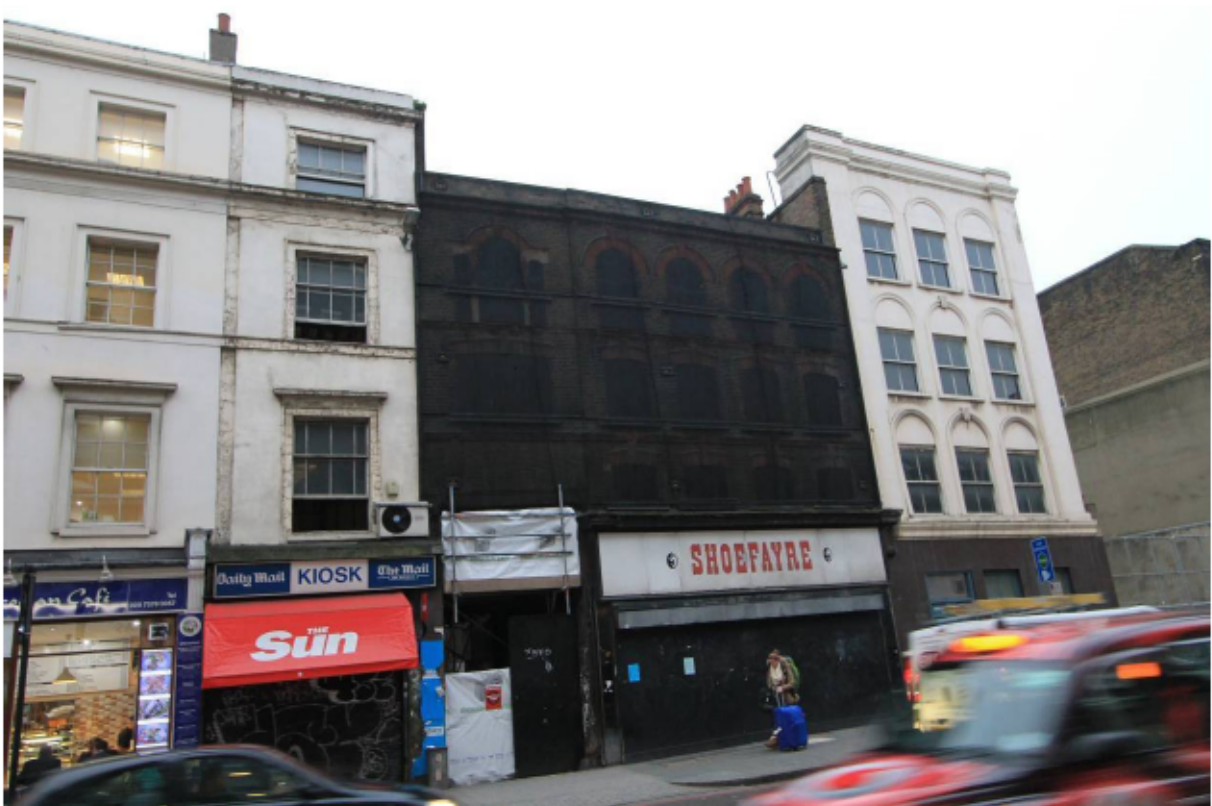
Plate 2 No. 127 (left) and nos 129 to 135, looking south-east
