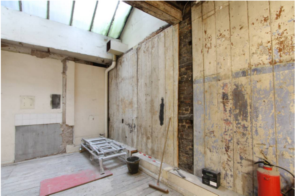
Plate 11 Lean-to extension GF3 showing timber boarding, looking south-east
