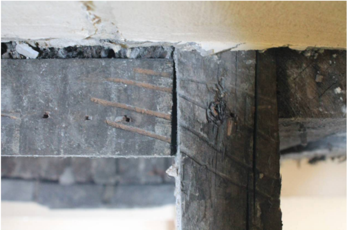
Plate 23 Later scribed carpenters re-assembly marks on primary braced wall frame in the west wall of room SF2, looking west
