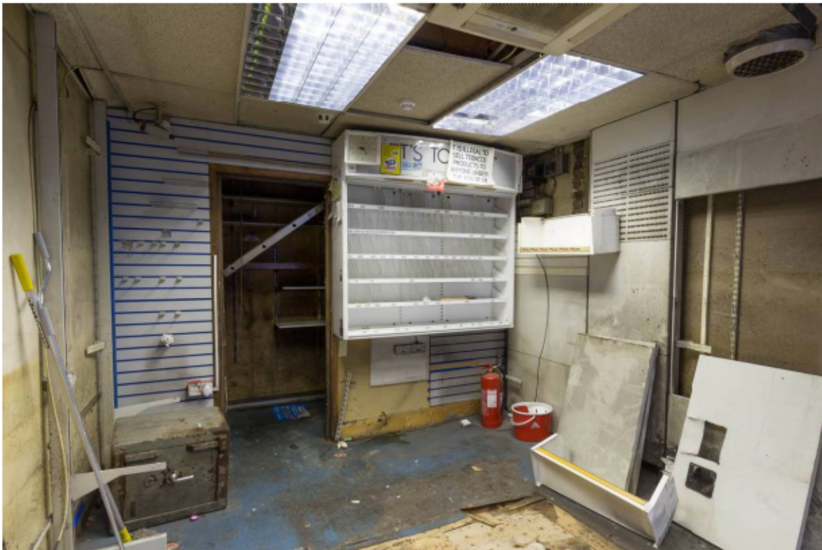
Plate 6 Tobacconist kiosk (GF1) prior to stripping out, looking east
