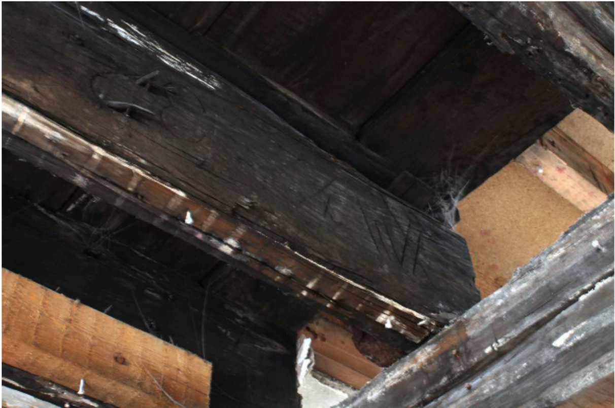
Plate 30 Baltic marks on ceiling joists in room TF1, looking north
