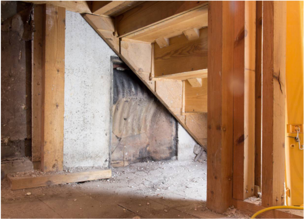
Plate 9 Former fireplace blocked by modern stair in GF2, looking north-east
