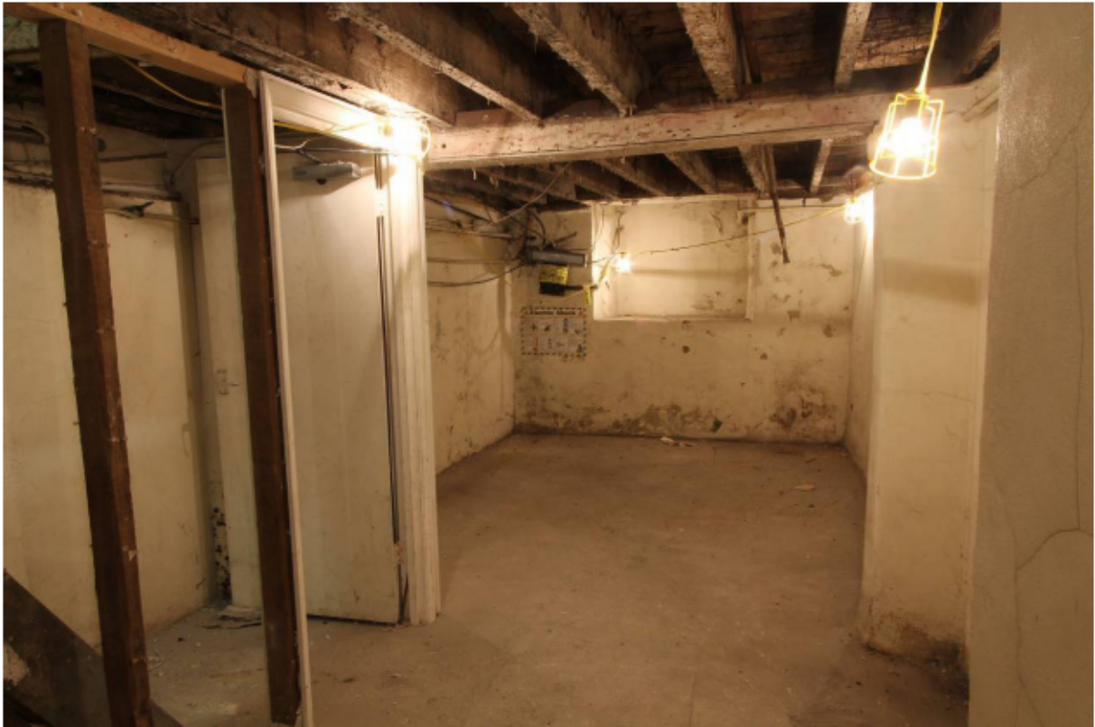
Plate 33 Basement, looking west
