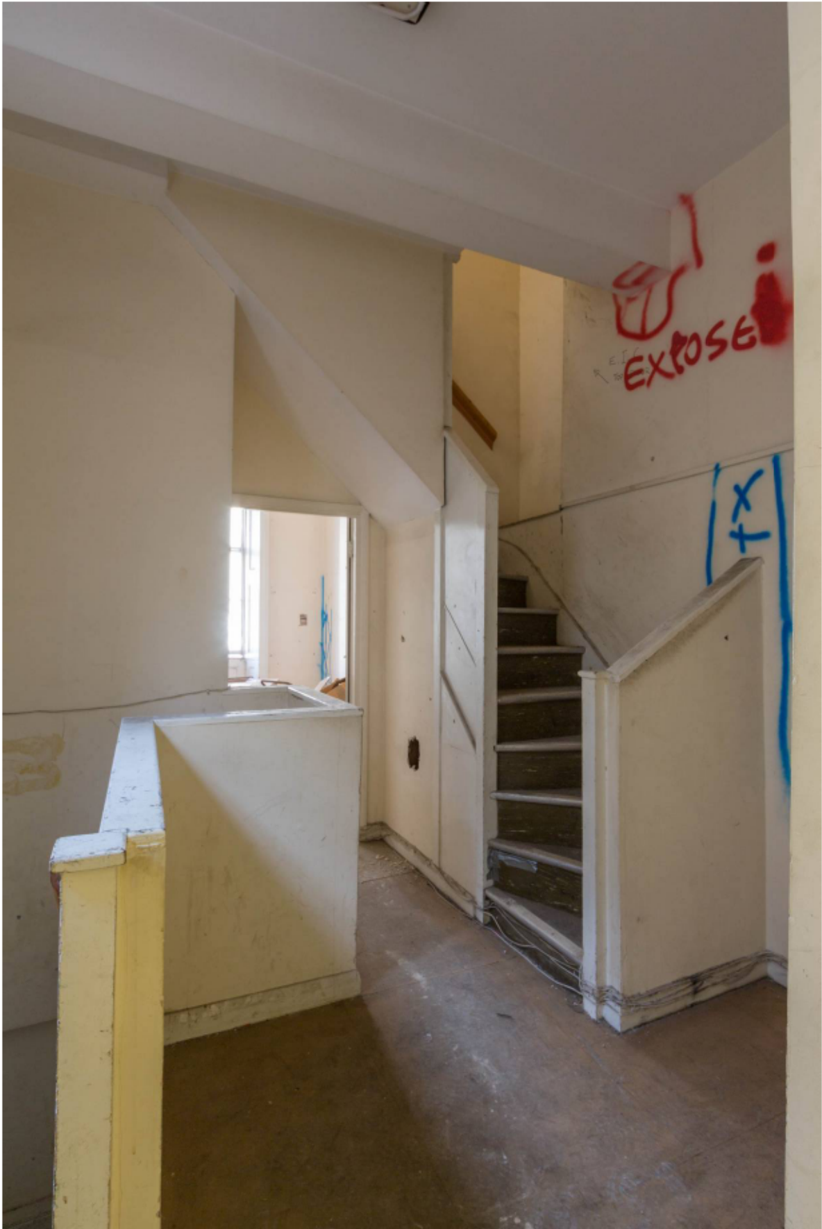
Plate 19 Stairwell FF2 before soft strip, looking north-west
