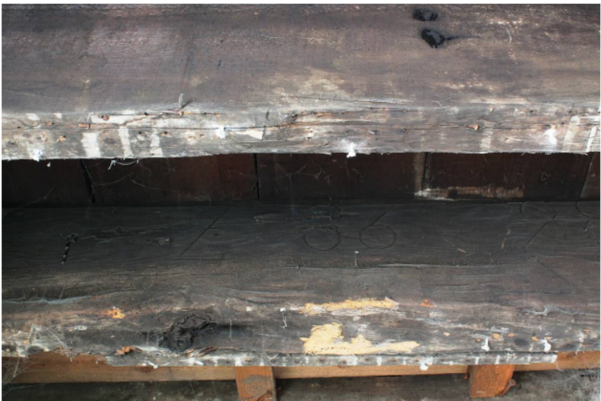
Plate 31 Circular Baltic marks on ceiling joist in room TF3, looking south
