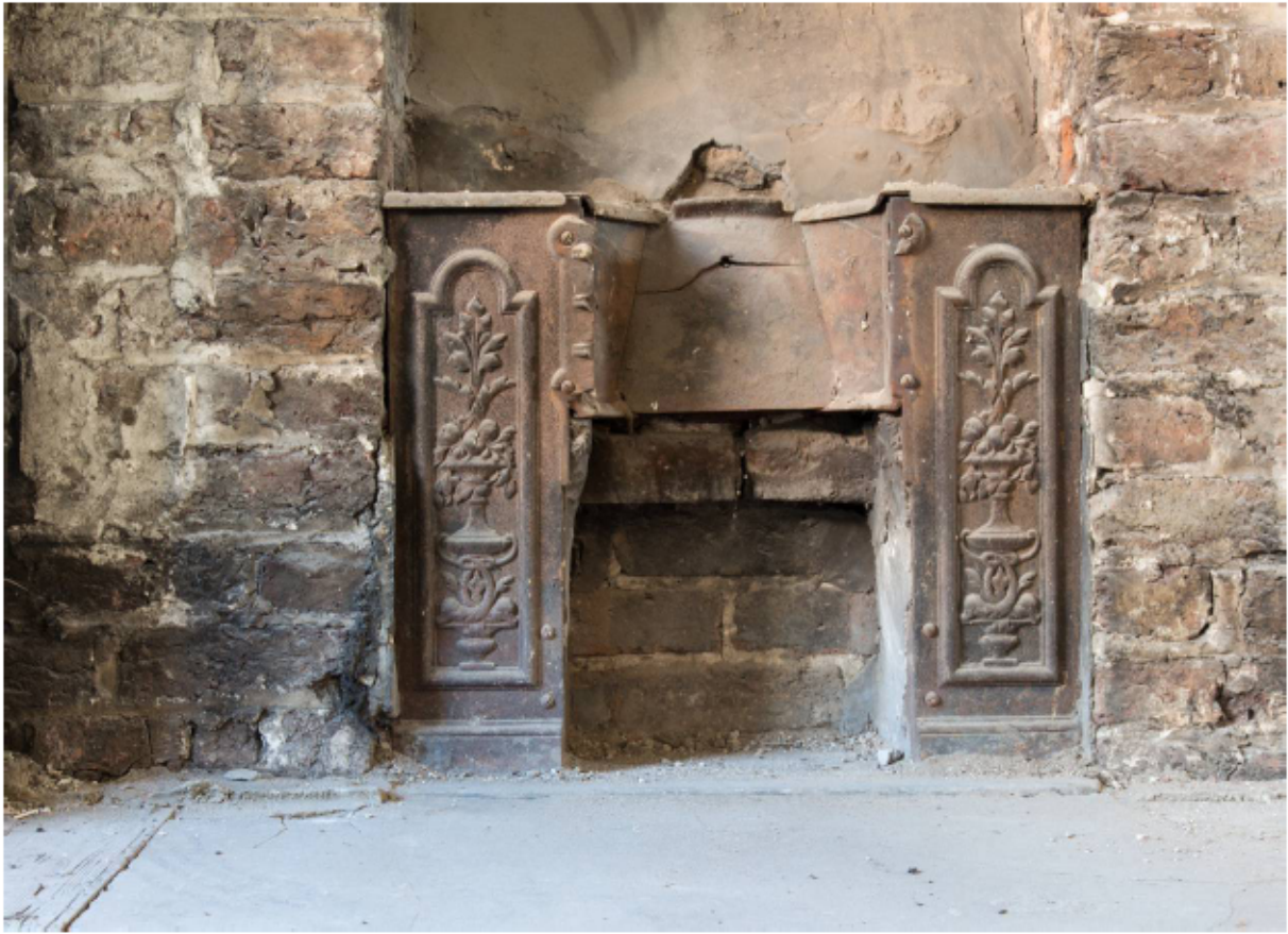
Plate 28 Exposed cast-iron hob grate in room TF1, looking north
