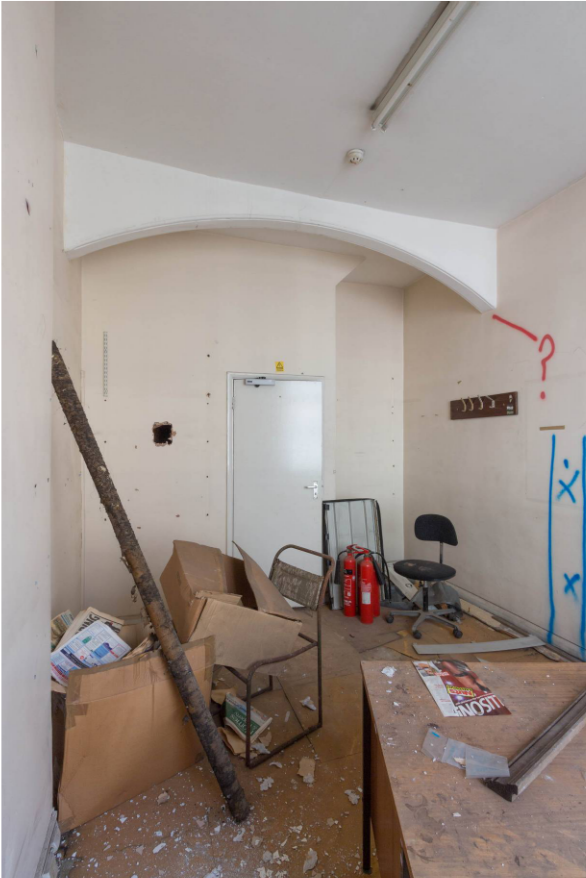
Plate 13 Former sitting room FF1 before soft stripping, looking east
