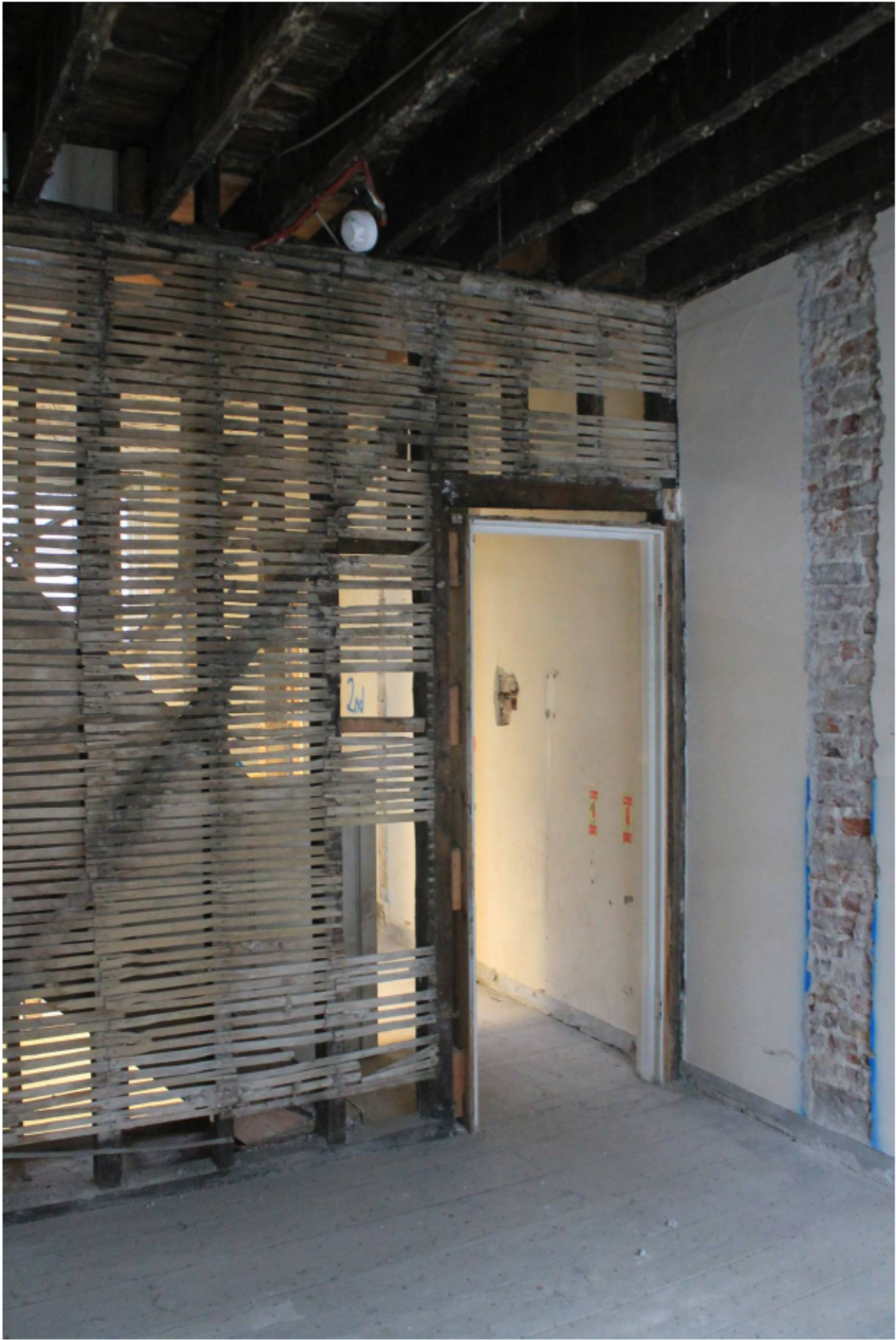
Plate 21 Room SF1 after soft stripping, looking south-east
