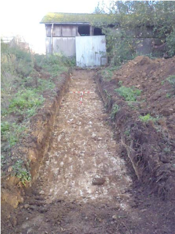
Plate 5: Trench 4 (looking East 2 x1m and 0.3m scales)
